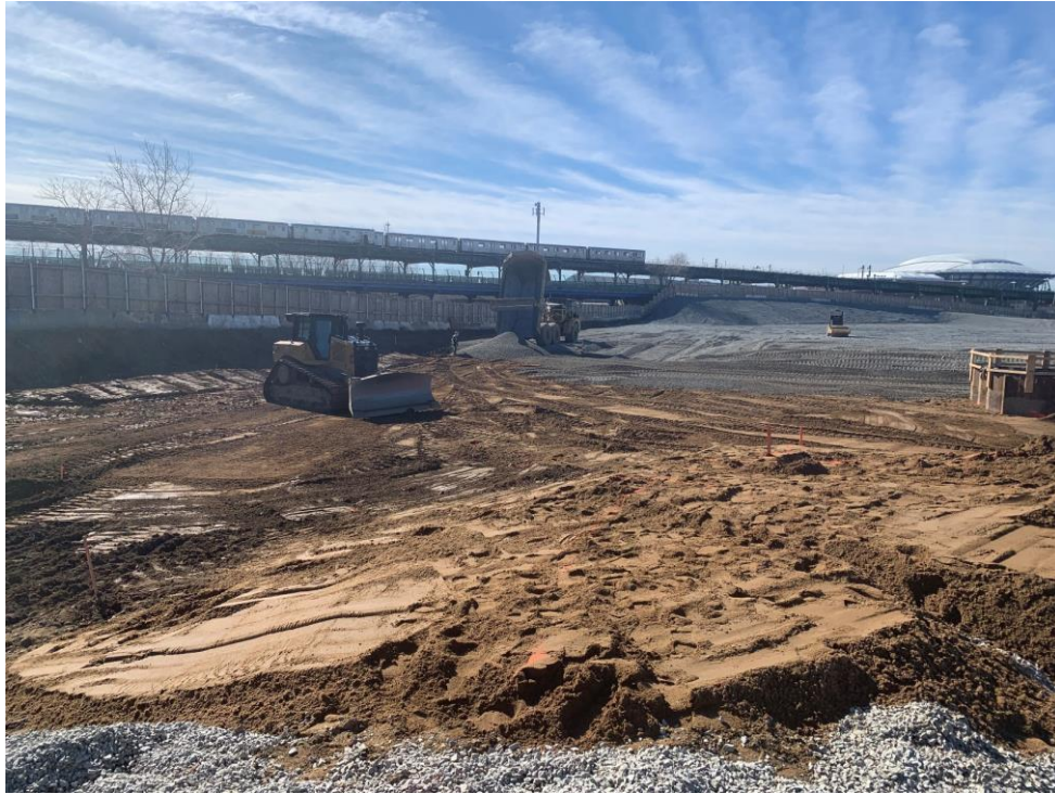
Photo 1: Backfilling and grading composite cap in grids G8 and G9 (facing south).
