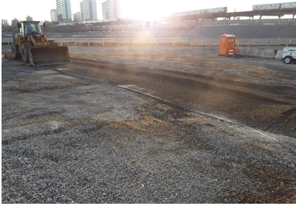
Photo 1: Triumph temporarily backfilling the dewatering trench with imported RCA (facing east)
