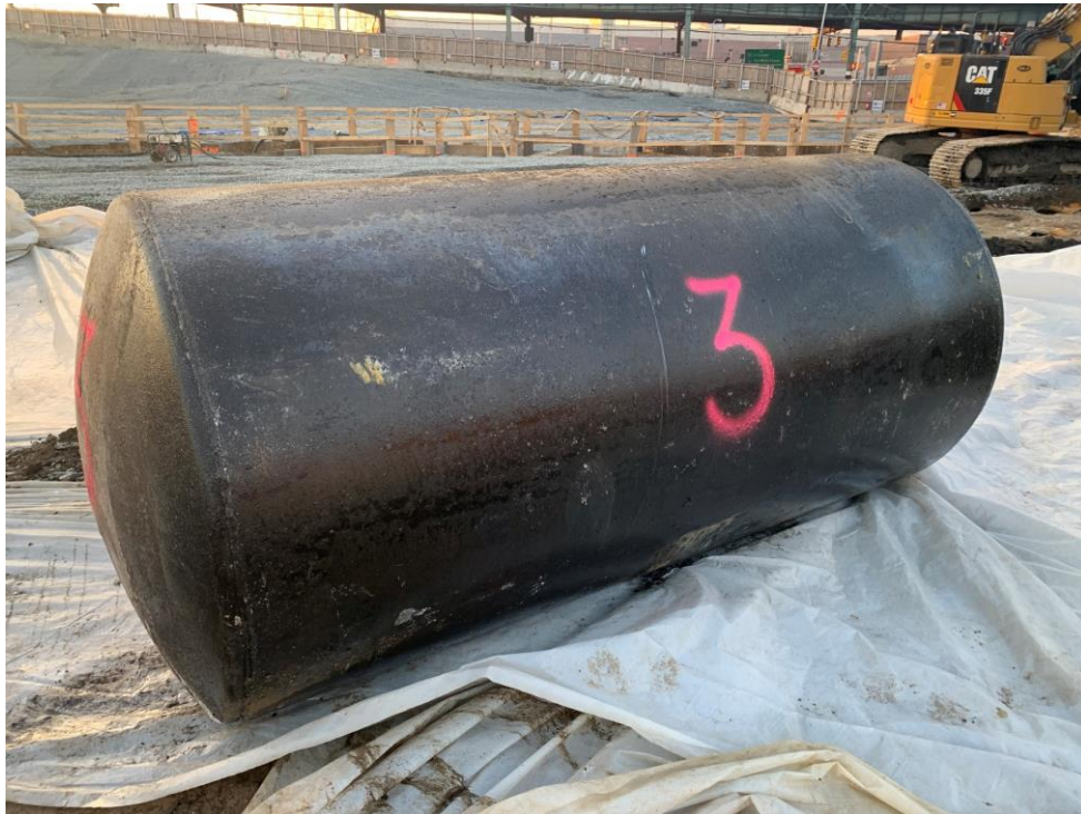
Photo 3: UST removed for inspection and cleaning (facing southeast).
