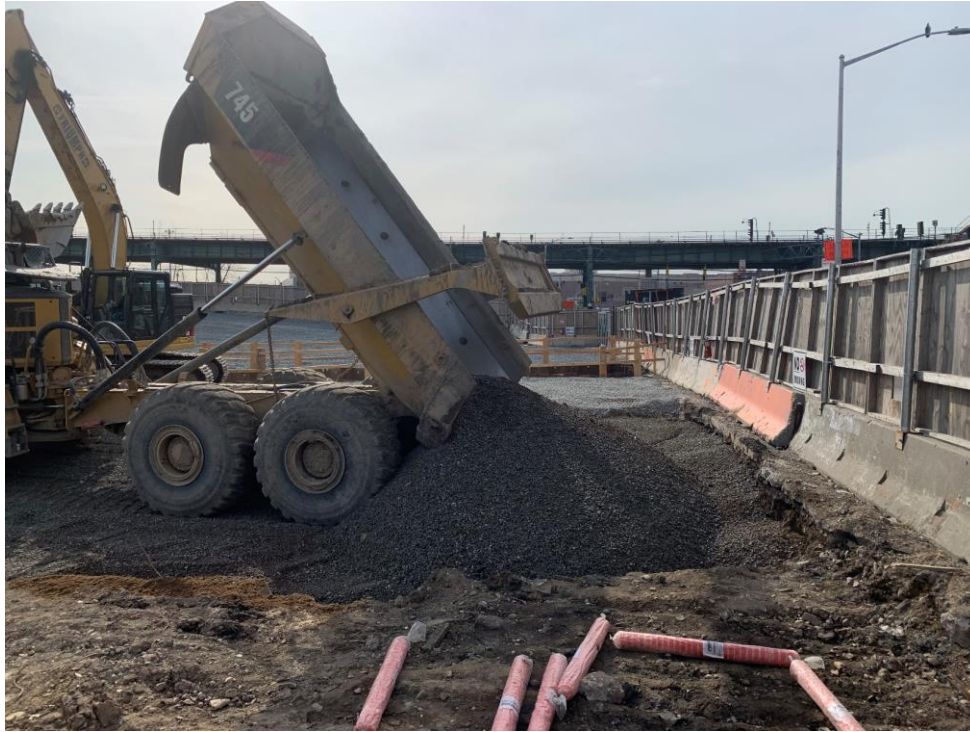
Photo 1: Backfilling UST removal excavation (facing east).
