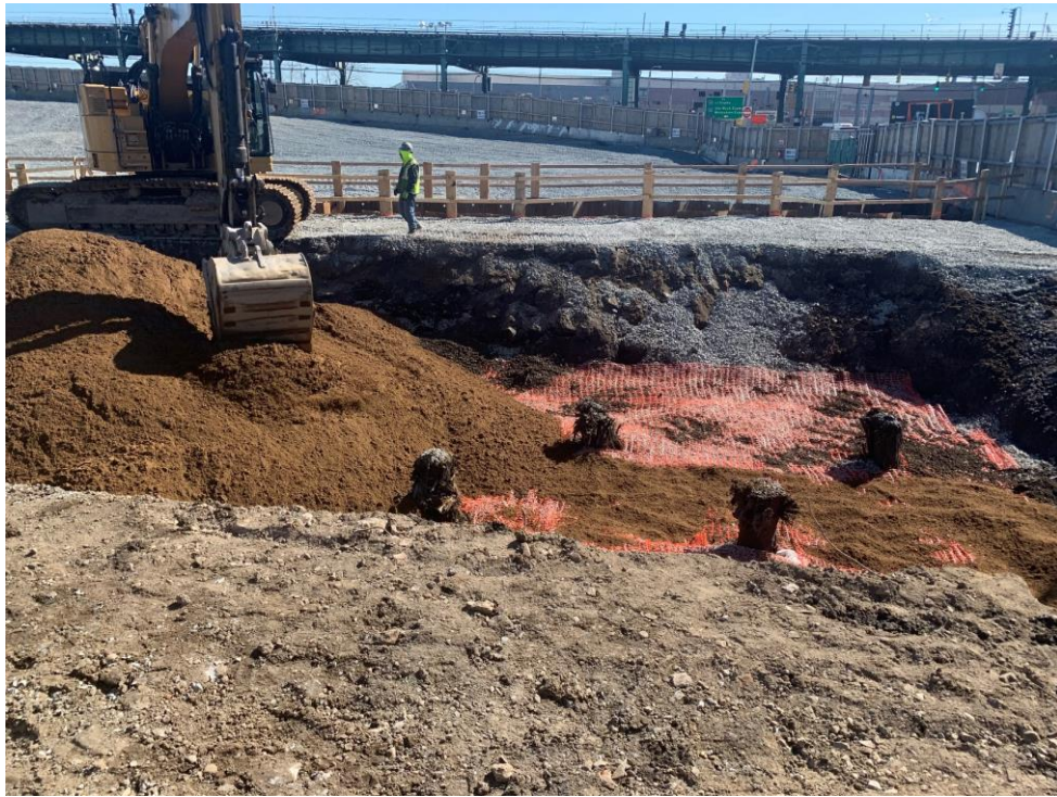
Photo 3: UST removal excavation being backfilled (facing south)
