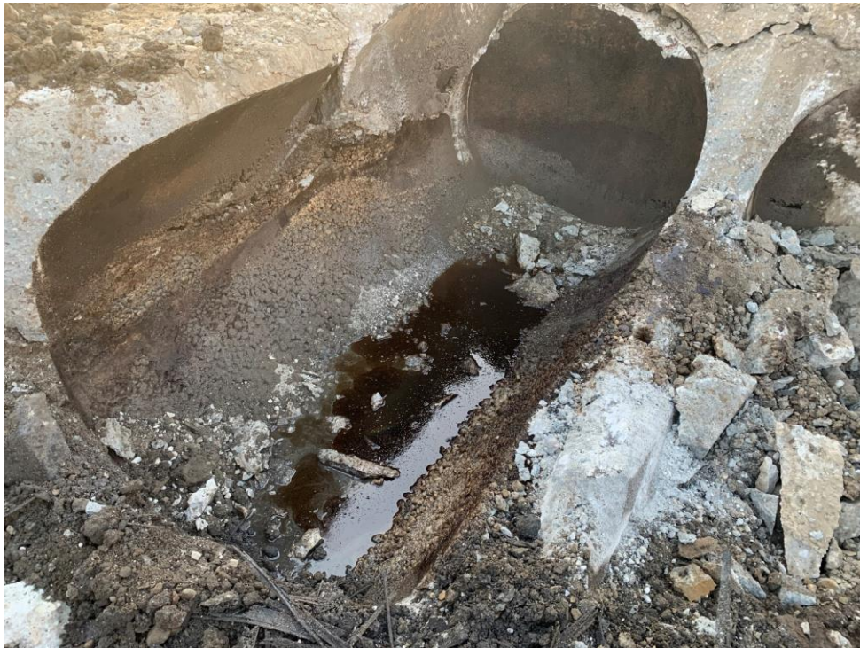
Photo 2: Petroleum-like product in bottom of concrete cradle (facing down)
