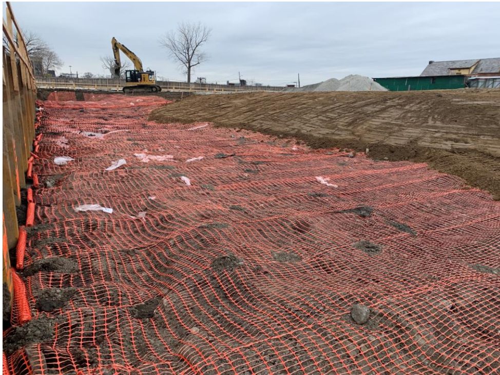
Photo 2: Demarcation and cap progress north of service street SOE in E9 (facing west)
