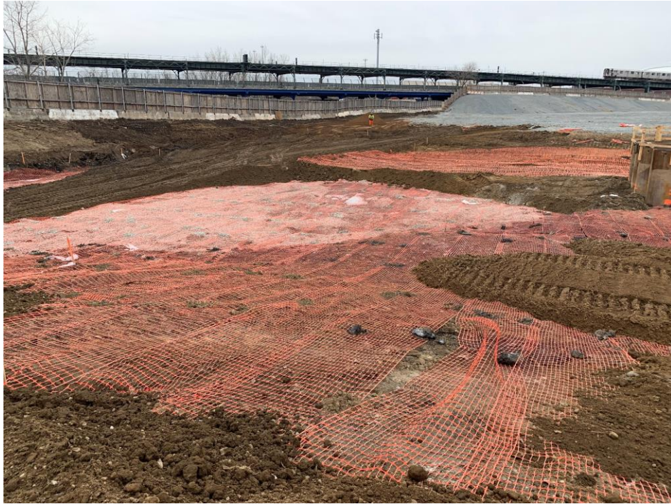
Photo 1: Demarcation placed within grids G8 and G9 and cap construction progress (facing southeast).
