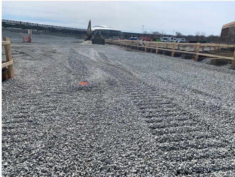
Photo 2: Grading 4-inch layer of quarry gravel (facing south)
