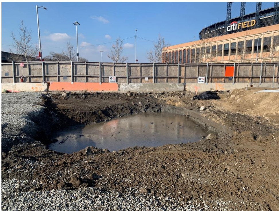
Photo 4: Groundwater with petroleum-like odor and sheen in UST removal excavation (facing west)
