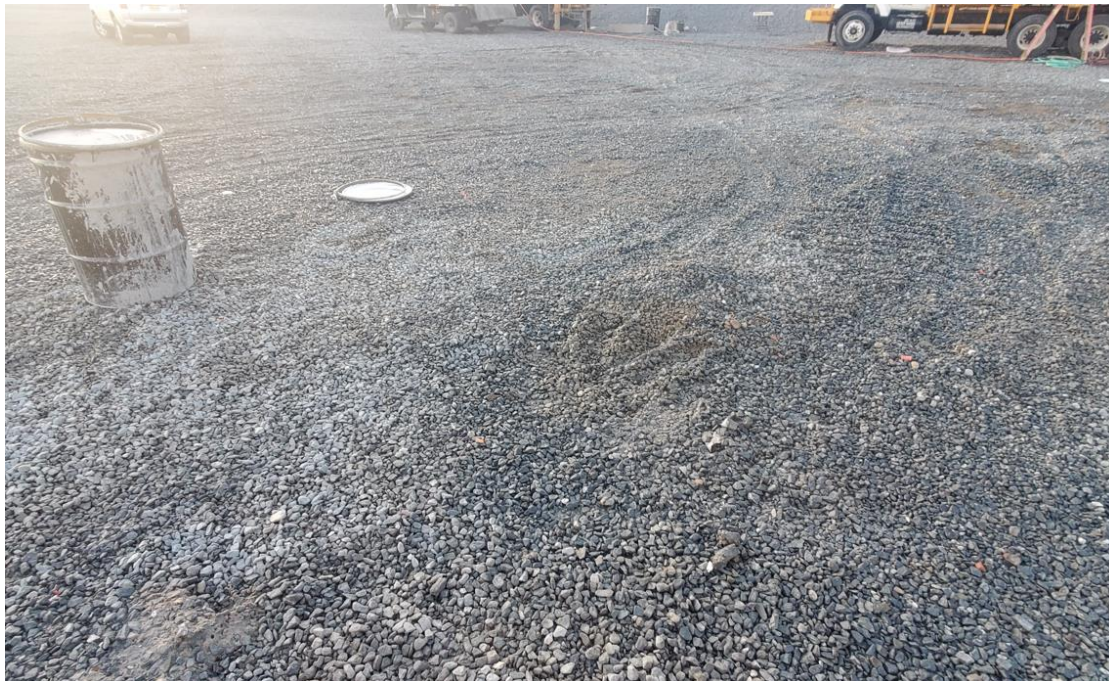
Photo 1: LB-02 backfilled with site cap
