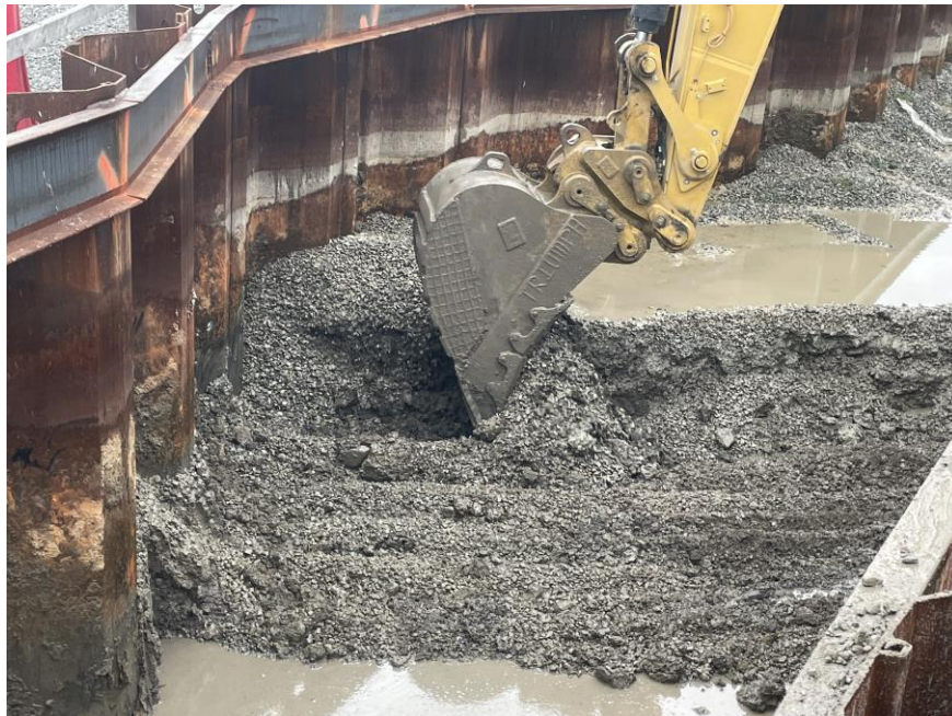
Photo 2: Triumph excavating 3/4-inch stone in the northern part of the 72" truck water main (facing northwest)
