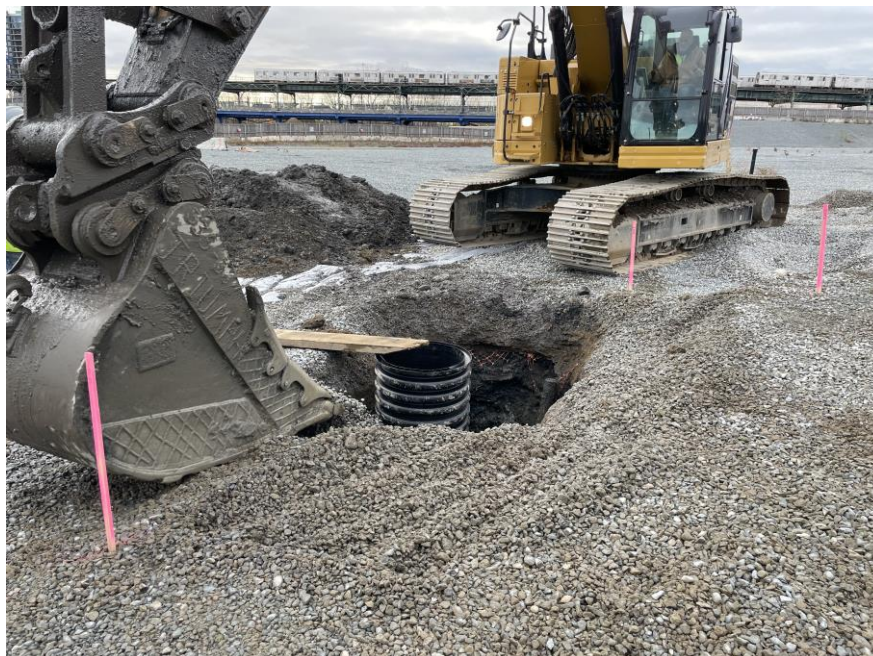
Photo 2: Triumph backfilling excavated area with 3/4-inch stone and imported clean fill (facing southeast)
