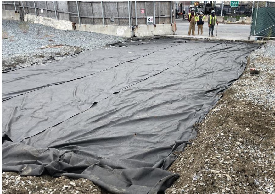
Photo 2: View of placing geotextile fabric for construction entrance in the southwest part of the site (facing southwest)
