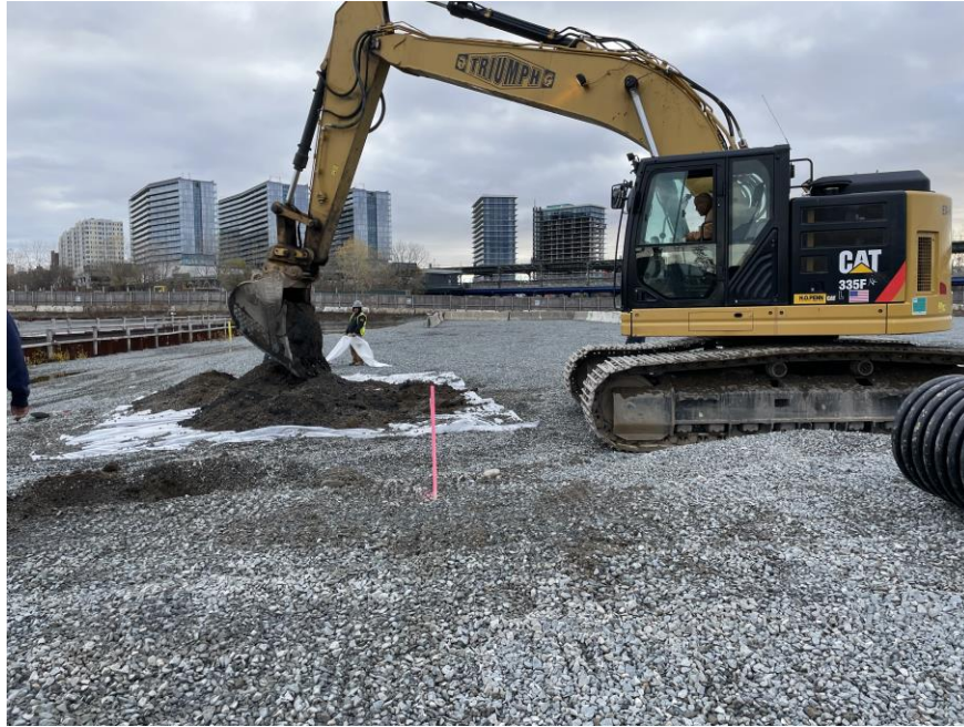
Photo 1: Triumph excavating and segregating clean fill and contaminated fill adjacent to excavation in the southern part of site (facing east)
