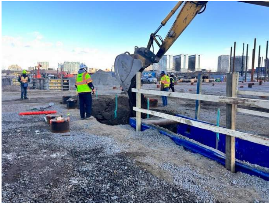
Photo 10: Ferreira backfilling around utilities in the northwestern portion of the Site, facing north. Taken on 1/8/2025.
