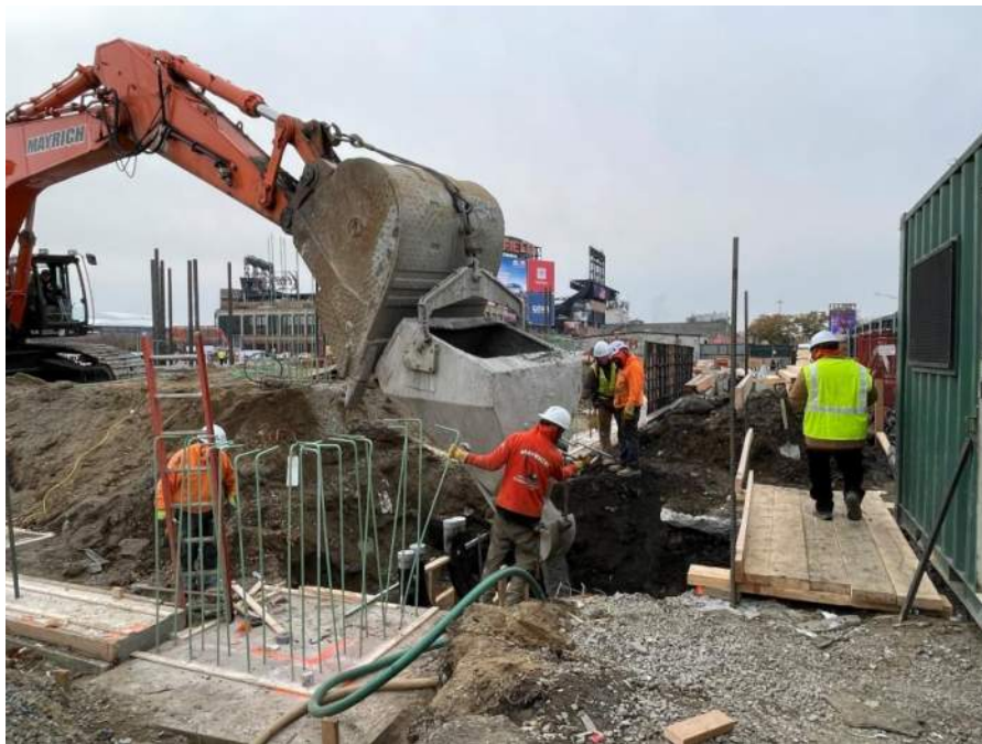
Photo 8: Mayrich pouring concrete in the northeast part of the Site, facing west. Taken on 12/4/2024.
