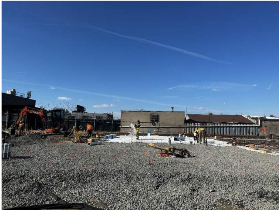
Photo 15: Maccarone installing vapor barrier in the northwest portion of the Site, facing north. Taken on 3/3/2025.
