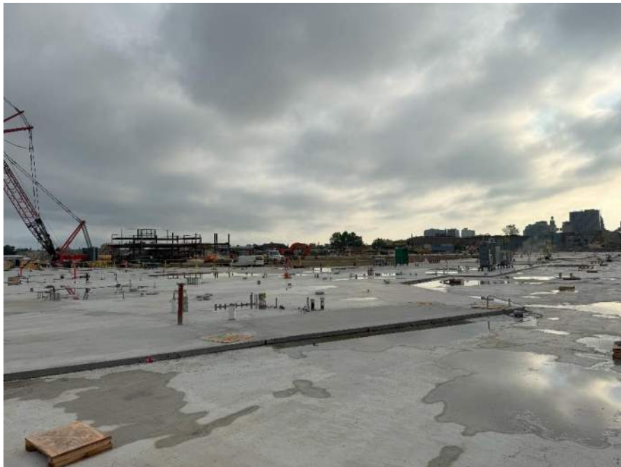
Photo 24: View of completed concrete slab in the southern part of the site, facing northeast. Taken on 7/9/2025.
