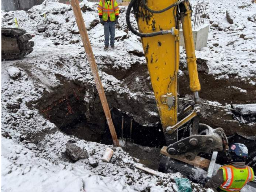
Photo 9: Ferreira excavating for utility installation in the western portion of the Site, facing northwest. Taken on 12/24/2024.
