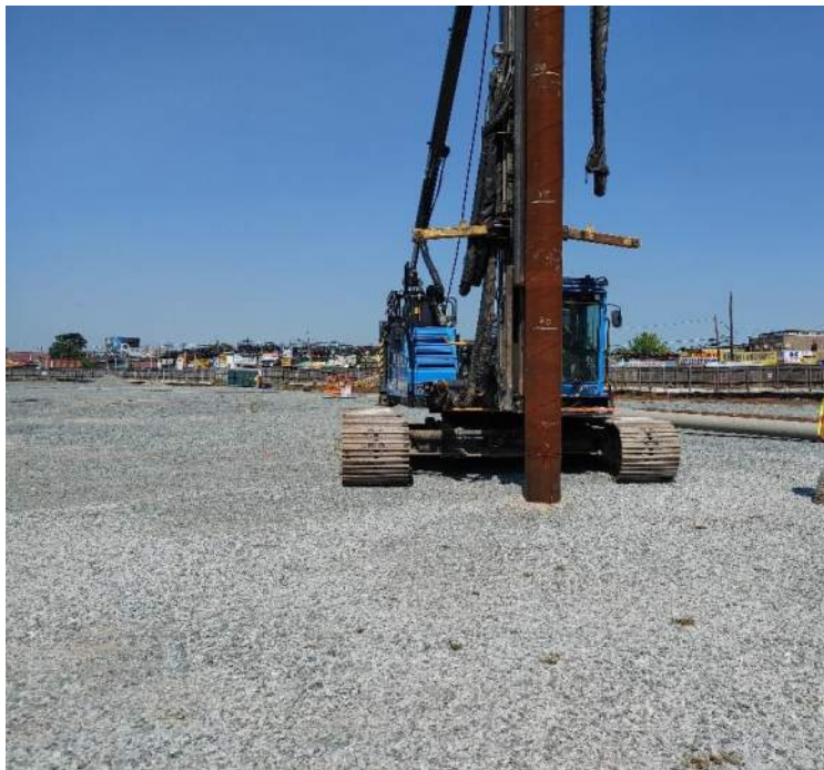
Photo 2: NYCC pile driving a closed-end tapertube pile in southern portion of the Site, facing northeast. Taken on 9/12/2024.
