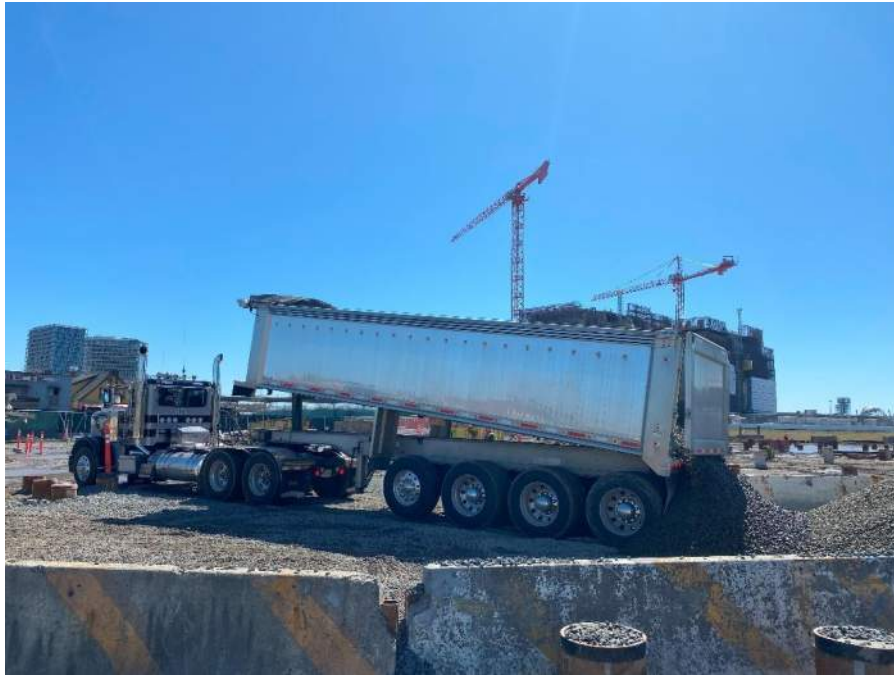
Photo 17: Mayrich importing ASTM #5 stone in the northeast portion of the Site, facing southeast. Taken on 3/21/2025.
