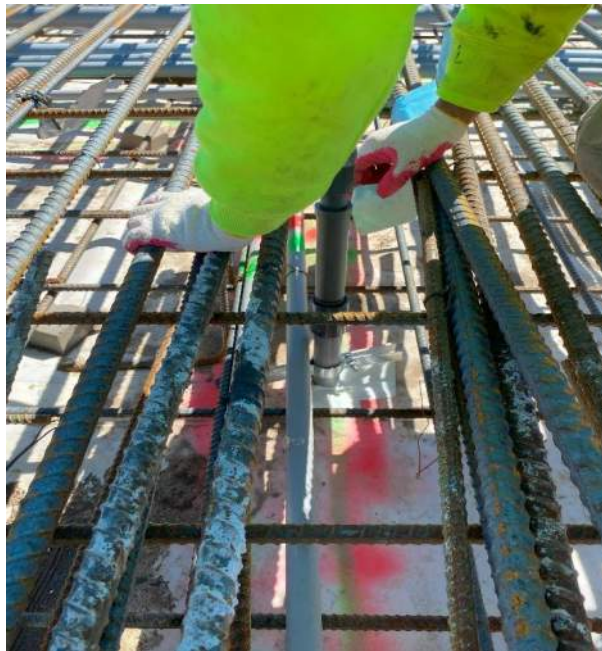
Photo 18: Starbright patching waterproofing and vapor barrier around SMD components in the northwest portion of the Site, facing southeast. Taken on 3/21/2025.
