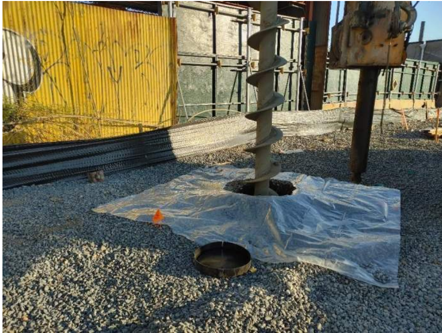
Photo 5: Typical pile pre-augering. Facing northwest, taken on 10/23/2024.
