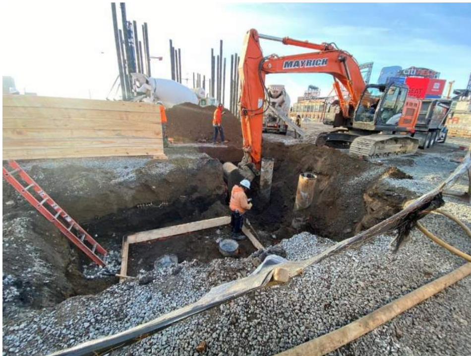
Photo 6: Typical excavation at a pile cap in the northeast part of the Site, facing southwest. Taken on 11/27/2025.
