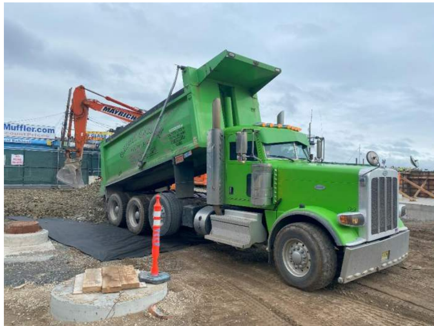
Photo 20: Mayrich importing 2 to 4-inch Granite Stone in the western portion of the Site, facing west. Taken on 4/11/2025.
