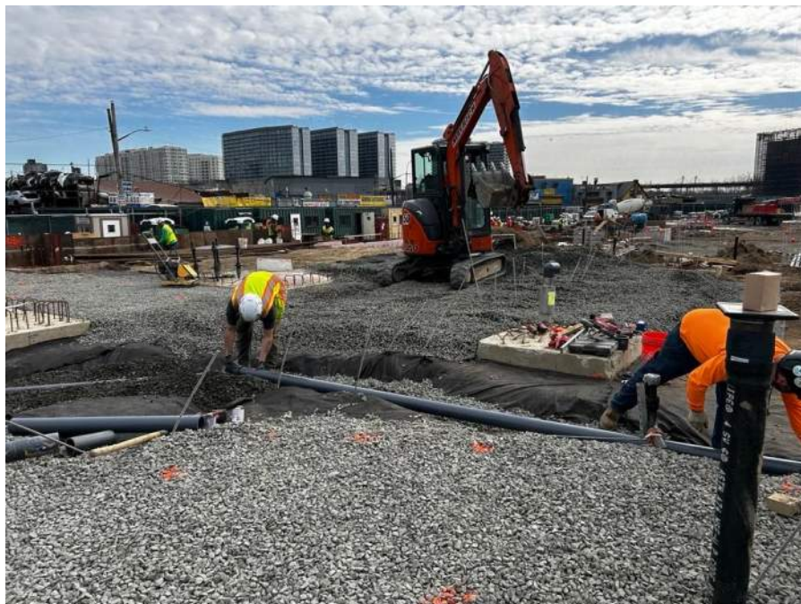
Photo 14: Maccarone installing sub-grade SMD components in the northeast portion of the Site, facing east. Taken on 2/25/2025.
