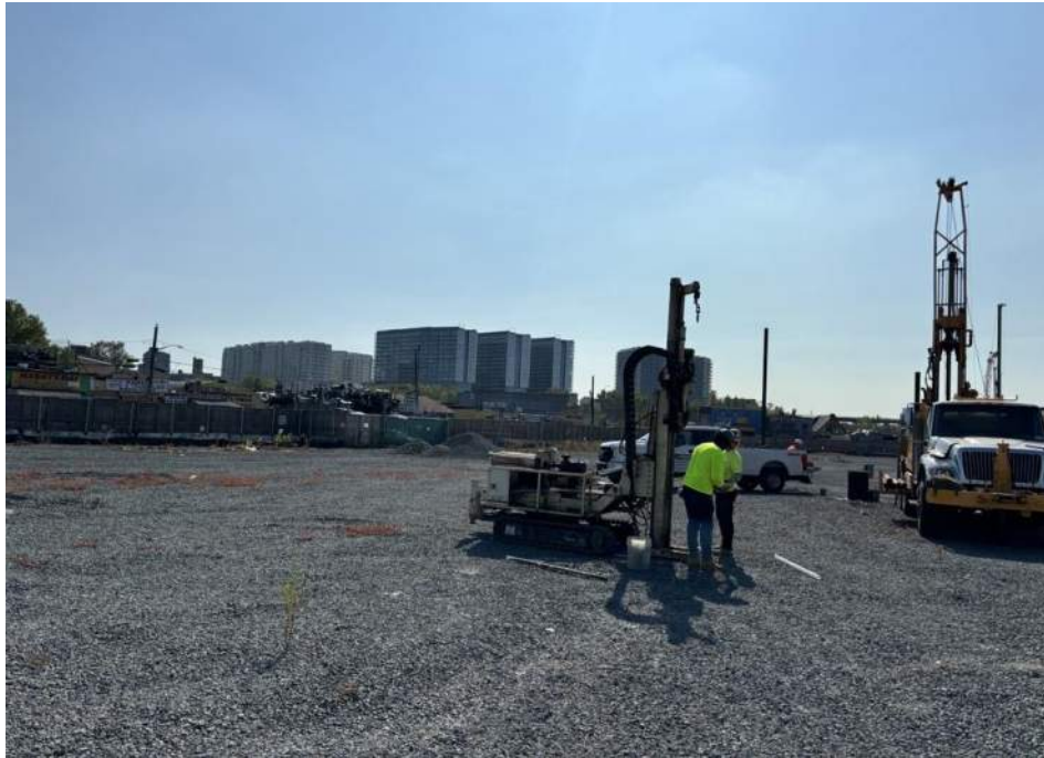
Photo 3: AARCO using Geoprobe 6610DT to advance a waste characterization soil boring, facing south. Taken on 9/13/2024.
