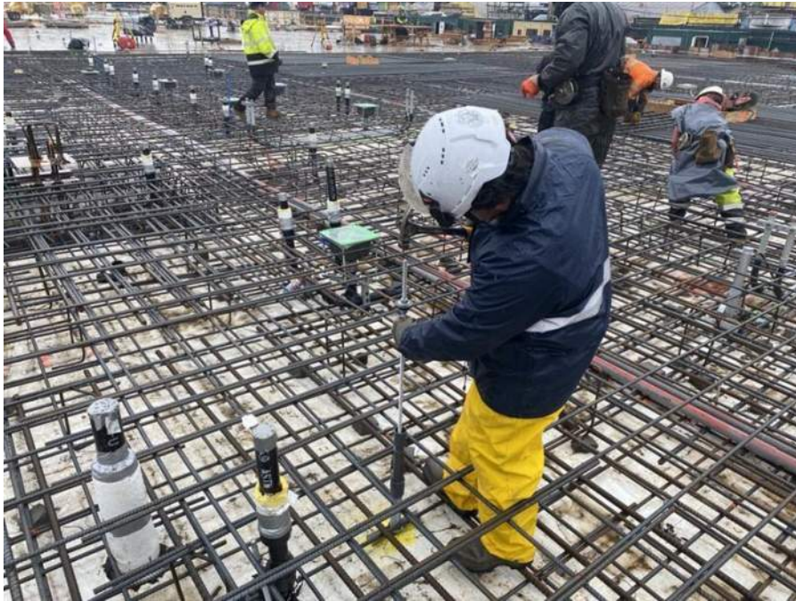
Photo 21: Maccarone installing a vapor monitoring point in the eastern part of the Site, facing north. Taken on 5/9/2025.
