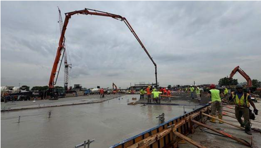
Photo 23: Mayrich pouring concrete for the foundation slab in the eastern part of the site, facing north. Taken on 7/2/2025.
