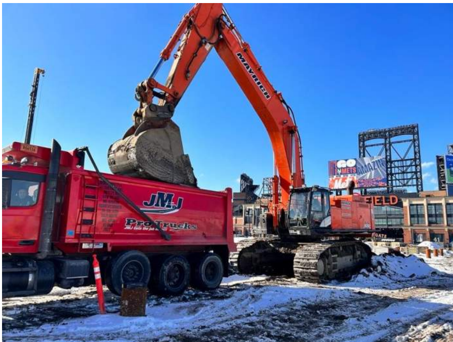
Photo 12: Mayrich exporting soil and fill from the central portion of the Site, facing west. Taken on 2/10/2025.
