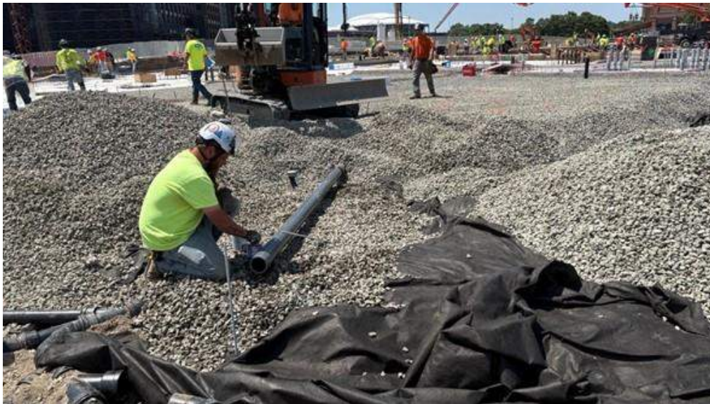
Photo 22: Maccarone installing sub-slab piping and the gas permeable aggregate layer as part of SMD System 10 in the eastern part of the site, facing southeast. Taken on 6/20/2025.
