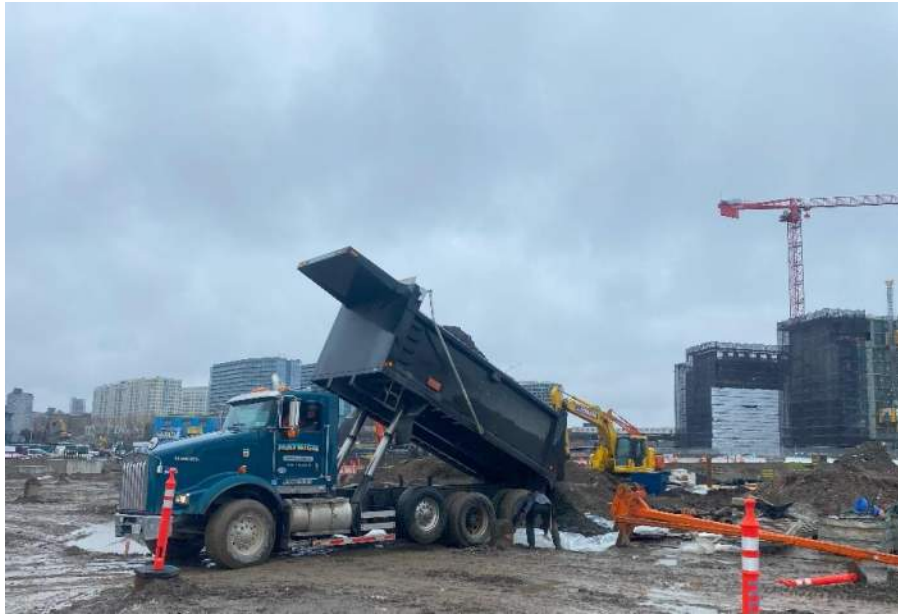
Photo 19: Mayrich stockpiling excavated soil on polyethylene sheeting pending off-site disposal in the central part of the Site, facing southeast. Taken on 4/2/2025.
