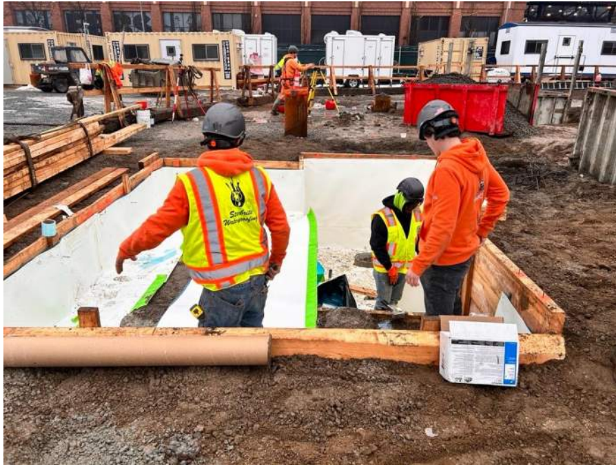
Photo 13: Starbright installing waterproofing in the southwest portion of the Site, facing west. Taken on 2/13/2025.
