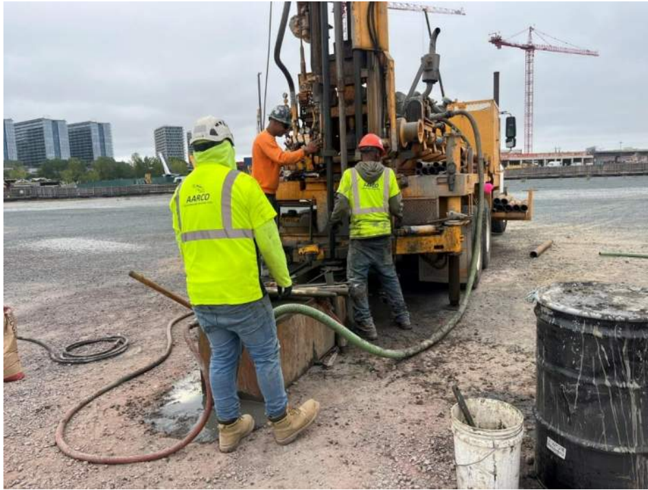
Photo 1: AARCO advancing soil boring as part of a geotechnical investigation in the central part of the Site, facing south. Taken 9/6/2024.
