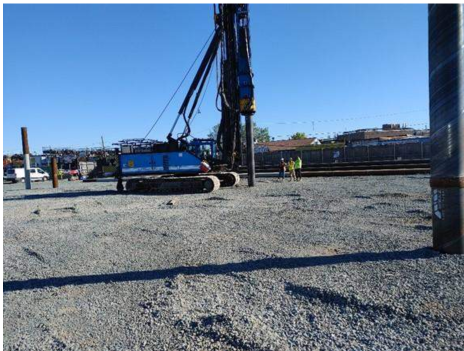
Photo 4: NYCC driving a closed-end tapertube pile, Pile 309-4, facing northeast. Taken on 10/8/2024.
