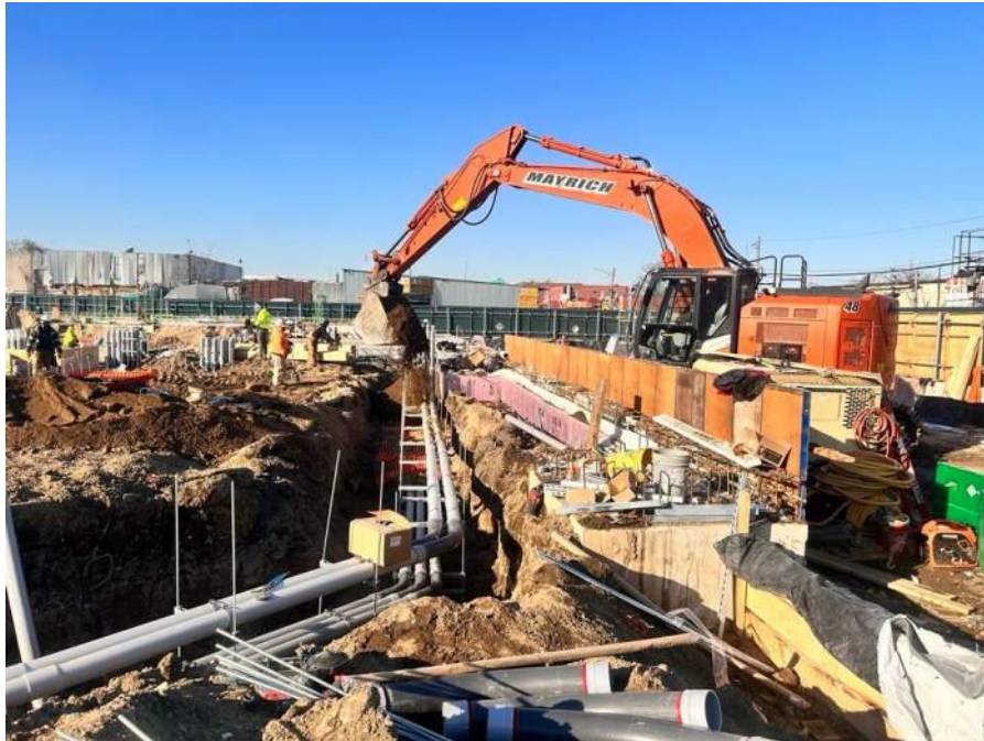
Photo 11: Mayrich backfilling with imported clean fill in the northeast portion of the Site, facing north. Taken on 1/22/2025.
