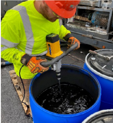
The image shows the homogenization of PetroFix using a high torque/high rpm mixer with appropriate mixing paddle.
