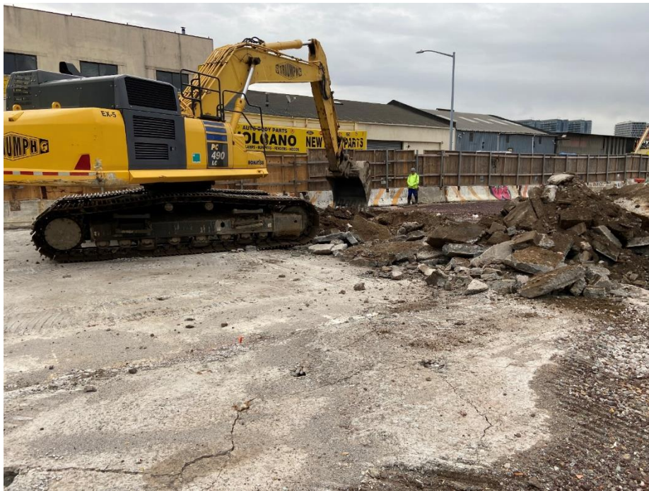
Photograph 10: Triumph excavating and removing the former building slab on the northeastern part of the Site (facing southeast). – 5/2/2023
