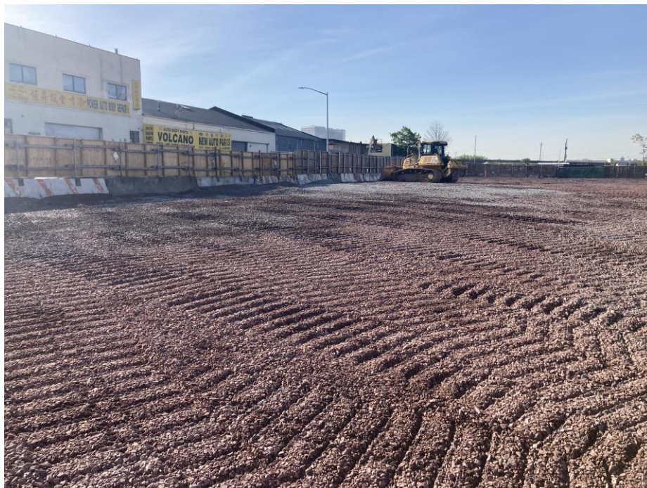
Photograph 12: Triumph grading 0.75-inch stone above in the eastern part of the Site (facing south). – 5/8/2023
