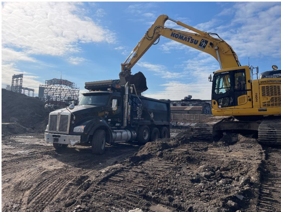
Photograph 4: Triumph loading non-hazardous fill from the Site into a truck for off-site disposal (facing southwest). – 1/30/2023
