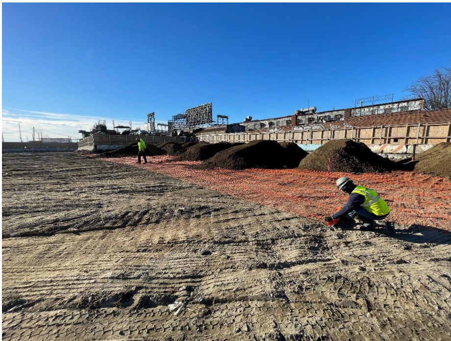
Photograph 6: View of Triumph placing the demarcation layer in the western part of the Site (facing southwest). – 2/10/2023
