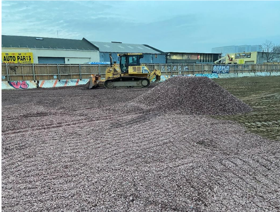
Photograph 9: Triumph backfilling 0.75-inch stone in the eastern part of the Site (facing southeast). – 3/23/2023
