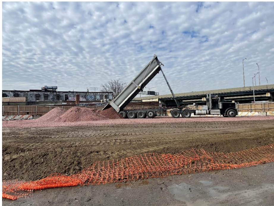
Photograph 8: View of 0.75-inch stone being imported in the northern part of the Site (facing west). – 3/1/2023
