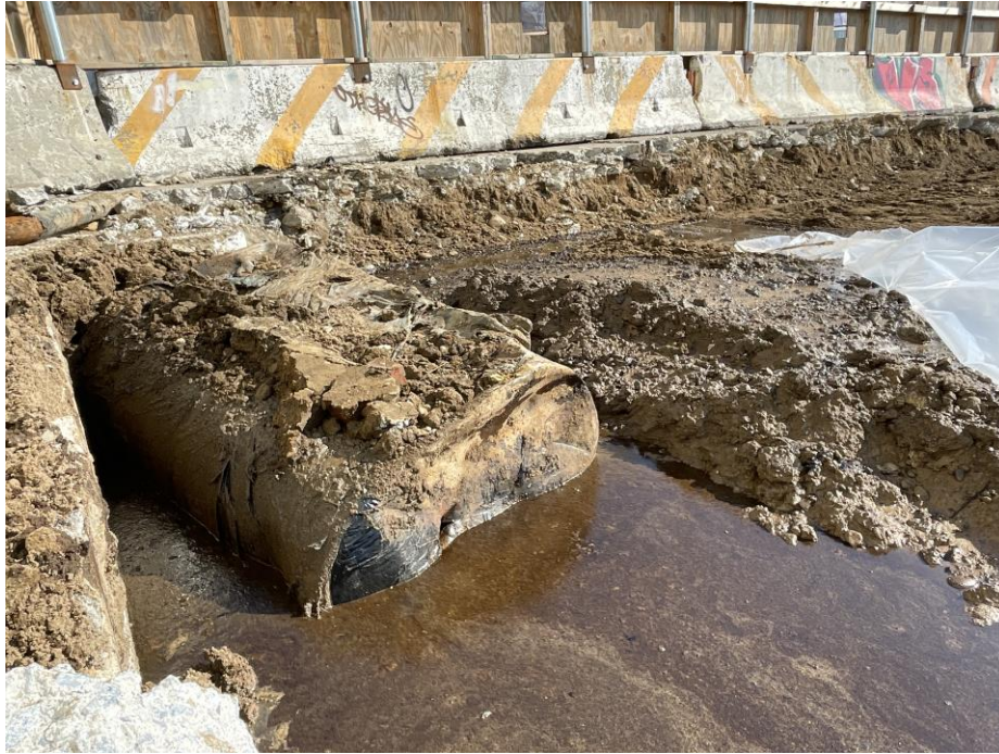
Photograph 5: View of the UST that was uncovered on the eastern part of the Site (facing east). – 2/6/2023
