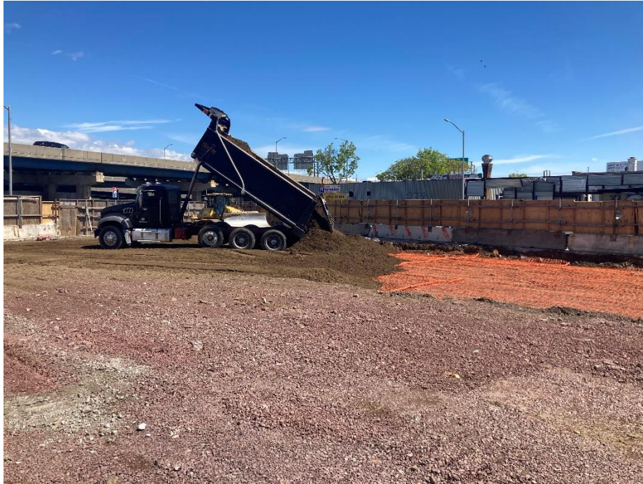
Photograph 11: Triumph backfilling clean fill above a demarcation barrier in the northeastern part of the Site (facing northeast). – 5/5/2023
