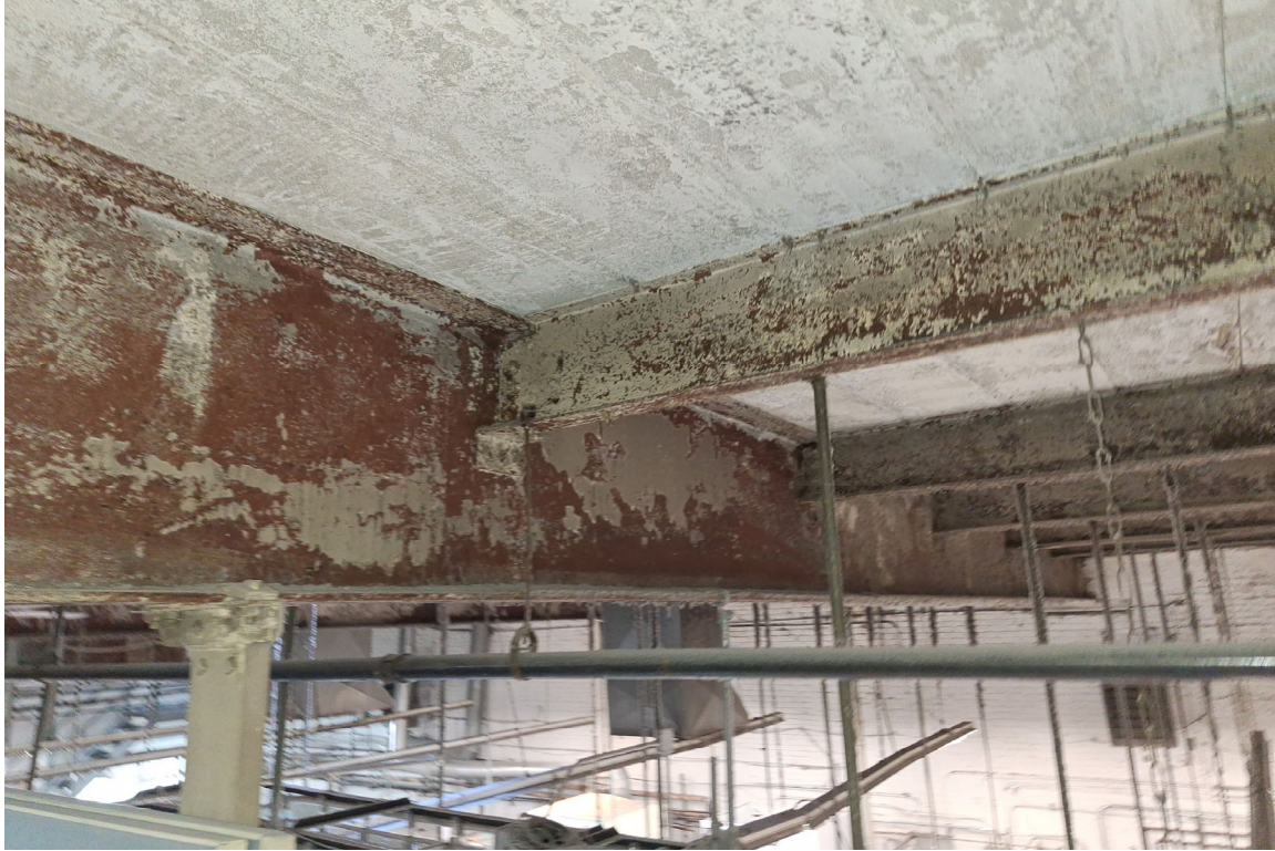
Photo 3. View of the underside of the roof structure with main girder, secondary beam, and precast concrete planks.
