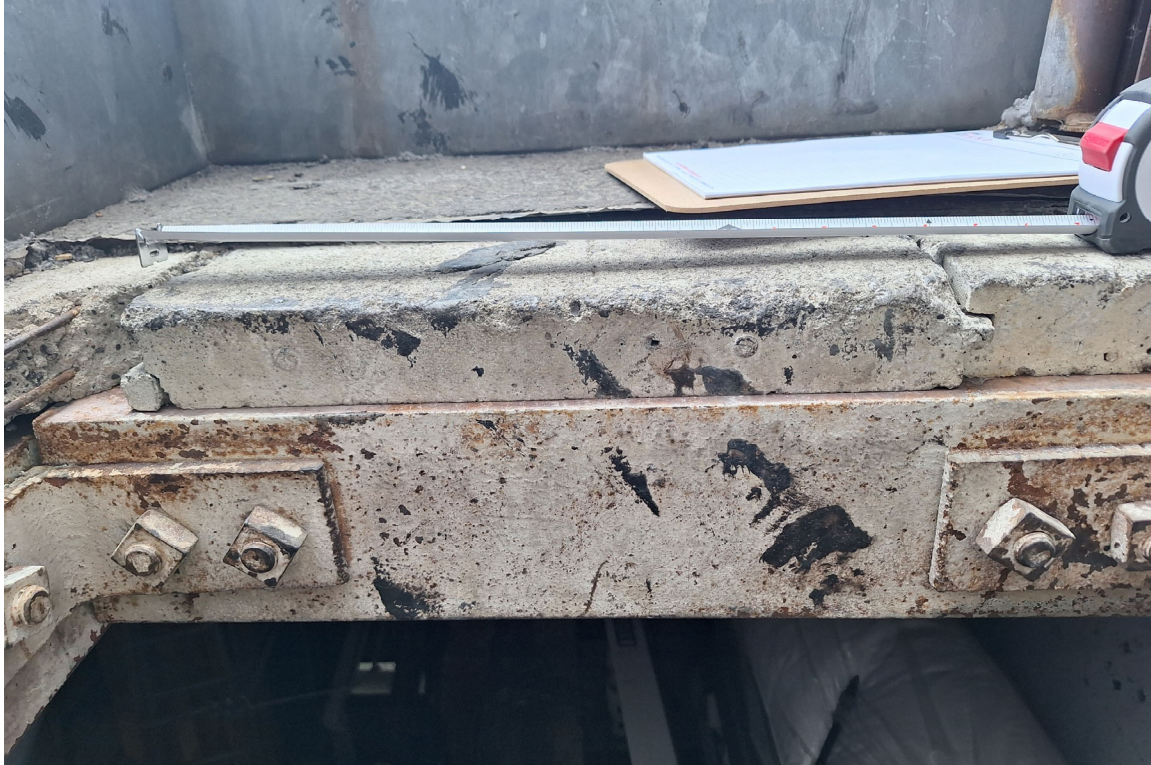
Photo 3. View of the underside of the roof structure with main girder, secondary beam, and precast concrete planks.
