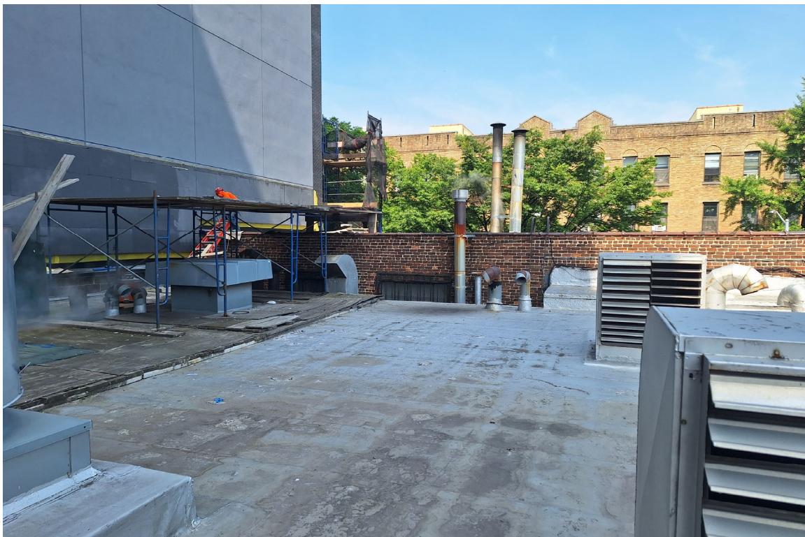
Photo 2. Roof of the southern portion of 35-45 35 th Street; looking west.
