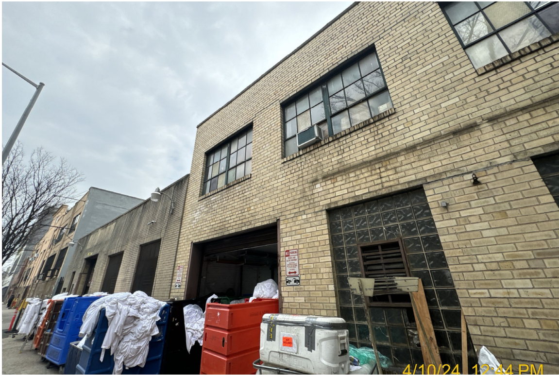
Photo 1. 35 th Street elevation view of 35-45 35 th Street.
