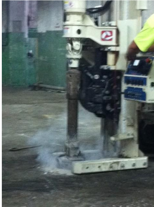
Photograph 1: View of Craig advancing a soil boring at the Site.
