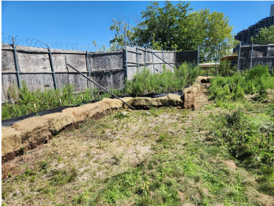
Photo 9: View of repaired sediment/erosion fence and replaced hay bales along northeastern site boundary, facing east (taken on 08/25/23)
