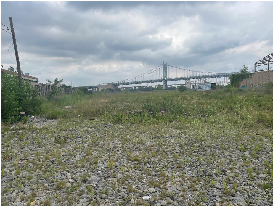
Photo 2: View of site cover system during annual inspection, facing north (taken on 06/27/2023)
