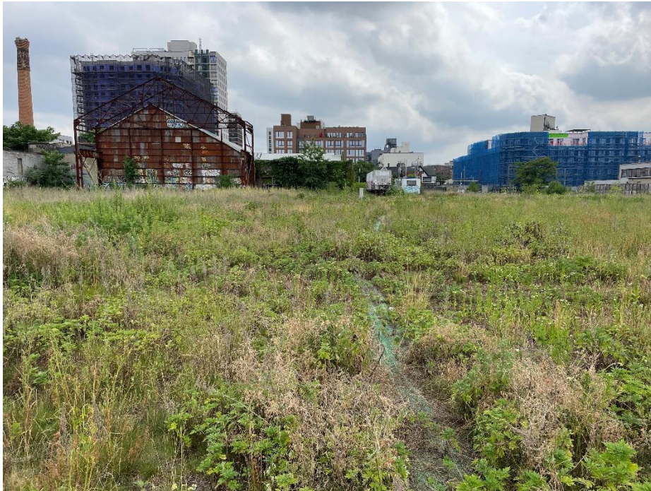
Photo 1: View of site cover system during annual inspection, facing south (taken on 06/27/2023)
