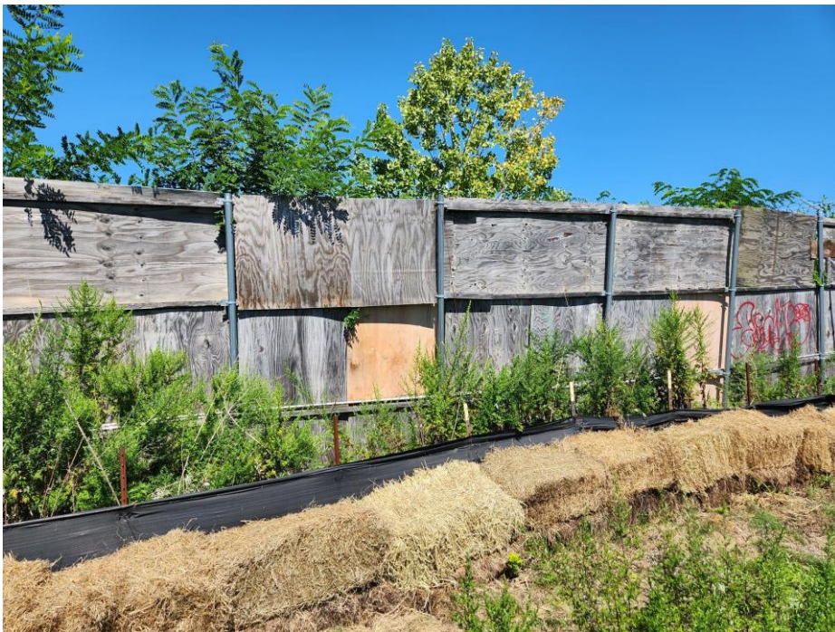
Photo 9: View of repaired perimeter fencing along the northern site boundary, facing northeast (taken on 08/25/2023)
