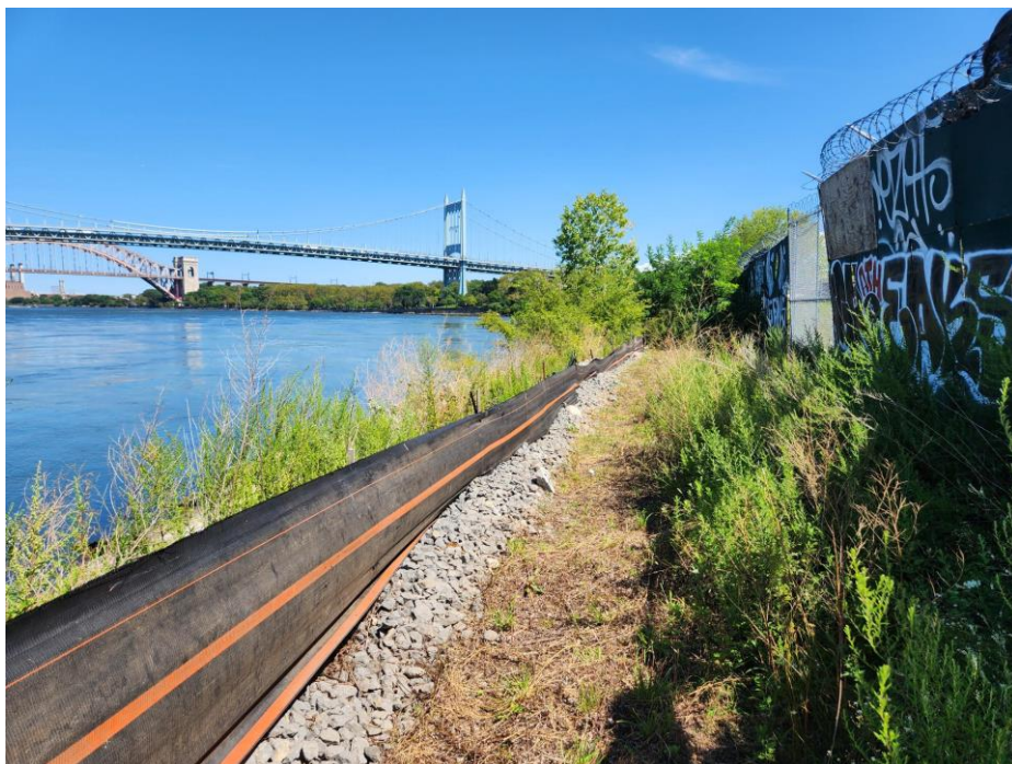
Photo 10: View of repaired silt fence along the river edge, facing east (taken on 08/25/23)
