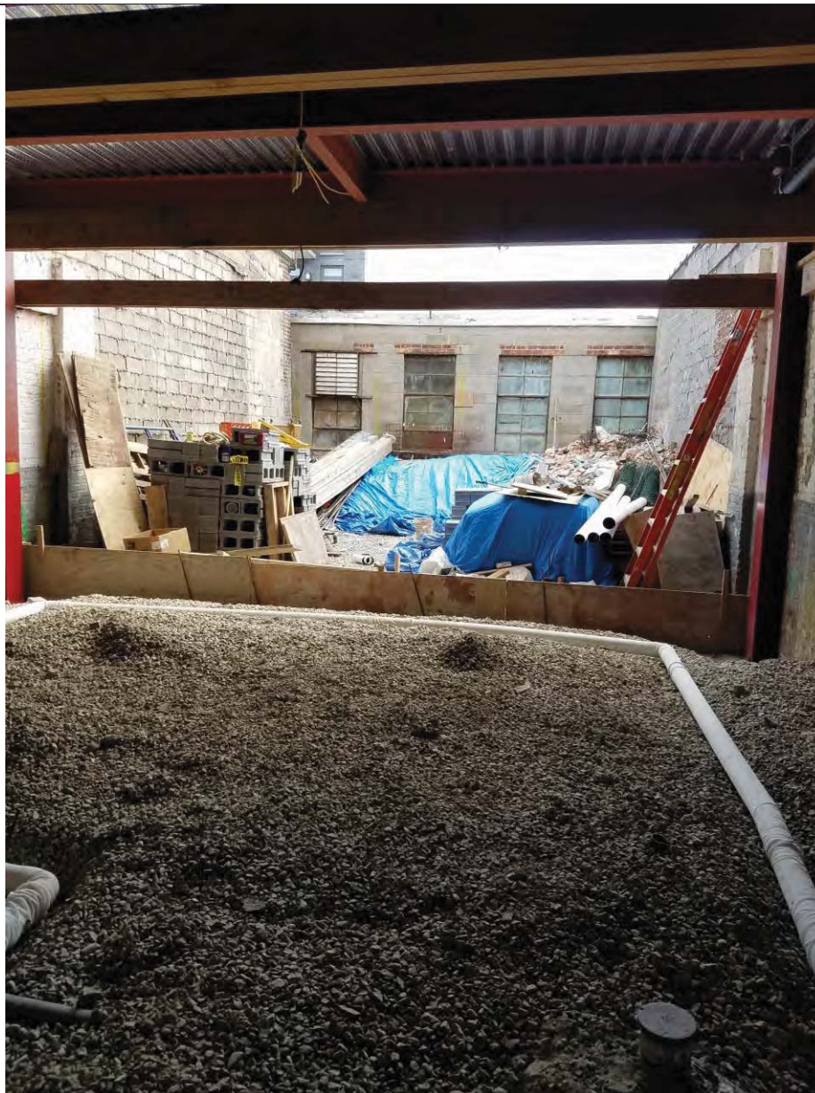
Photo 2– View of Site, Rear Yard, and SSDS Pipe
