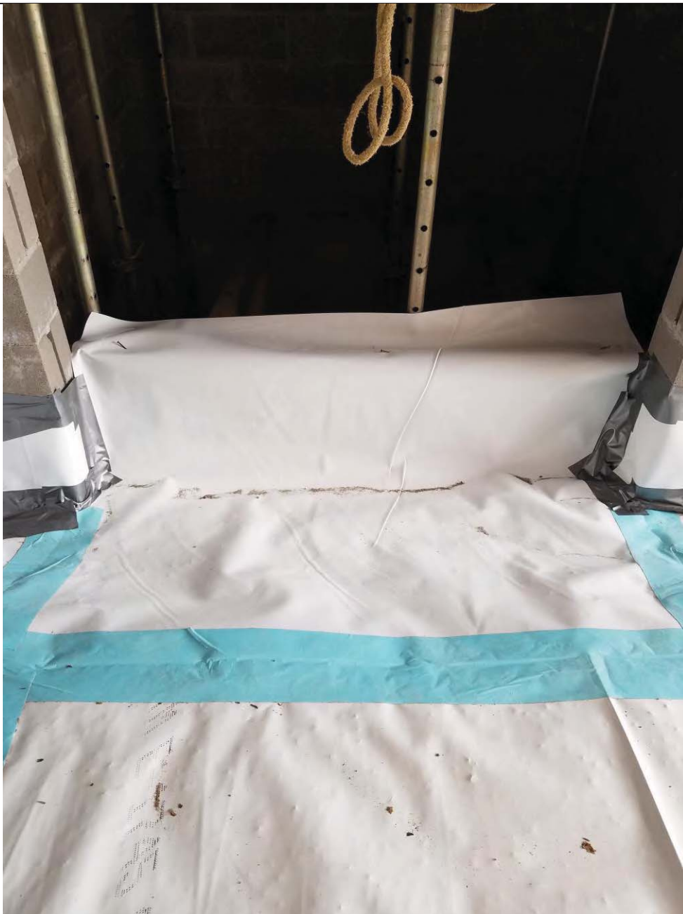
Photo 2– Vapor barrier near elevator pit
