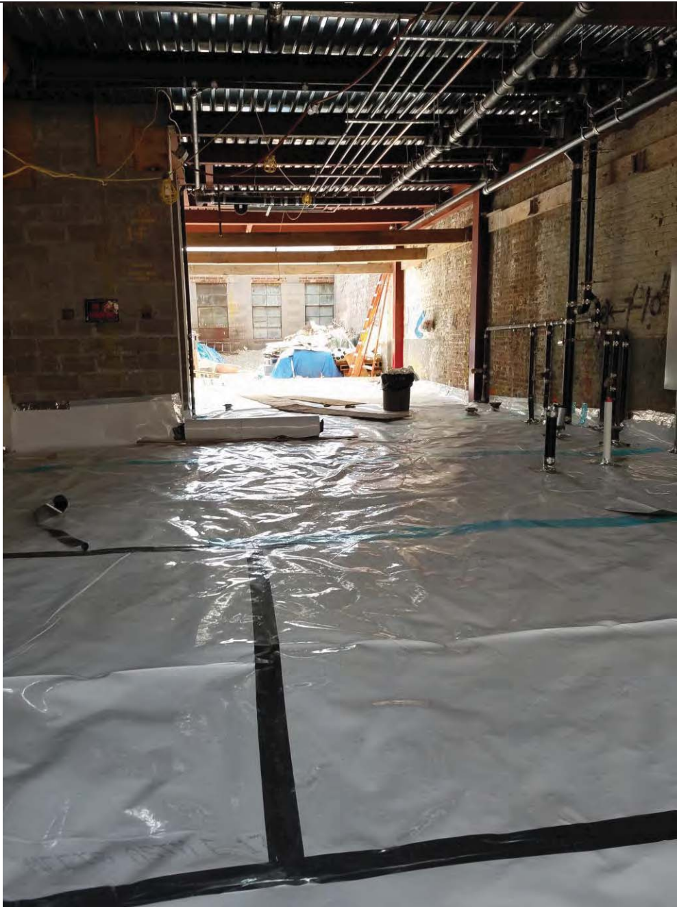
Photo 1 – View of vapor barrier across entire site
