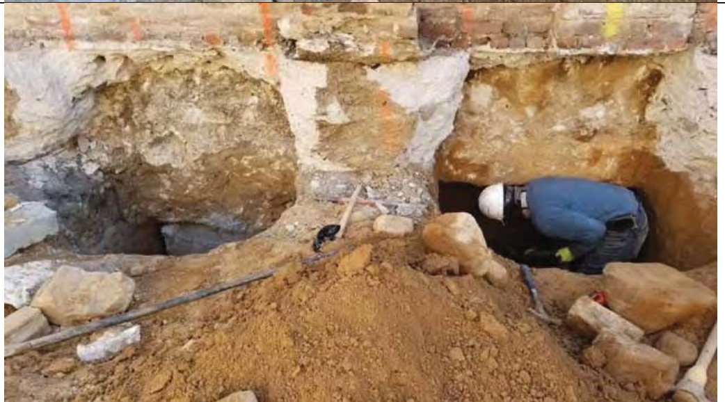
View of underpinning pits
