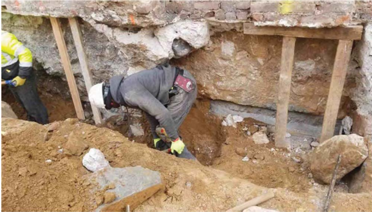
Hand excavation of underpinning pits
