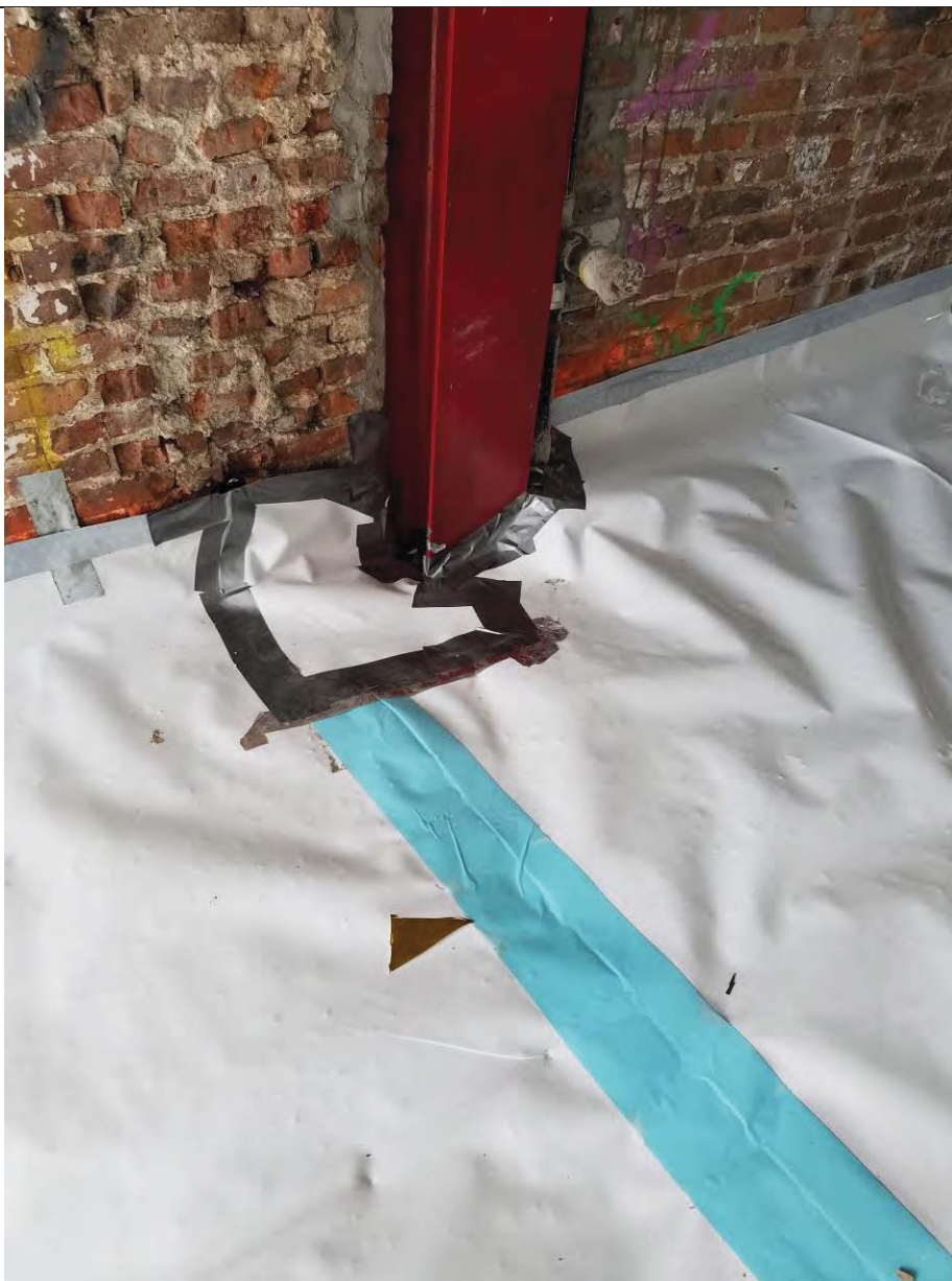
Photo 3— Tape used to secure vapor barrier and prevent opening from forming in between barrier pieces
