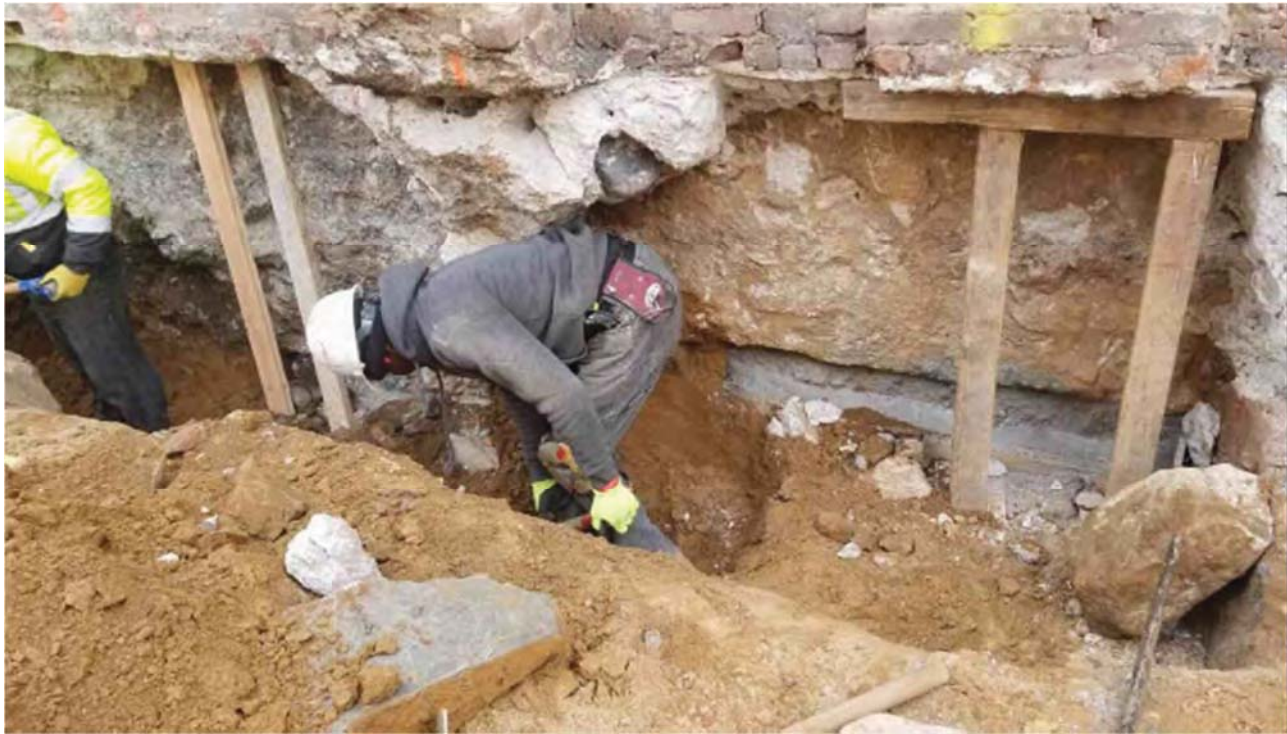
Hand excavation of underpinning pits
