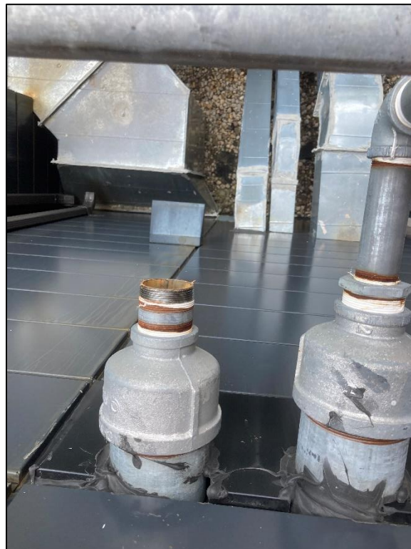
Photo 20, 07/06/2022: View of the disconnected SMD riser piping roof penetration connecting to the deficient blower.
