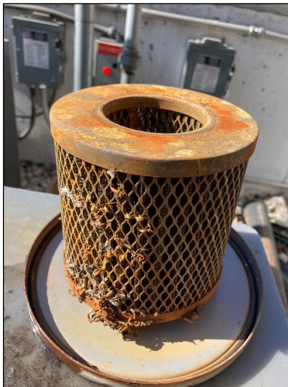
Photo 5, 02/16/2022: View of filter attached to north SMD blower.
