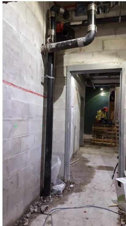
Photo 6, 03/16/2017: View of SMD riser pipe penetration through cellar slab (facing north).
