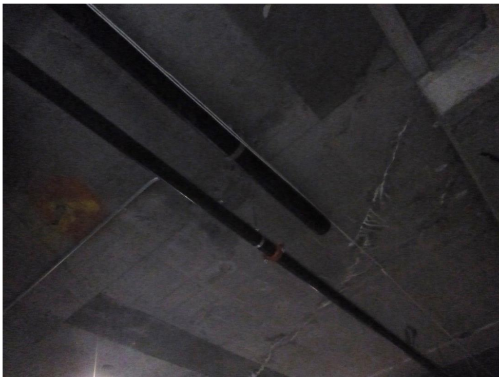
Photo 4, 03/01/2017: View of SMD riser pipes partially installed along the cellar ceiling (facing south).
