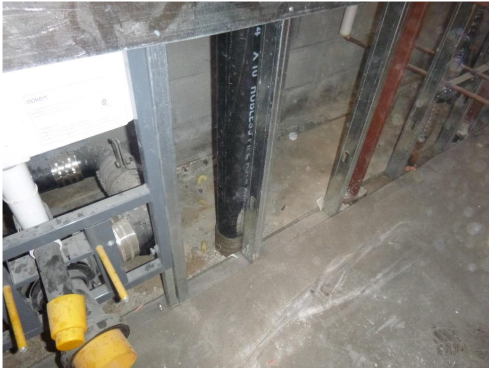
Photo 3, 03/01/2017: View of submembrane depressurization (SMD) system riser pipe penetration through the cellar slab (facing northeast).
