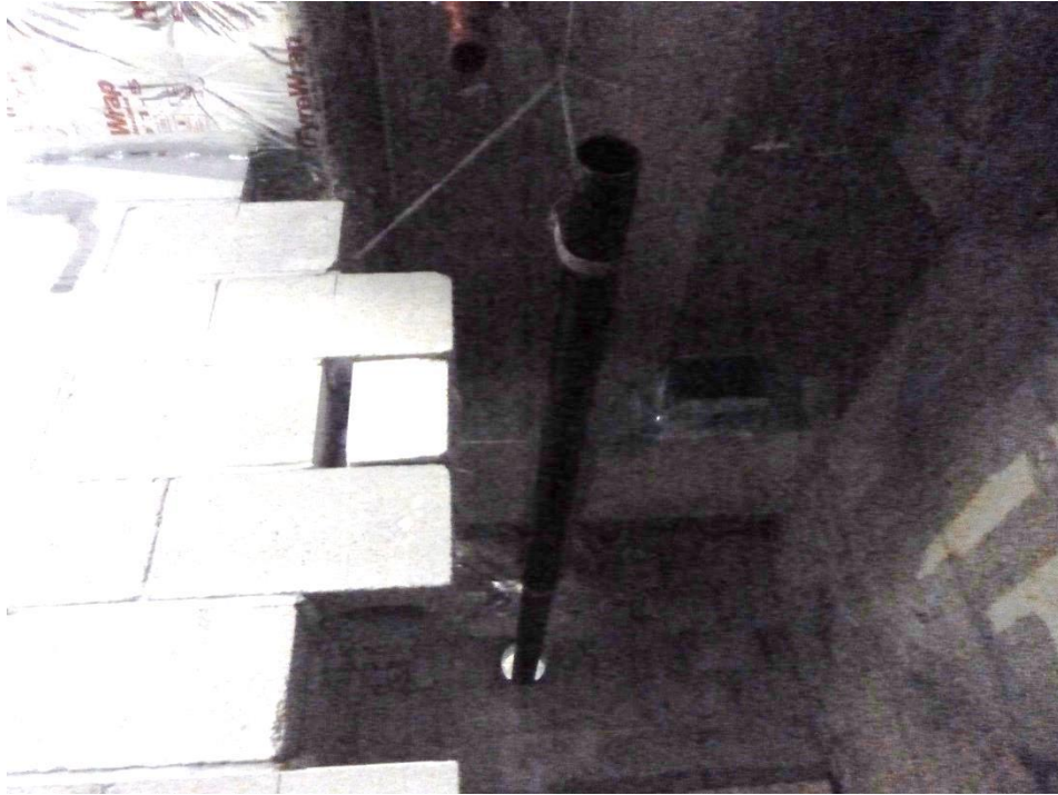
Photo 5, 03/01/2017: View of metal riser conveyance pipes partially installed within in the cellar ceiling (facing west).
