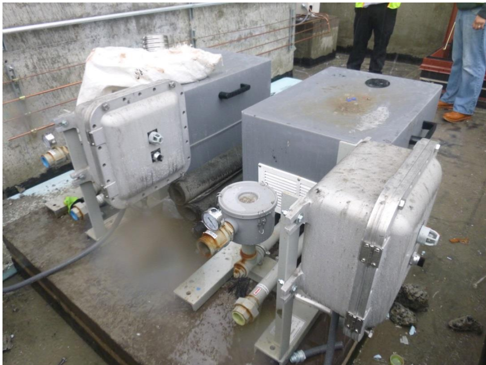
Photo 16, 03/01/2017: View of SMD blowers installed on the building roof (facing southeast).
