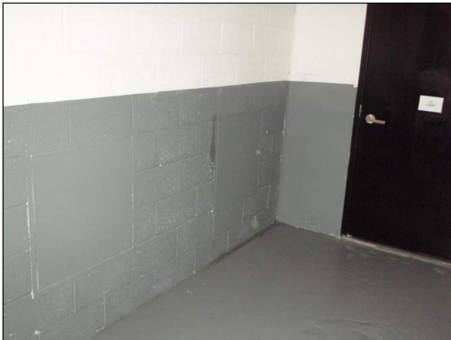
Photo 18, 12/19/2018: View of SMD system riser pipe access hatches in maintenance hallway (facing northwest).
