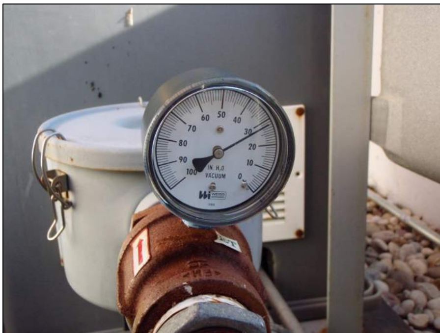
Photo 4, 12/19/2018: View of vacuum gauge connected to roof blower (facing east).
