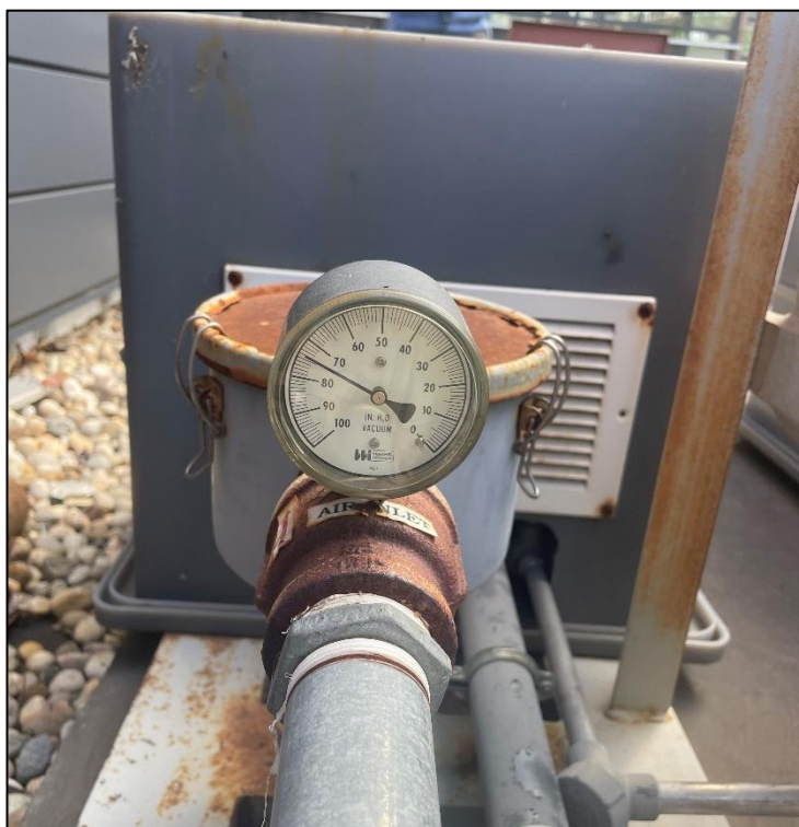
Photo 4, 05/17/2023: View of vacuum gauge connected to roof blower (facing east).
