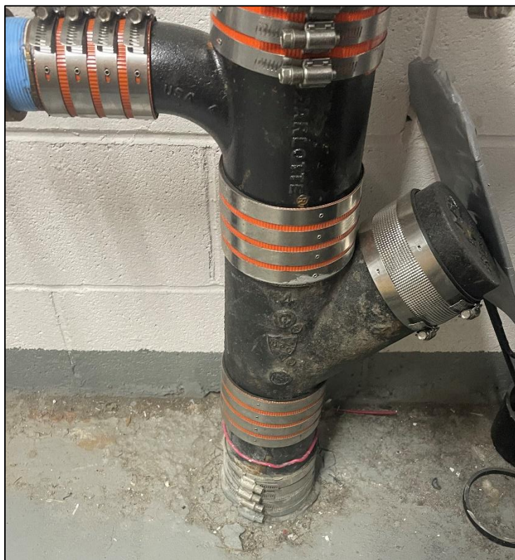
Photo 21, 05/17/2023: View of SMD riser behind maintenance hallway wall panel.
