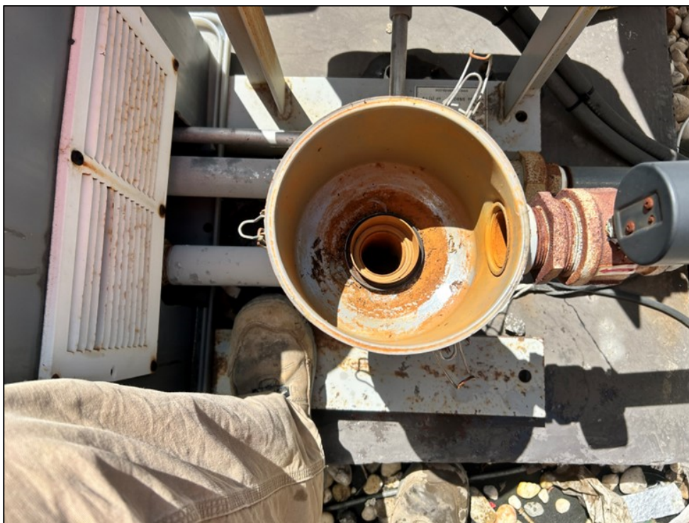
Photo 8, 05/28/2024: View within the filter segment of the south blower.
