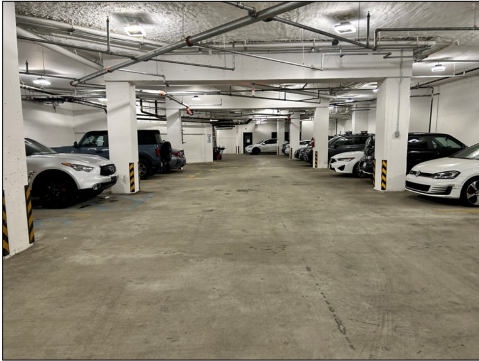
Photo 9, 05/28/2024: View of concrete building slab composite cover in ventilated parking garage (facing east).
