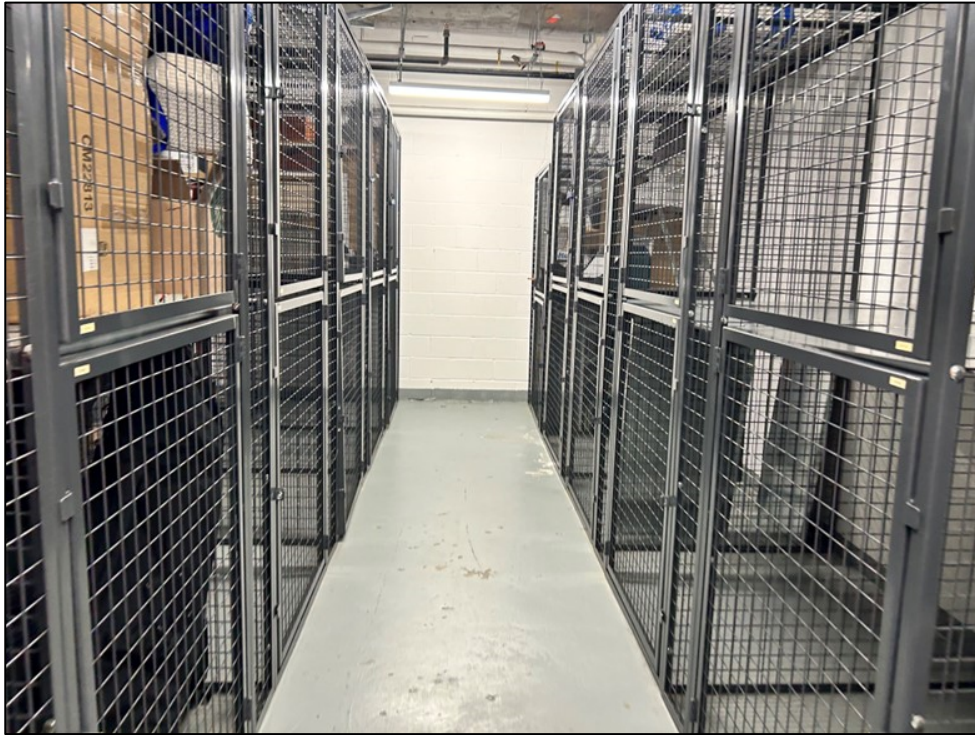
Photo 13, 05/28/2024: View of composite cover in resident storage room (facing west).
