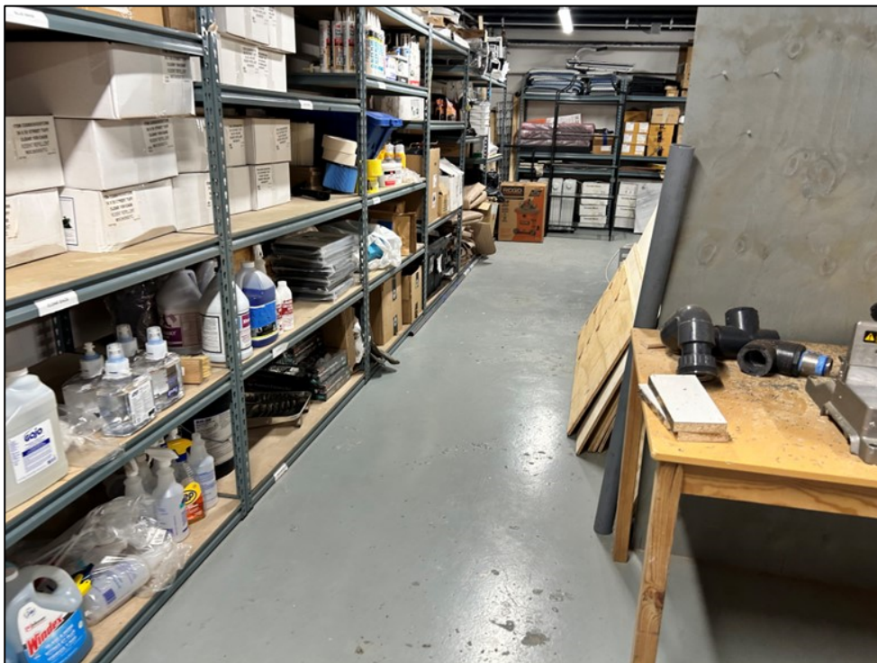
Photo 17, 05/28/2024: View of composite cover in supply room (facing south).
