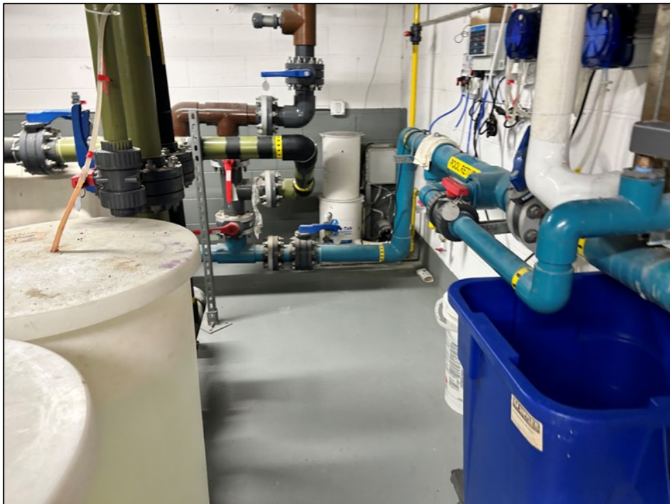
Photo 16, 05/28/2024: View of composite cover in pool storage room (facing south).
