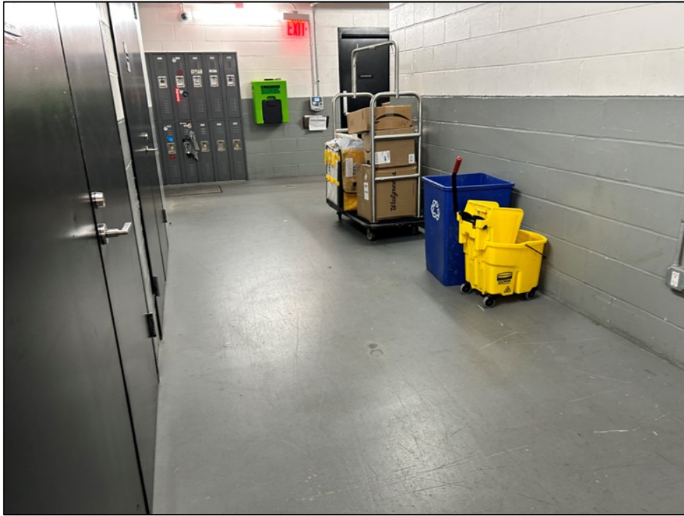
Photo 23, 05/28/2024: View of composite cover in maintenance hallway (facing east).
