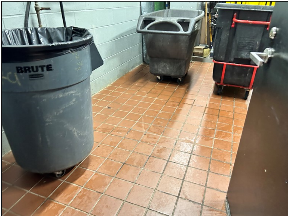
Photo 14, 05/28/2024: View of composite cover in compactor room (facing southeast).
