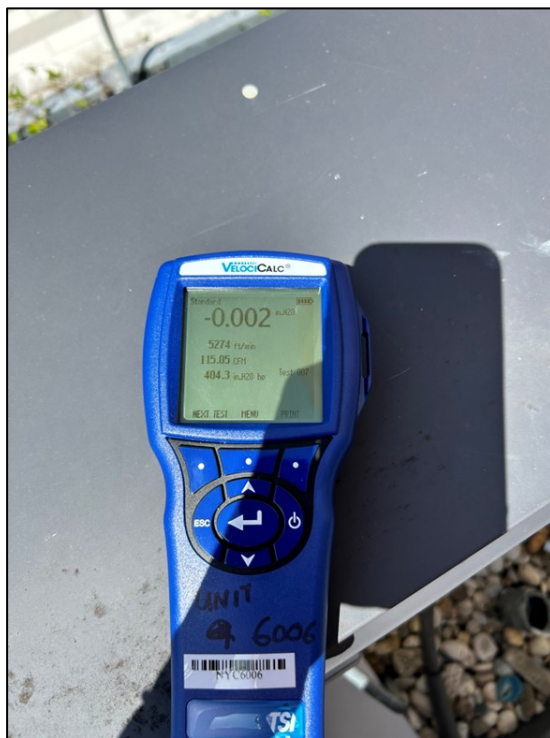
Photo 6, 05/28/2024: View of flow readings collected from the south blower (facing northwest).
