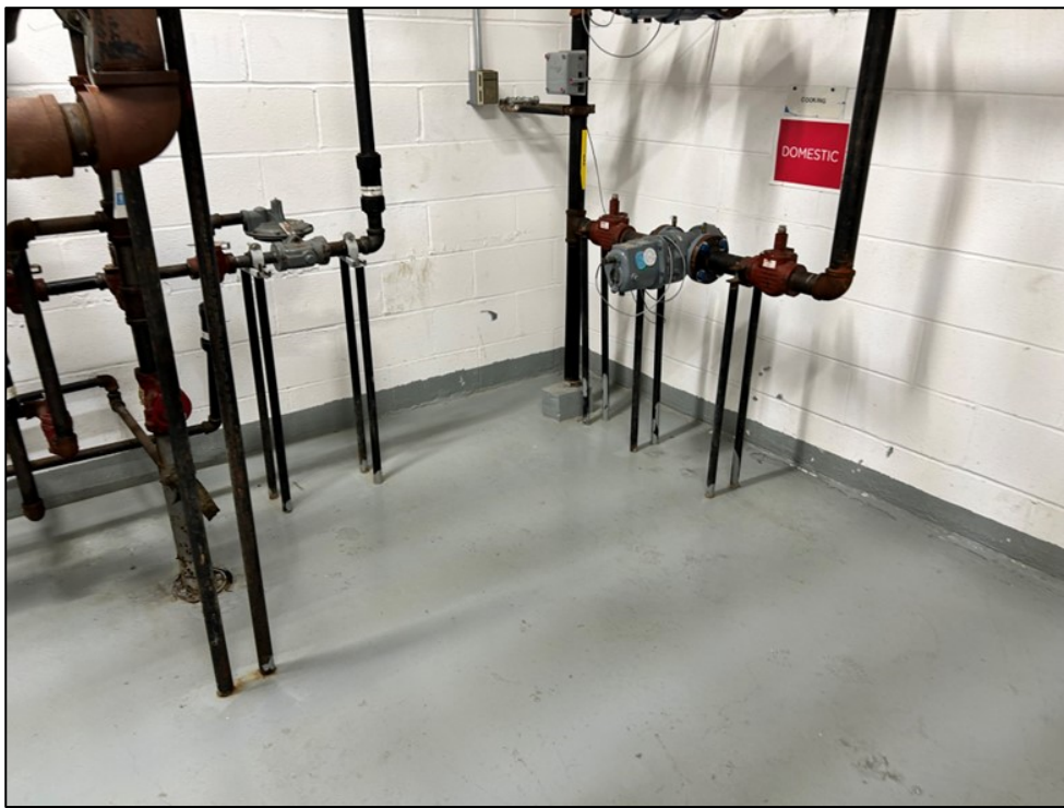
Photo 10, 05/28/2024: View of concrete building slab composite cover in gas meter room (facing northeast).
