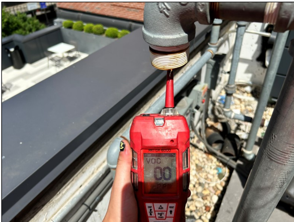
Photo 7, 05/28/2024: View of photoionization detector (PID) readings collected from the south blower (facing northwest).
