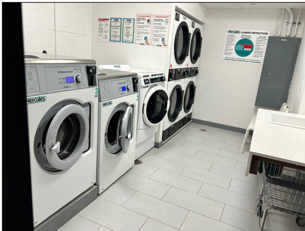
Photo 11, 05/28/2024: View of composite cover in laundry room (facing southwest).
