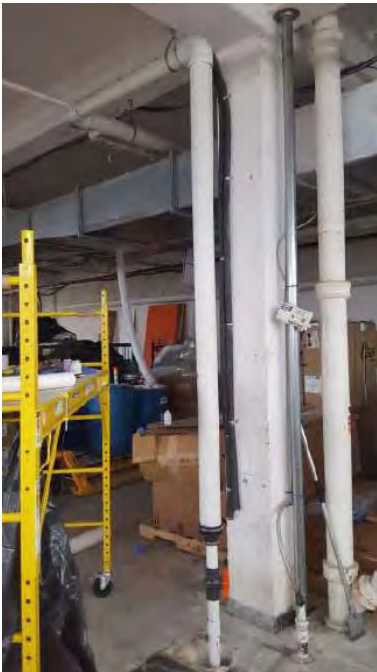
Photo 5 View of VE4 being installed
