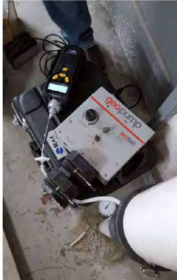
Photo 9 – Sampling of SVE system.
