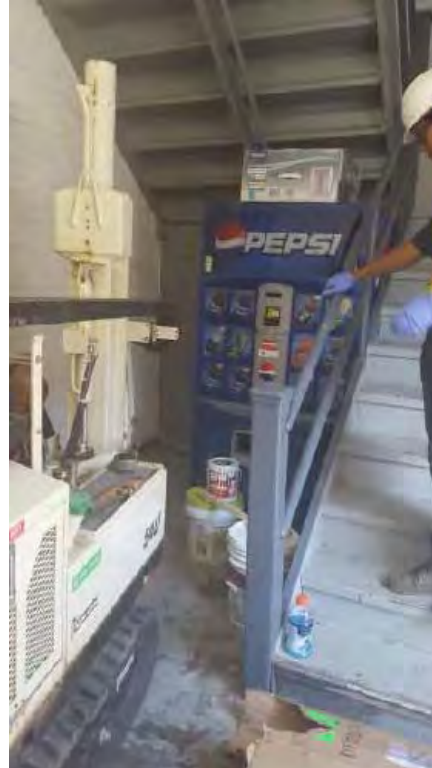
Photo 4 – View of soil sampling on 1 st floor.
