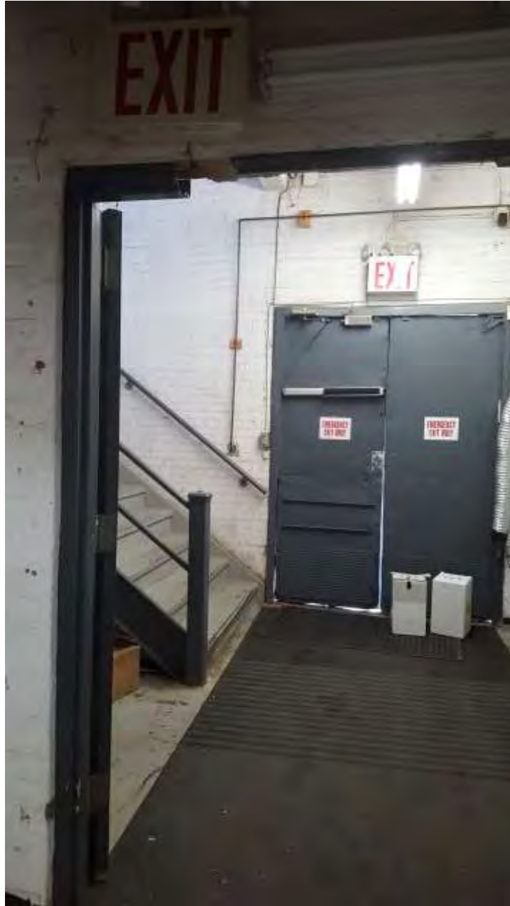
Figure 1 Doors closed for sampling
