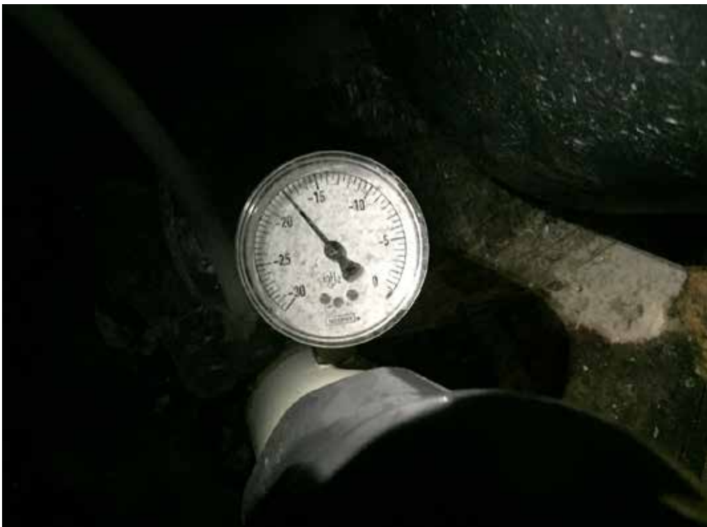
Photo 8: VE-3 vacuum dial showing -18 inches of water gauge.
