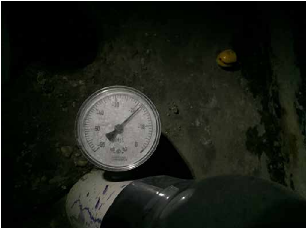
Photo 7: VE-2 vacuum dial showing -18 inches of water gauge.
