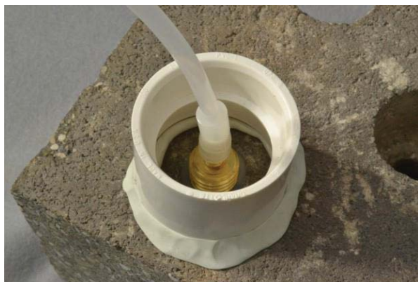
Figure 6. Water dam used for leak detection
