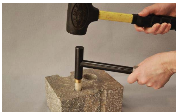
Figure 2. Installing the VAPOR PIN®
