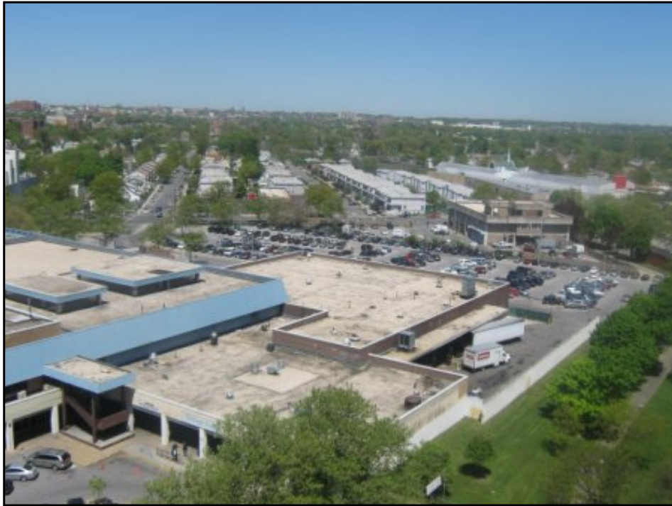
View of the larger shopping mall, and further to the north
