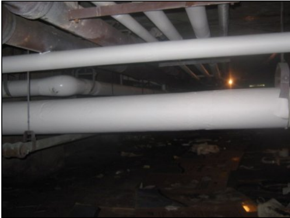
Crawlspace in the residential building that has recently been abated for asbestos- containing materials
