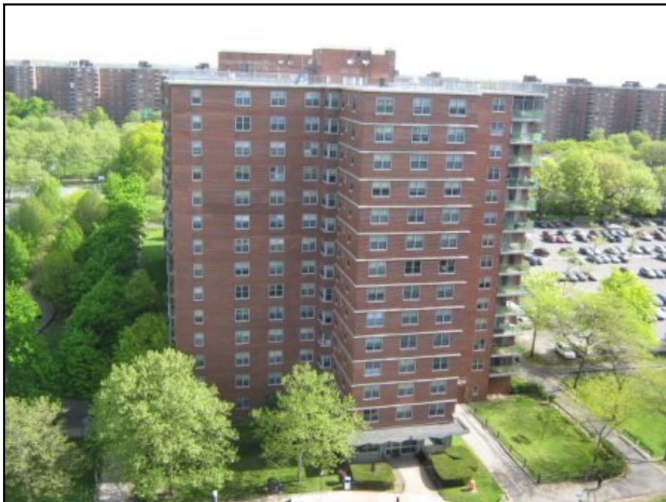
View of one of the residential buildings at Rochdale Village
