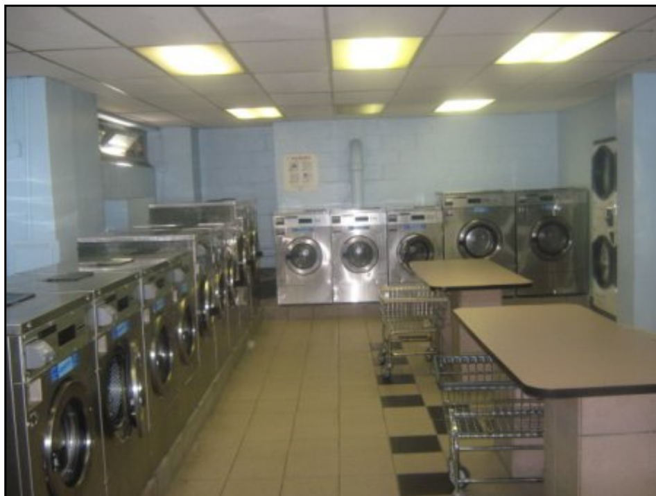
Typical laundry room
