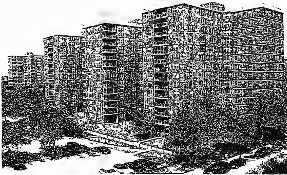
Photo 1: Building exterior, parking areas, and landscaping
