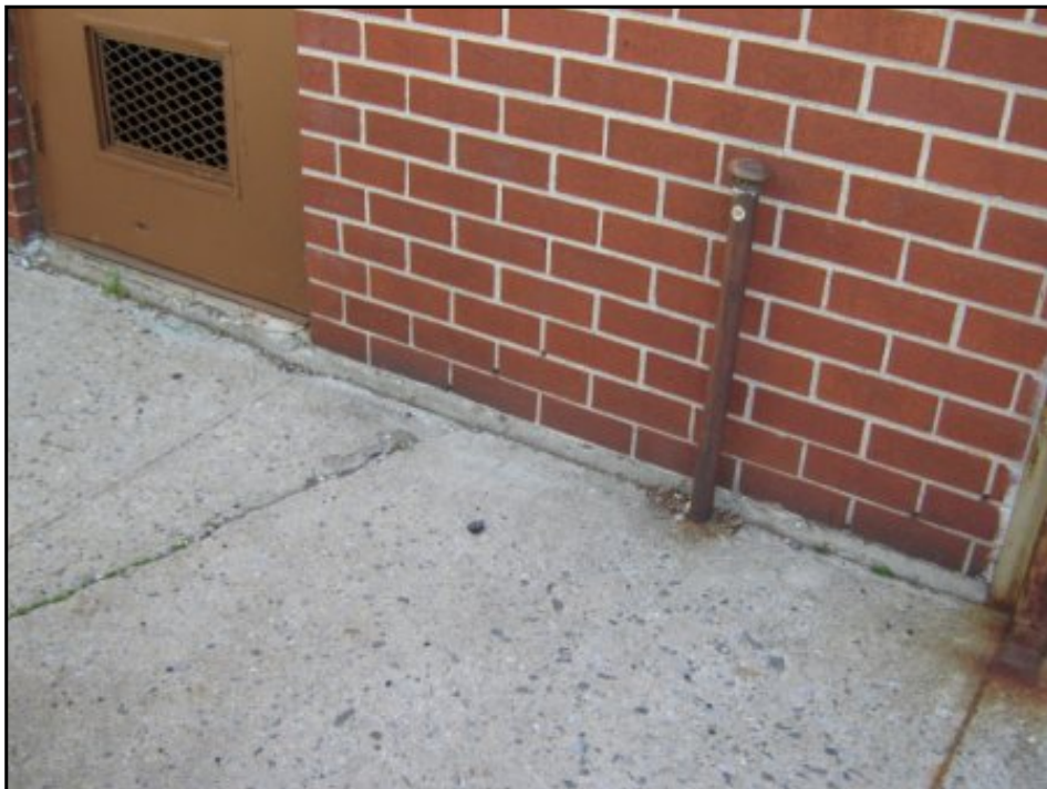
Vent pipe at the rear of HIP Cleaners
