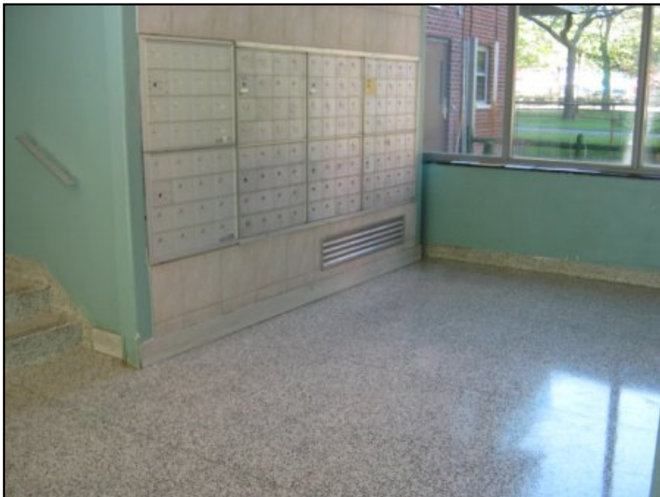
Typical common area finishes in residential building
