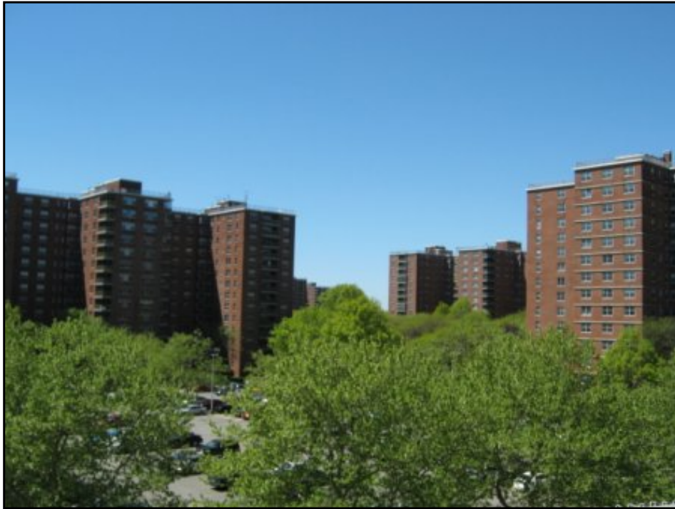
Rochdale Village taken from the roof of the power plant
