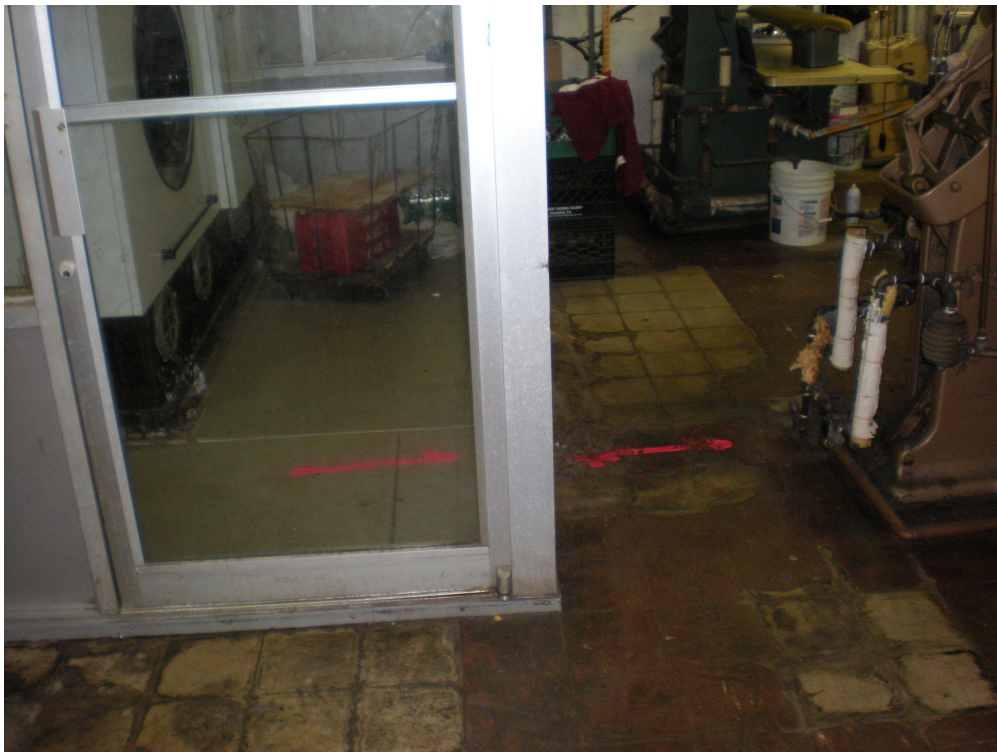
Figure 2 – Steam line designated with pink paint. Note the dry cleaning equipment and interior walls limiting the scope of the survey.
