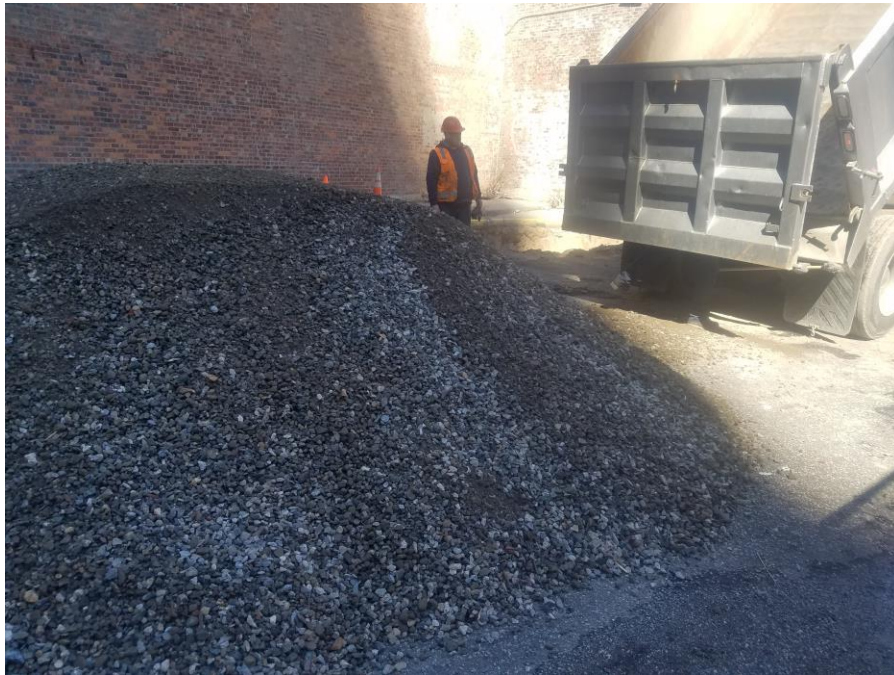
Photo 3: AARCO importing ¾-inch RCA from Evergreen Recycling of Corona (facing northwest).
