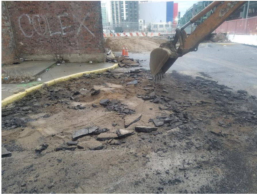
Photo 1: AARCO using an excavator to remove asphalt from the excavation area (facing north).
