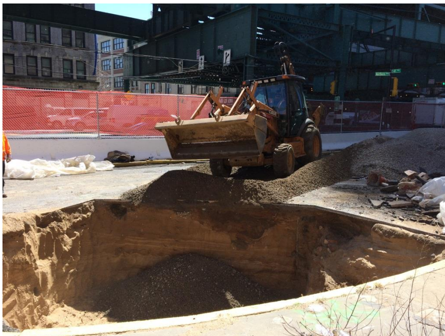
Photo 11: AARCO using imported RCA to backfill the excavation on Lot 10. (3/29/2017)
