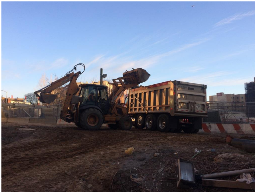
Photo 13: AARCO loading a truck with hazardous lead-impacted soil for off-site transport and disposal. (3/30/2017)
