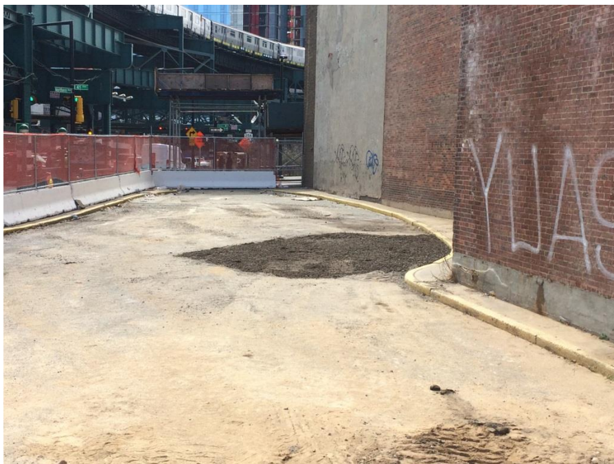
Photo 16: View of the backfilled excavation on Lot 10. (3/30/2017)
