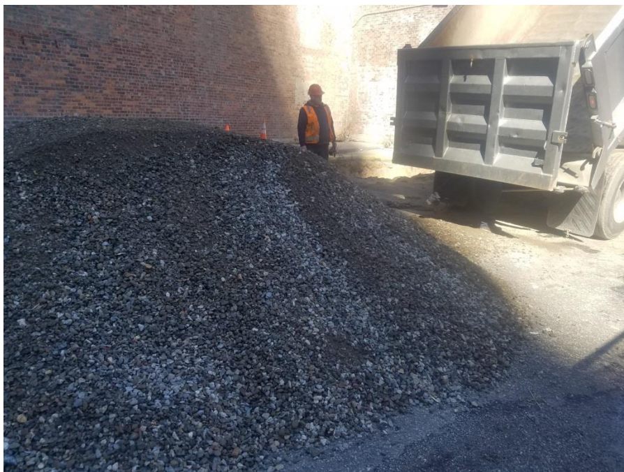
Photo 8: AARCO unloading imported recycled concrete aggregate (RCA) on Lot 10. (3/8/2017)
