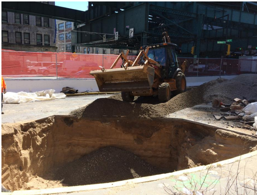
Photo 2: AARCO backfilling the excavation with imported RCA (facing east).
