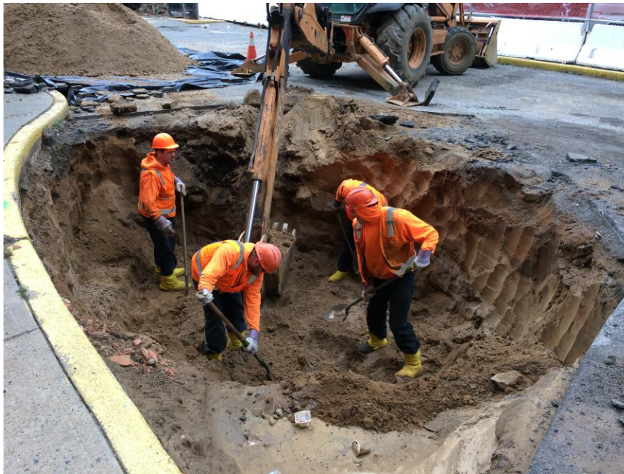
Photo 1: AARCO using shovels to excavate hazardous lead-impacted material (facing north).
