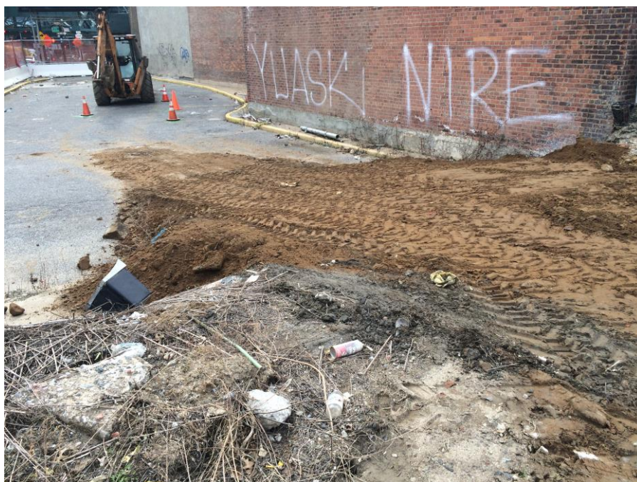
Photo 3: View of the ramp graded by AARCO to connect Lot 6 with Lot 10 (facing south).
