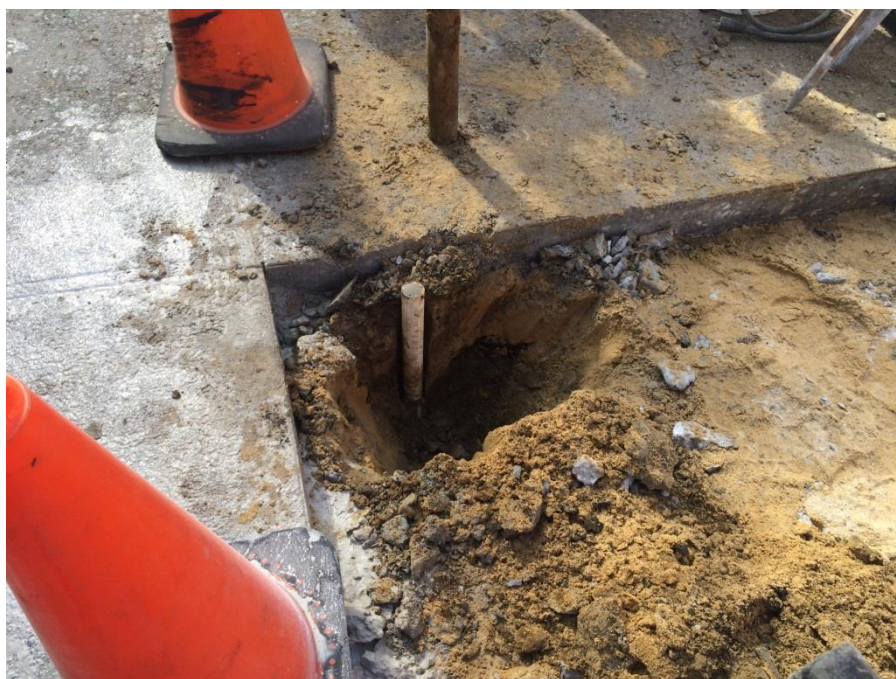
Photo 4: View of the polyvinyl chloride (PVC) pipe located beneath the fill port in the Northern Boulevard sidewalk. (2/28/2017)
