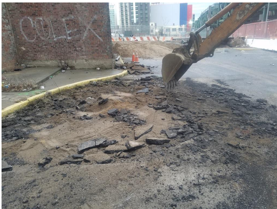
Photo 6: AARCO removing surface cover from the hazardous lead-impacted soil excavation area on Lot 10. (3/8/2017)
