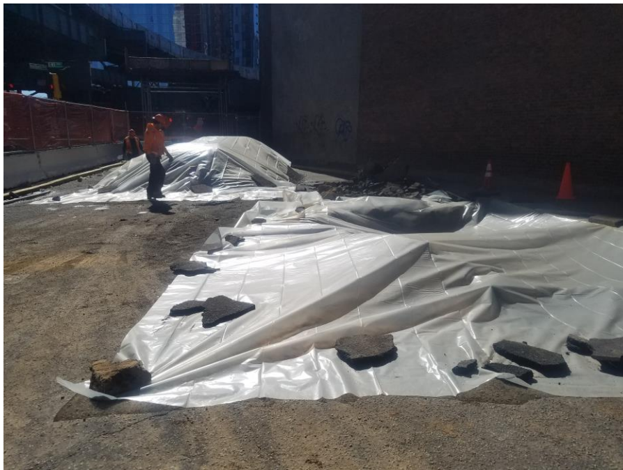
Photo 4: AARCO covering the open excavation and RCA stockpile with polyethylene sheeting (facing south).
