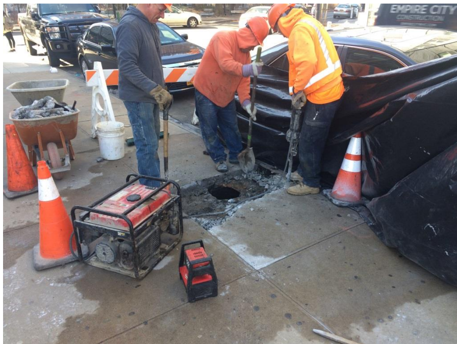
Photo 1: AARCO removing the sidewalk around the abandoned fuel oil fill port located in the 41 st Avenue sidewalk. (2/28/2017)
