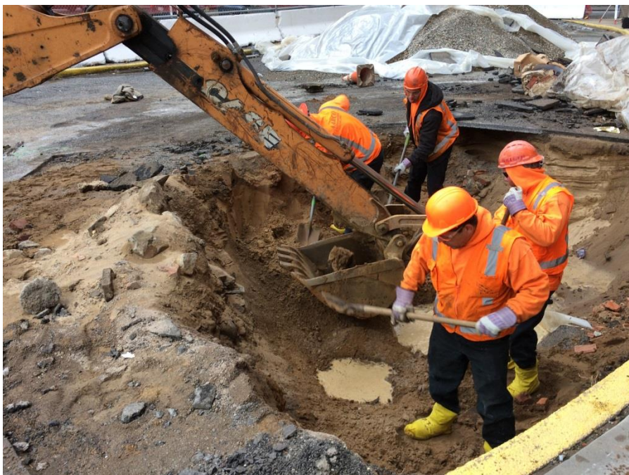
Photo 9: AARCO excavating hazardous lead-impacted soil using hand tools. (3/29/2017)
