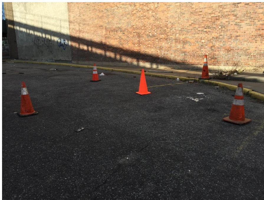
Photo 5: Placement of cones to mark-out the hazardous lead-impacted soil excavation on Lot 10. (2/28/2017)
