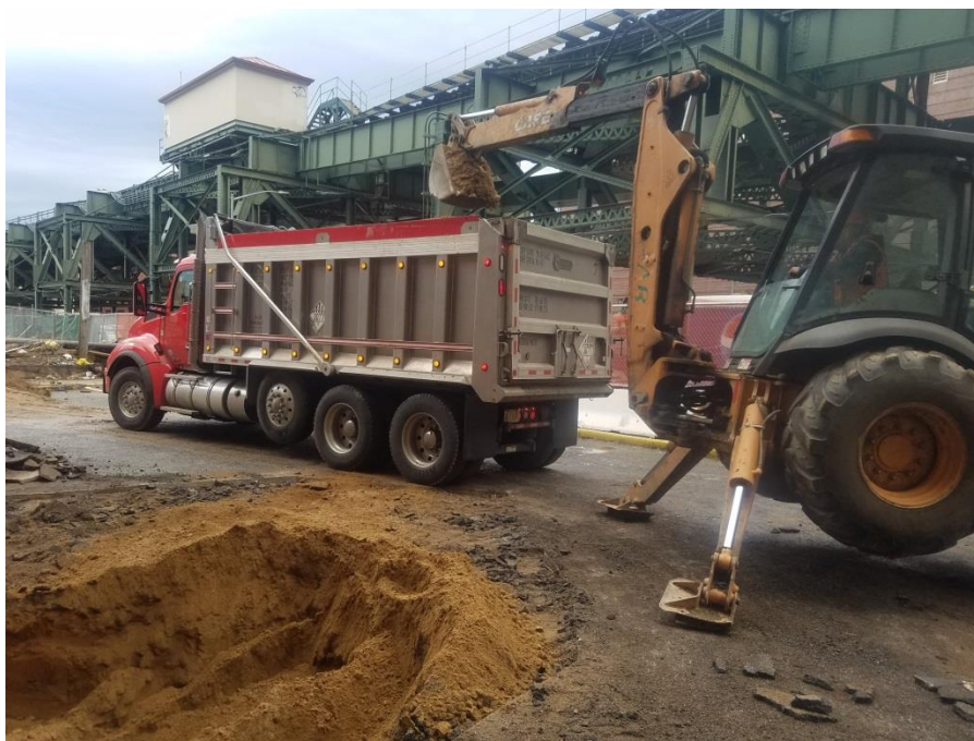
Photo 7: AARCO loading a truck with hazardous lead-impacted soil for off-site transport and disposal. (3/8/2017)
