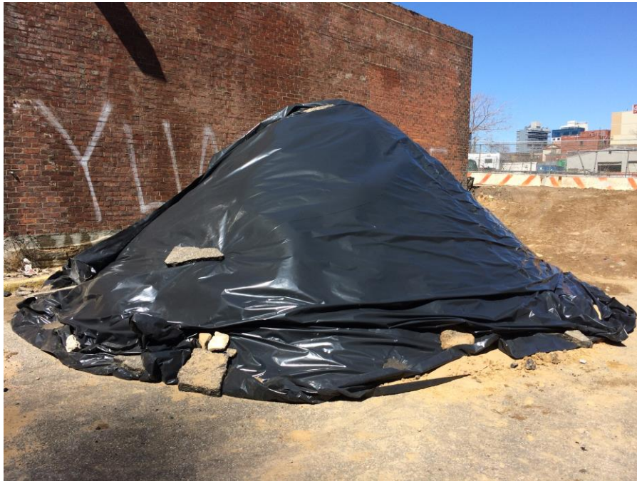
Photo 3: Stockpile of hazardous lead-impacted material sitting on top of and covered with polyethylene sheeting (facing northwest).
