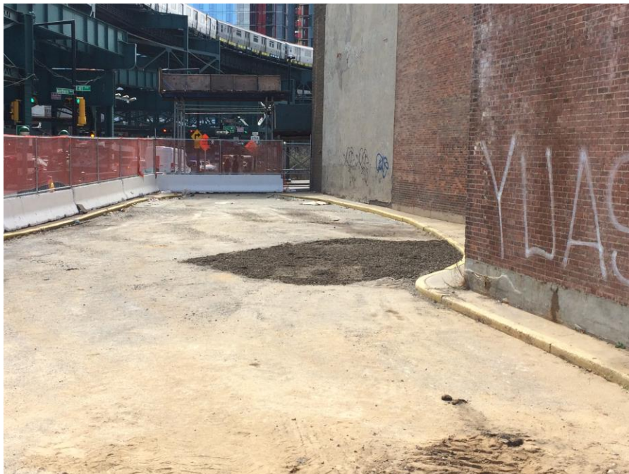
Photo 4: Backfilled and compacted area of excavation on Lot 10 (facing south).
