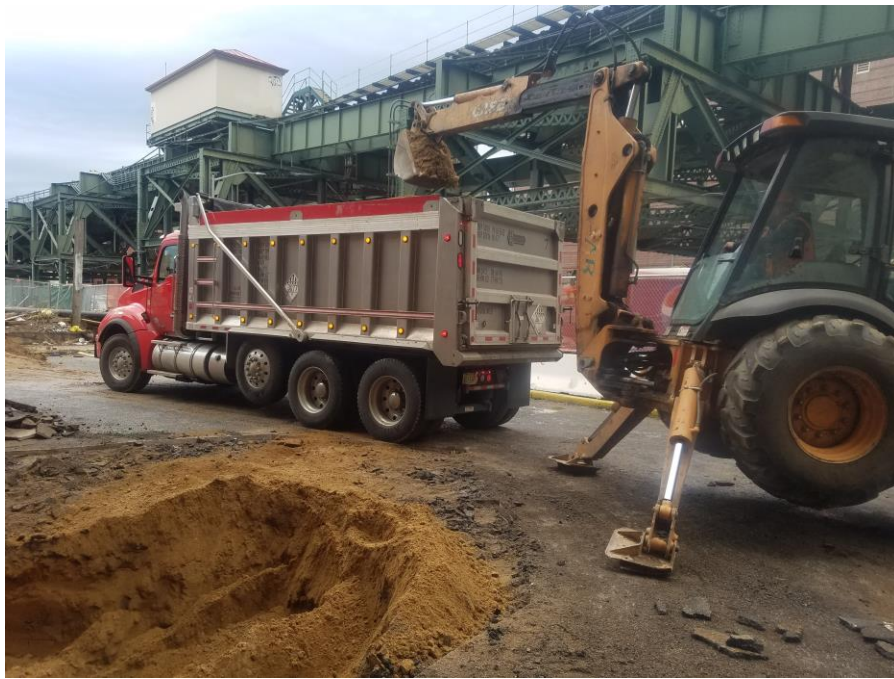
Photo 2: AARCO loading a truck with hazardous lead-impacted material (facing northeast).
