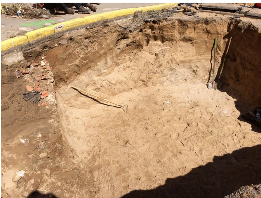
Photo 10: View of the hazardous lead-impacted soil area following excavation. (3/29/2017)
