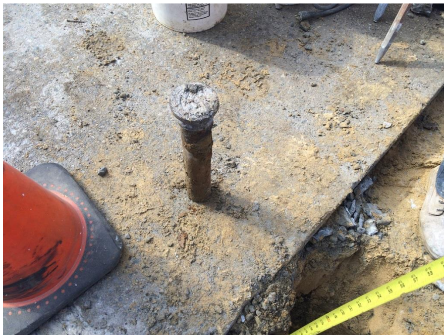
Photo 3: View of the fuel oil fill port removed from the Northern Boulevard sidewalk. (2/28/2017)
