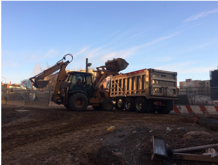
Photo 1: AARCO loading a truck with hazardous lead-impacted material (facing north).
