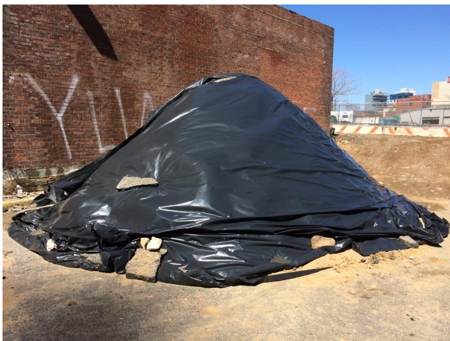
Photo 12: View of the covered stockpile of hazardous lead-impacted soil at the end of the workday. (3/29/2017)
