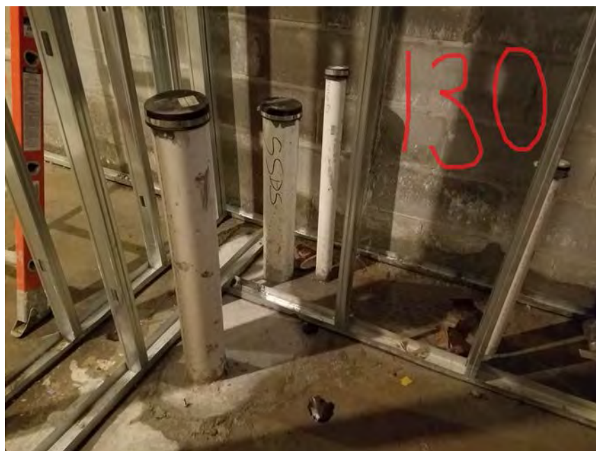
16. Condition and location of SSDS riser at Unit 130 in March 2018
