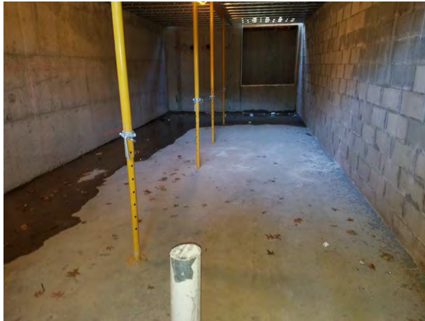
17. Condition and location of SSDS riser at Unit 150 in March 2018
