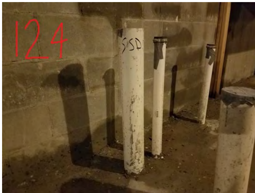
15. Condition and location of SSDS riser at Unit 124 in March 2018
