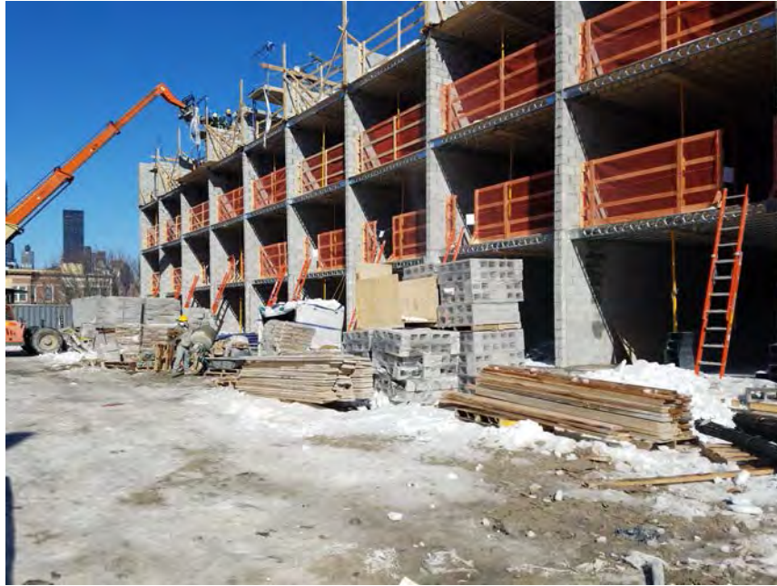
13. View northwest across interior courtyard showing site cover and progress of construction at rear of units along 45 th Road on March 17, 2017
