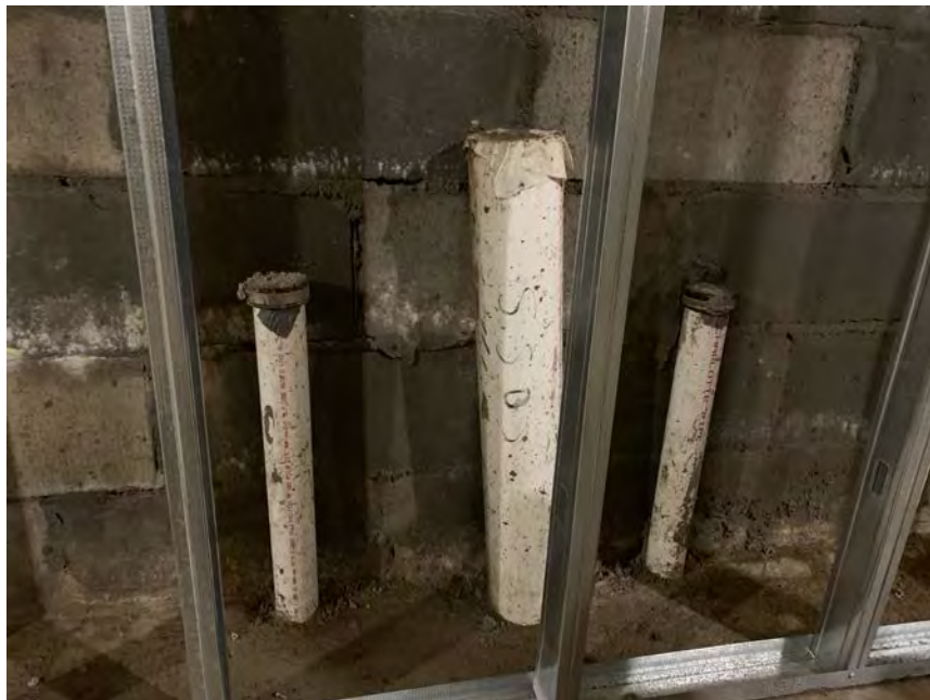
8. Condition and location of SSDS riser, Unit 148
