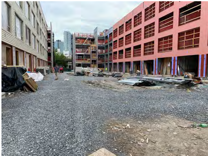
2. Cover system consisting of exposed soil and crushed blue stone, exterior courtyard area
