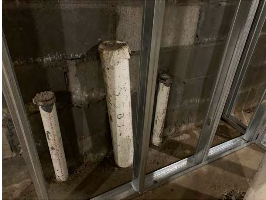
7. Condition and location of SSDS riser, Unit 140
