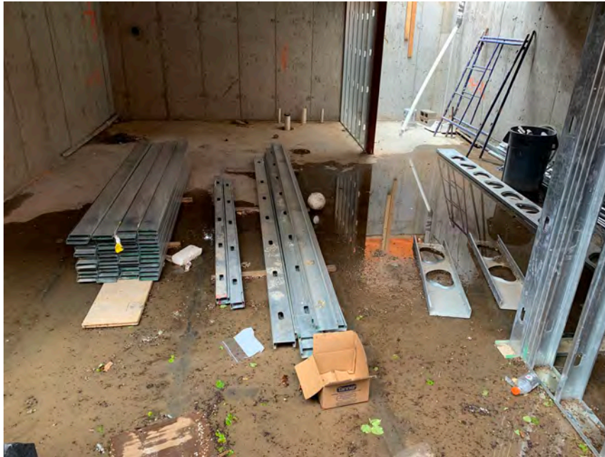
3. Concrete building slab at unit 134, observed to be in good condition
