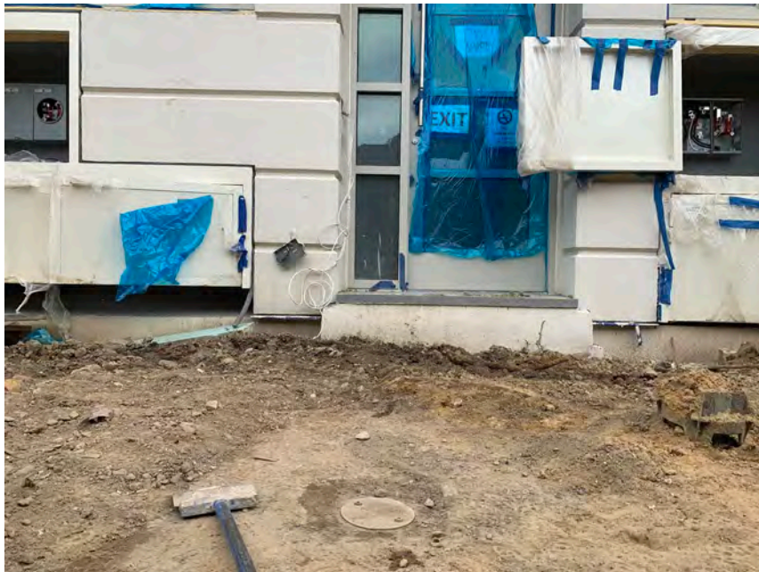
10. Off-site groundwater monitoring well (2MW-05) in good condition, along 45 th Road
