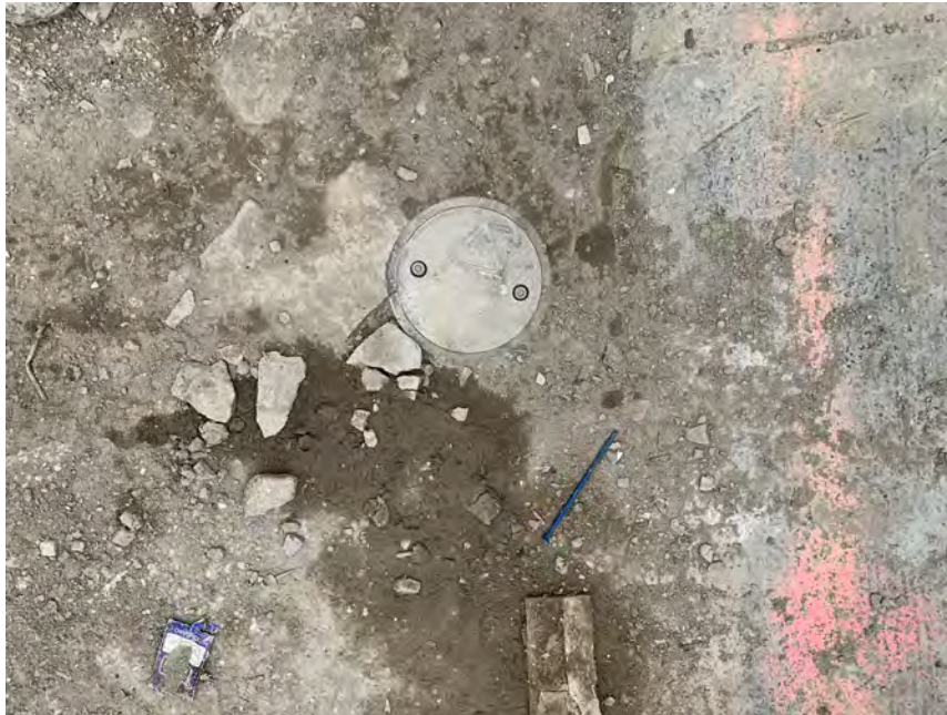
9. Off-site groundwater monitoring well (2MW-03) in good condition, along 45 th Road
