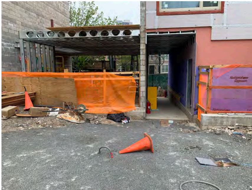
2. Construction at unit 134
