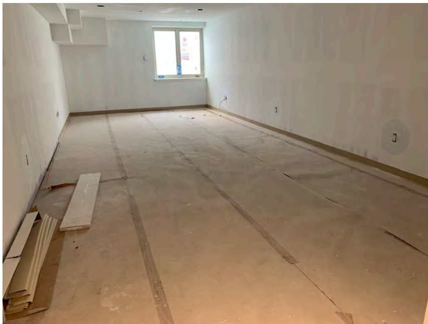
4. Typical cover system at building interior (concrete building slab, unit 127)
