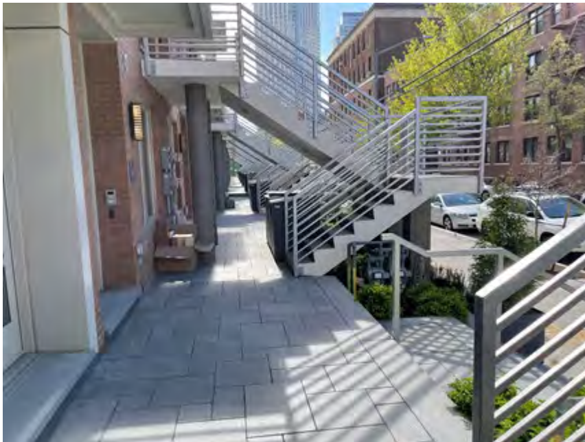
6. Typical cover system along 46 th Avenue (stone and pavement, overlying imported clean soil)
