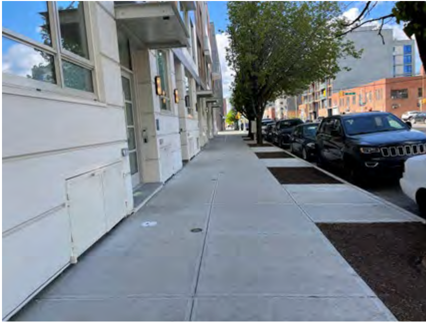
9. Off-site sidewalks along 45 th Road (newly retored)
