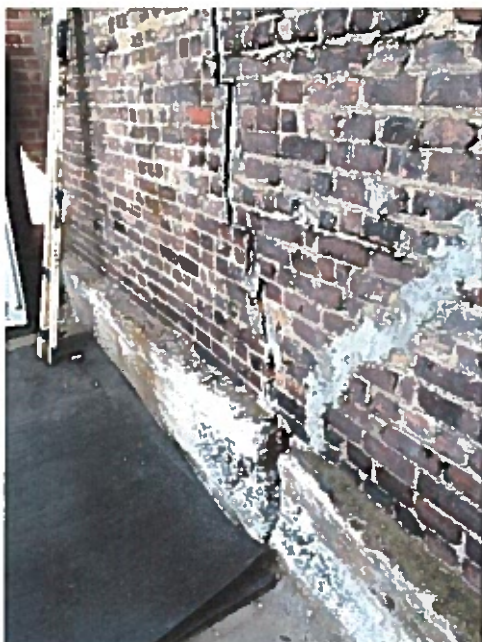
Condition of party wall, foundation and retaining wall
