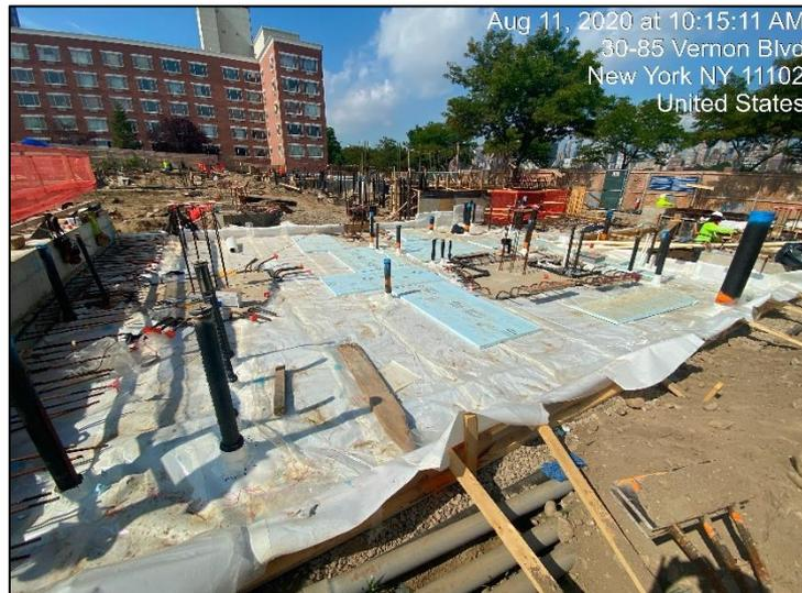
Photograph 11 – Installing the vapor barrier below the slab (August 2020)
