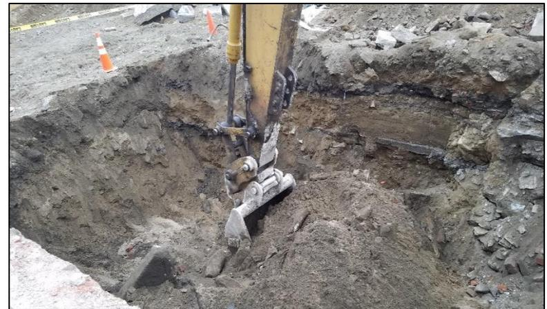
Photograph 4 – Petroleum-contaminated soil was excavated and removed following the tank removal (October 2018).
