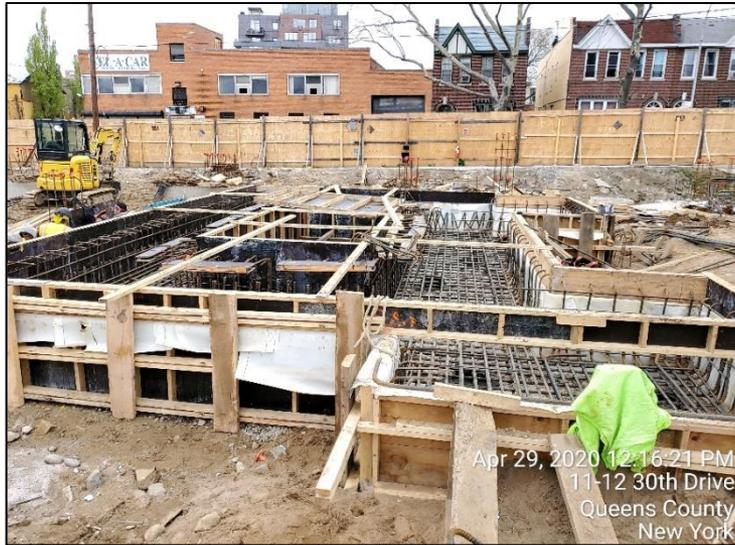
Photograph 9 – Installed GCP Preprufe 200 vapor barrier/waterproofing membrane below the foundation slab and behind subgrade foundation walls (April 2020).
