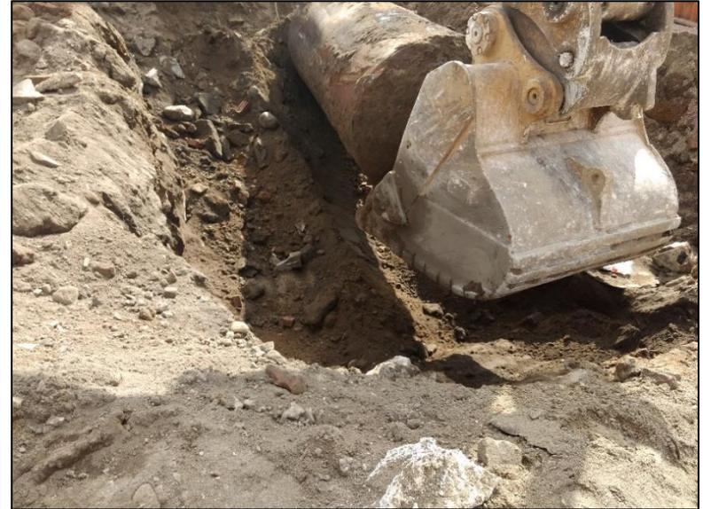
Photograph 2 – The tank was removed following removal of the oil-water mixture (October 2018).
