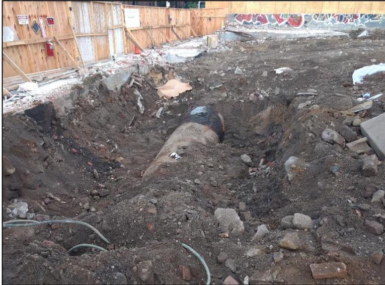
Photograph 1 – The underground storage tank (UST-1) was exposed for cleanup and removal (October 2018).
