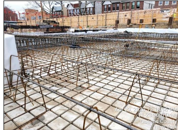
Photograph 10 – Installed GCP Preprufe 200 vapor barrier/waterproofing membrane below the foundation slab and behind subgrade foundation walls (April 2020).
