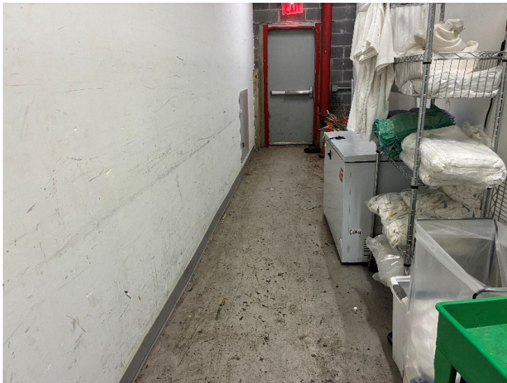
Photograph 3: Utility hallway showing concrete slab.
