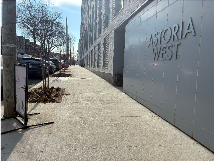
Photograph 1: Building entrance along 30 th Drive, facing southwest.
