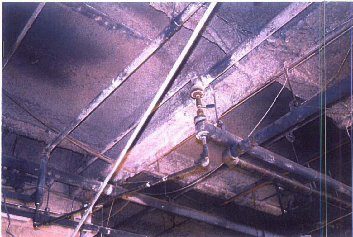
Sprayed-On Fire-Proofing, Suspect ACM
