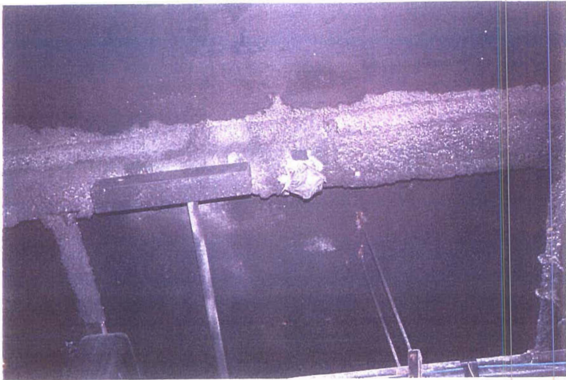
Sprayed-On Fire-Proofing, Suspect ACM
