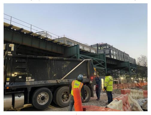
Photo 2: ECD installing a tarp and bungees on a disposal truck prior to departure (facing west).
