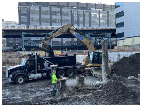
Photo 1: ECD loading hazardous lead-impacted soil/fill from HS-6 into a truck (facing north).
