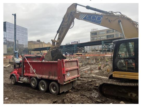
Photo 2: ECD live-loading a disposal truck with hazardous soil/fill from WCG COMP K2 (facing southwest).
