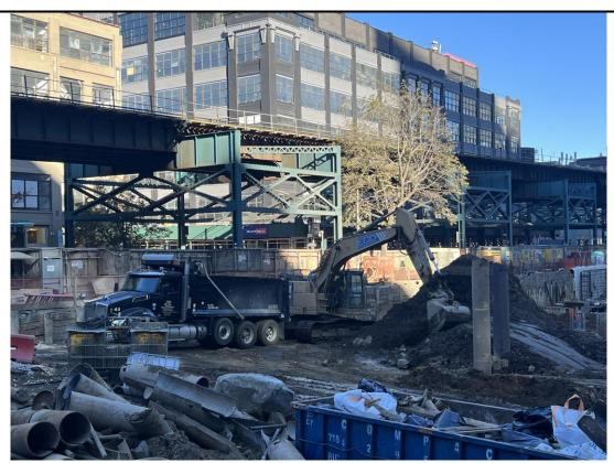
Photo 3: ECD loading a truck with non-hazardous soil/fill from WCG COMP F & B (facing northwest).
