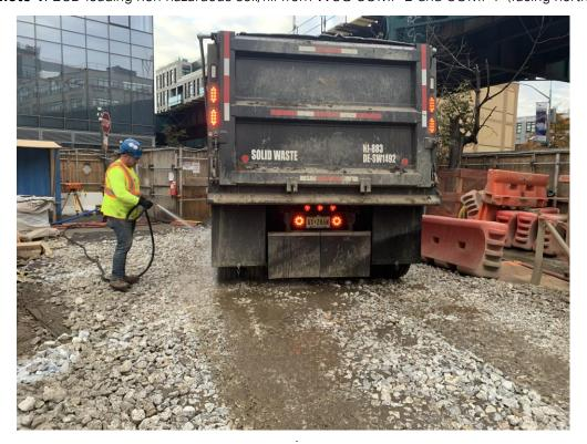
Photo 2: ECD washing truck tires in exit ramp (facing northwest).
