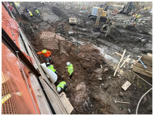
Photo 4: ECD installing lagging in WCG COMP K (facing down).
