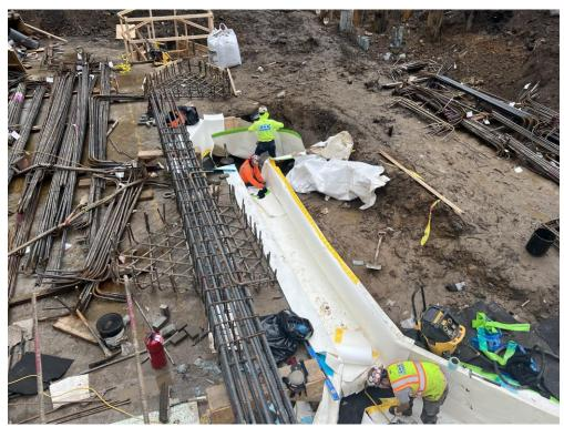
Photo 4: ECD installing vapor barrier in WCG COMP D (facing east).
