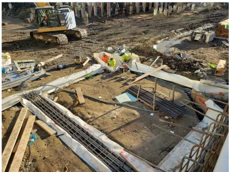
**Photo 4**: ECD installing GCP Preprufe vapor barrier and GCP Bituthene liquid membrane along pile caps in WCG COMP C (facing south).
