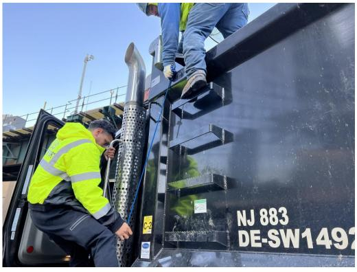
Photo 2: ECD installing bungees and a tarp on a disposal truck prior to departure (facing southwest).
