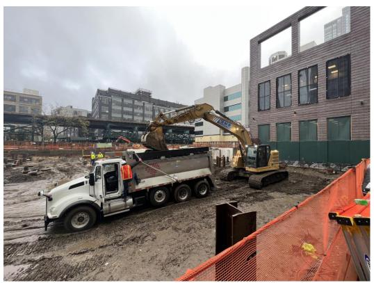
Photo 3: ECD live loading hazardous soil/fill from COMP K2 into a disposal truck (facing north).
