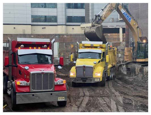
Photo 2: ECD loading non-hazardous soil/fill from WCG COMP C into a disposal truck (facing northeast).
