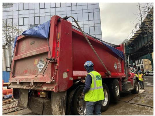
Photo 3: ECD applying a tarp and bungees to a disposal truck preparing to leave the site (facing southwest).
