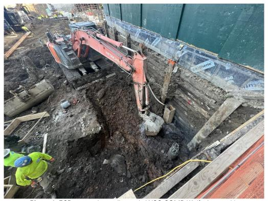
Photo 4: ECD excavating a pile cap in WCG COMP K2 (facing north).
