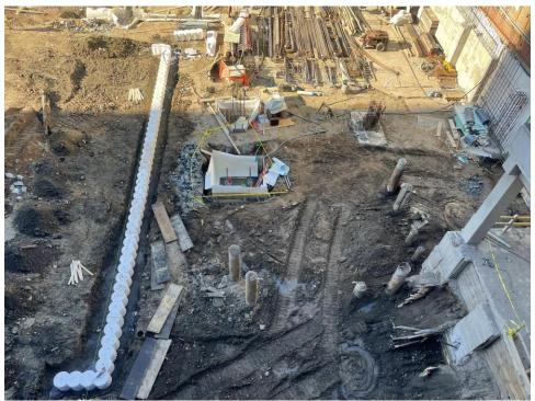
Photo 3: ECD installing a soil mix wall and vapor barrier in WCG COMP H and COMP D (facing northwest).
