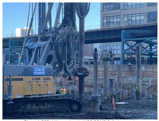
Photo 4: ECD drilling casings in WCG COMP G (facing west).
