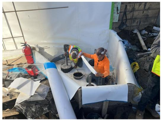
Photo 1: ECD installing vapor barrier in WCG COMP H (facing north).
