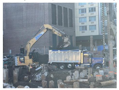
Photo 2: ECD loading hazardous lead-impacted soil/fill from HS-6 into a truck (facing northeast).
