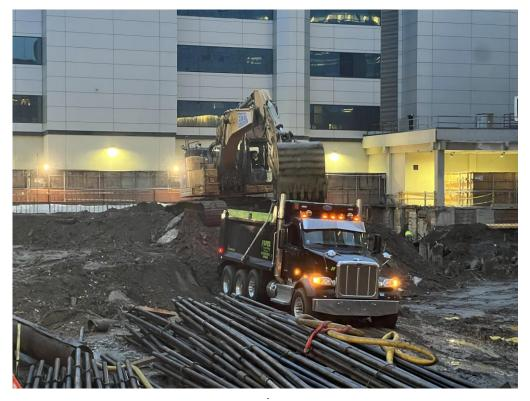
Photo 2: ECD loading non-hazardous soil/fill from the stockpile into a disposal truck (facing north).
