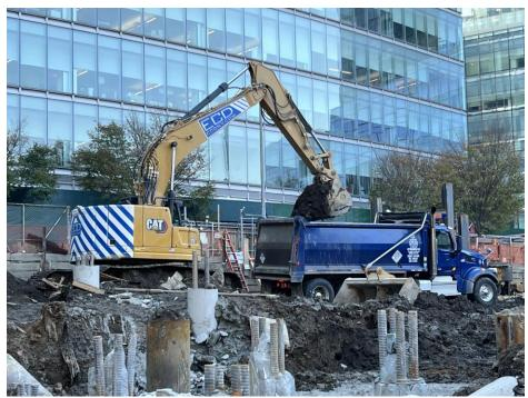
Photo 3: ECD loading hazardous soil/fill from WCG COMP G into a disposal truck (facing east).
