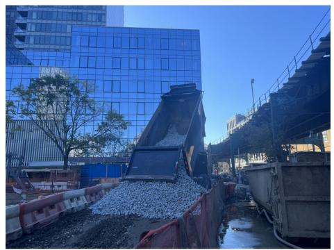
Photo 4: A truck dumping imported stone on the ramp in WCG COMP A (facing south).
