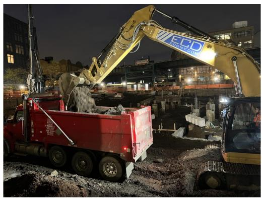
Photo 1: ECD live-loading non-hazardous soil/fill from WCG COMP J and K (facing west).
