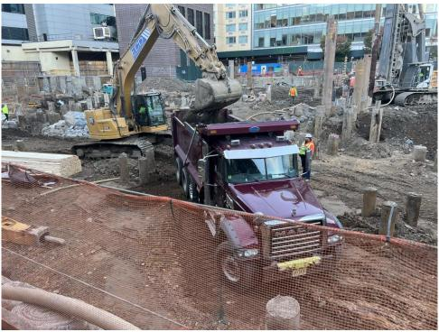
Photo 4: ECD loading C&D in a disposal truck (facing northeast).
