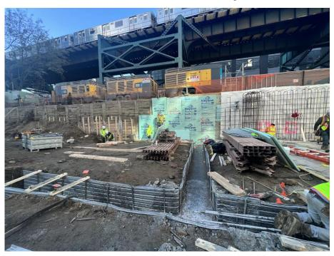
Photo 2: ECD installing a vapor barrier in WCG COMP C & D (facing west).
