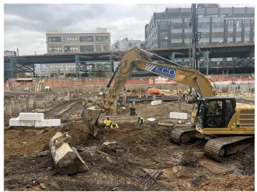
Photo 3: ECD excavating in WCG COMP K and J for soil mix wall installation (facing west).
