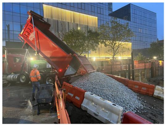
Photo 1: ECD importing tracking pad stone from Braen Aggregates, LLC (facing south).
