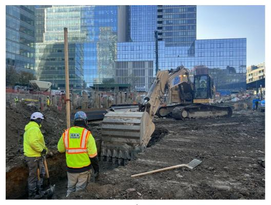
Photo 2: ECD excavating for soil mix wall installation in WCG COMP C (facing south).
