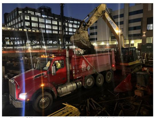
Photo 1: ECD live-loading hazardous soil/fill from WCG COMP K2 (facing north).
