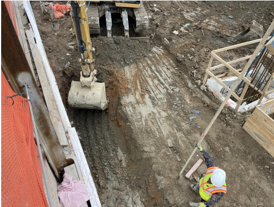
Photo 1: ECD excavating in WCG COMP J (facing south).
