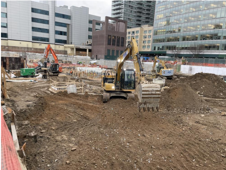
Photo 1: ECD grading in WCG COMP B (facing northeast).
