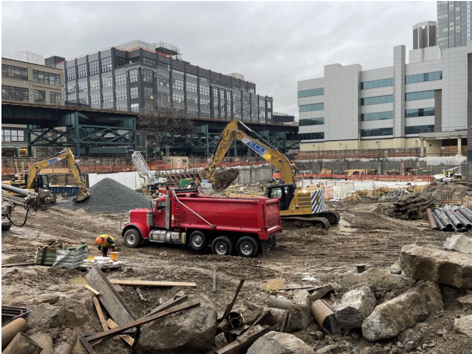
Photo 2: ECD loading non-hazardous soil/fill into trucks for offsite disposal (facing northwest).
