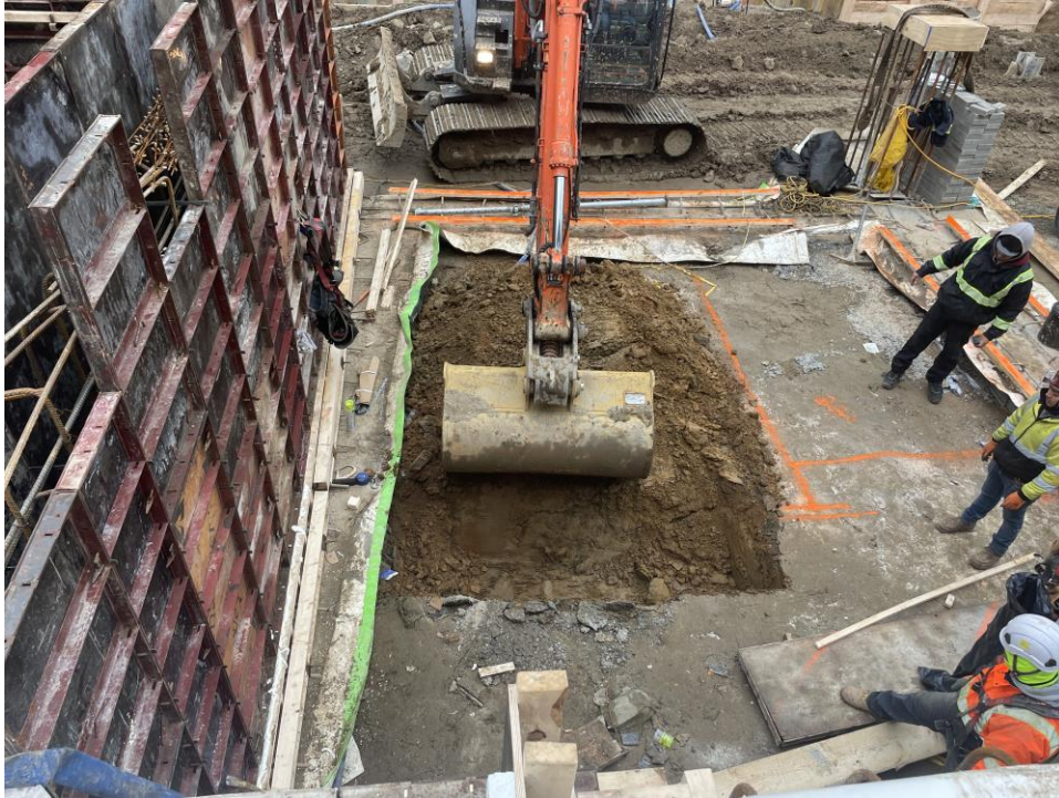
Photo 1: ECD excavating in WCG COMP L (facing east).
