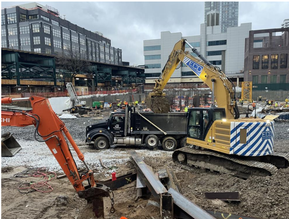
Photo 2: ECD loading a truck with fill/soil for export off-site (facing northwest).
