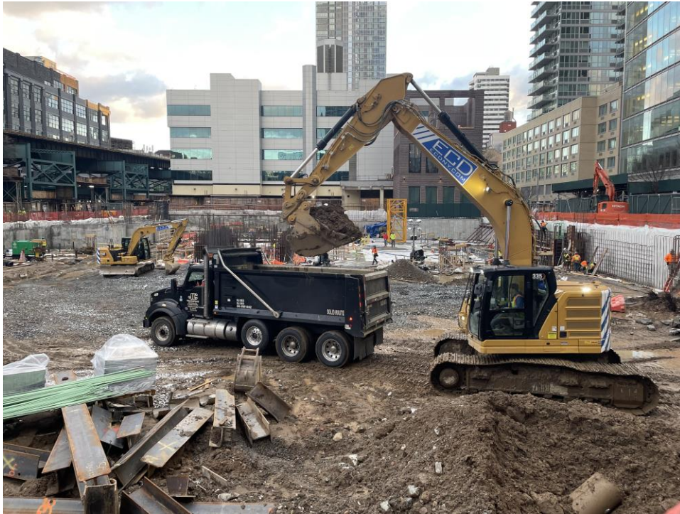
Photo 1: ECD loading a truck with fill/soil for export off-site (facing north).
