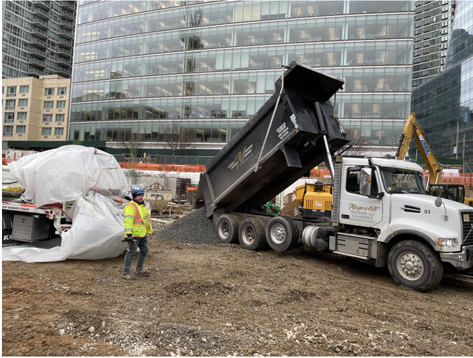
Photo 3: ECD importing ASTM #57 stone in the central part of the site (WCG F, facing east).
