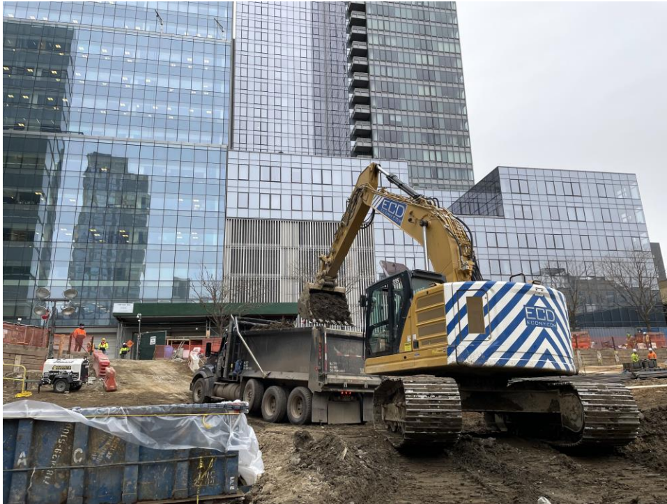
Photo 3: Loading a truck with fill/soil for export off-site (facing south).
