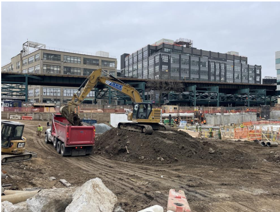
Photo 2: ECD loading trucks with previously stockpiled soil for off-site export (facing northwest).
