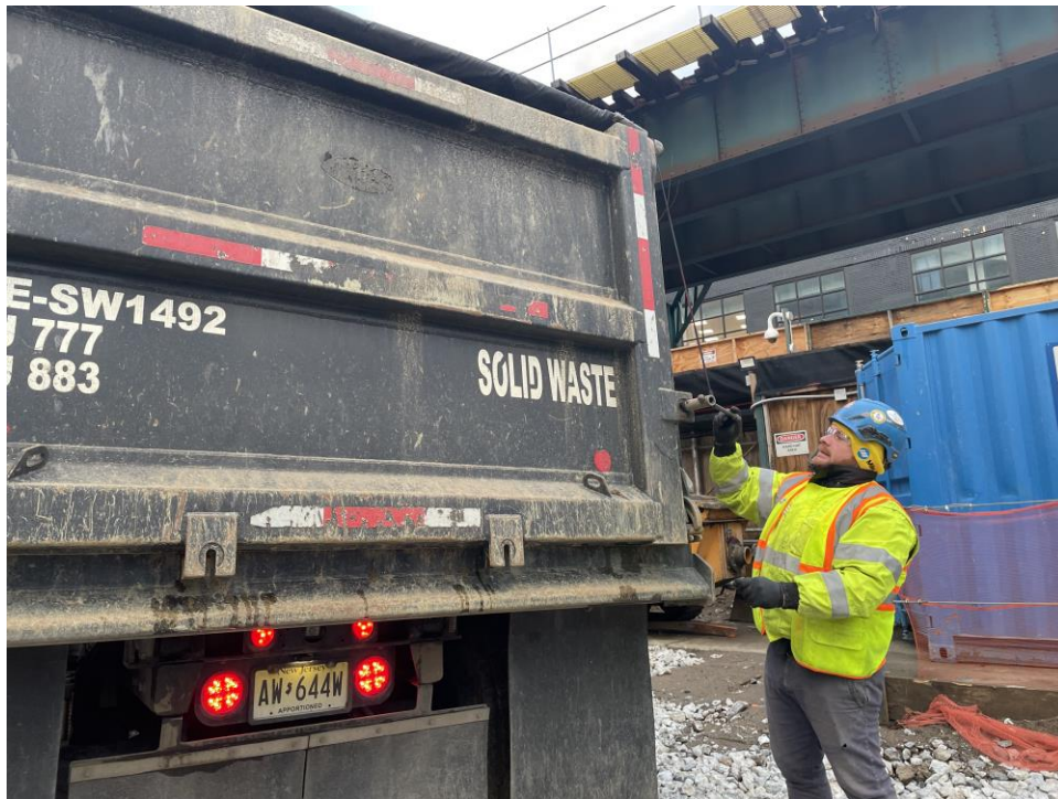
Photo 4: Securing truck cover with bungee cords for export off-site (facing southwest).
