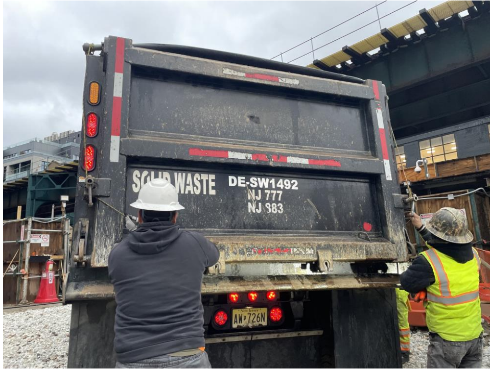
Photo 3: ECD securing truck cover with bungee cords for export off-site (facing southwest).
