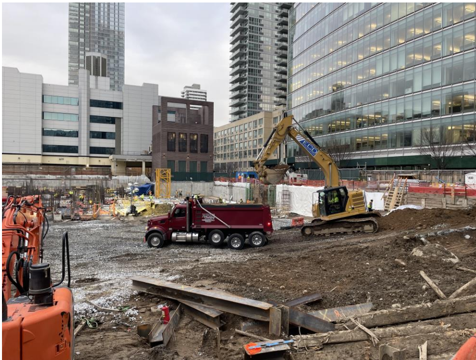
Photo 2: ECD loading a truck with fill/soil for export off-site (facing northeast).
