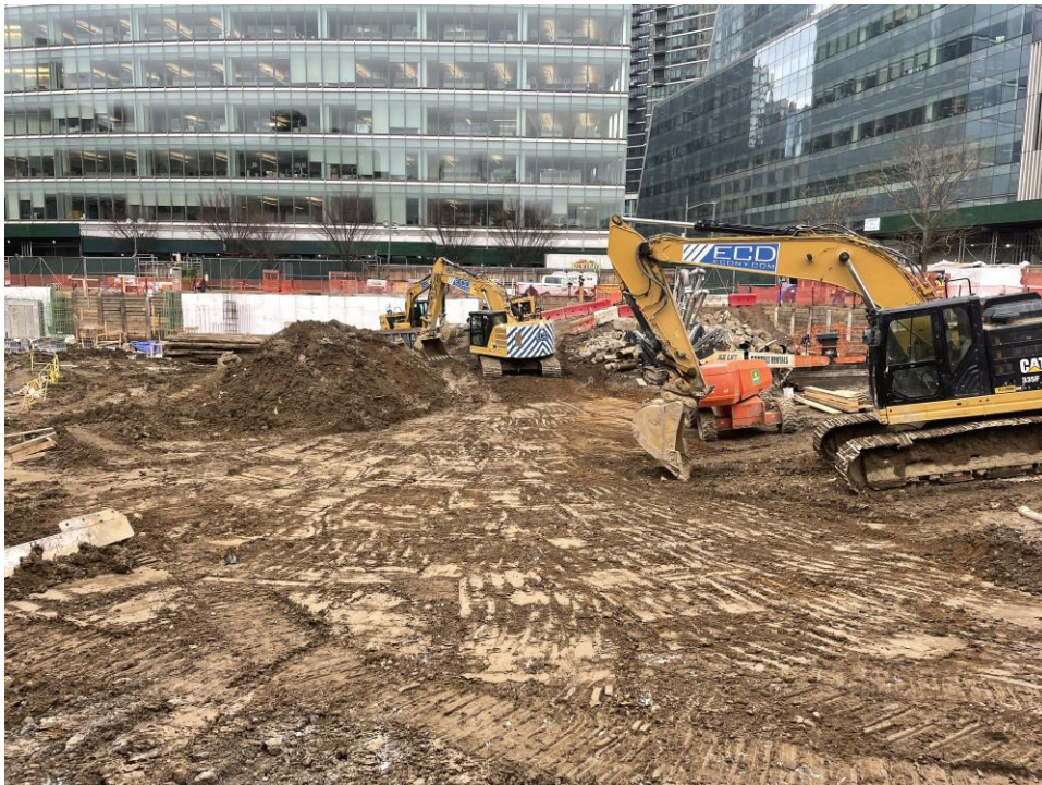
Photo 4: ECD grading in WCGs COMP B and C (facing east).
