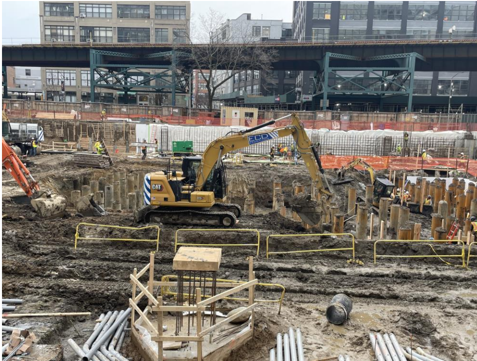
Photo 1: ECD excavating in the central part of the site (facing west).
