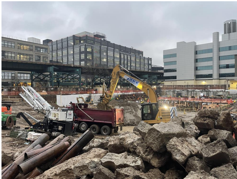
Photo 2: ECD loading previously stockpiled concrete for off-site export (facing northwest).
