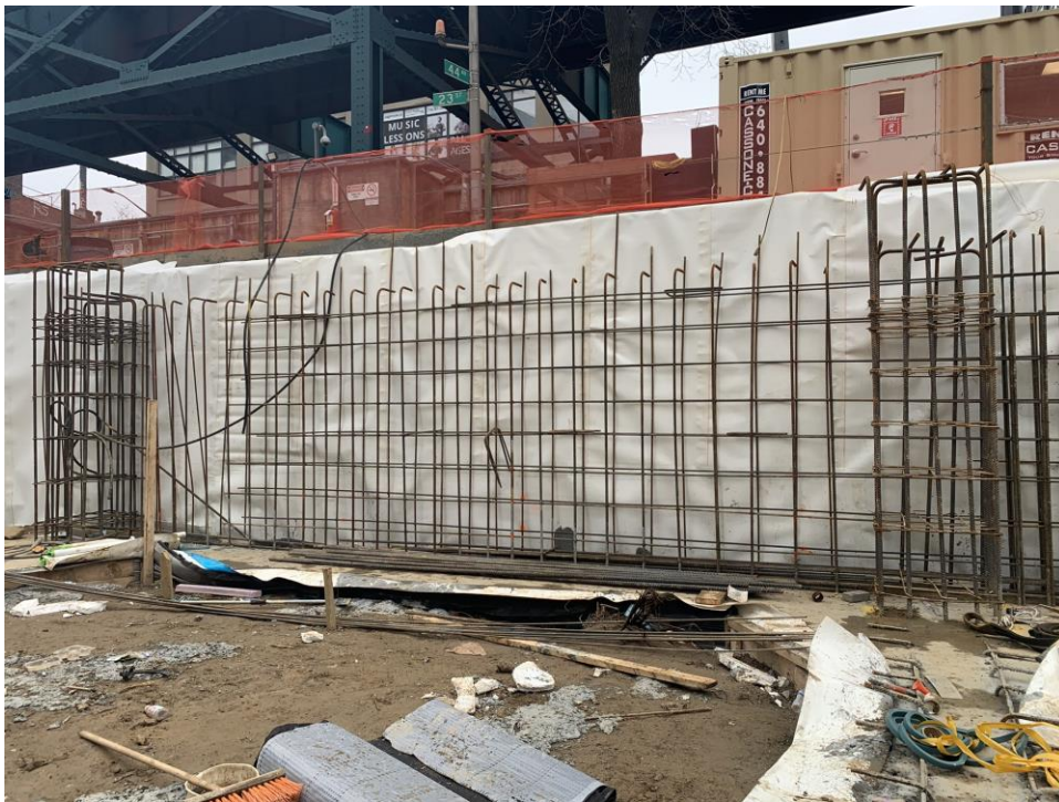
Photo 2: ECD installing waterproofing in WCG COMP B (facing west).
