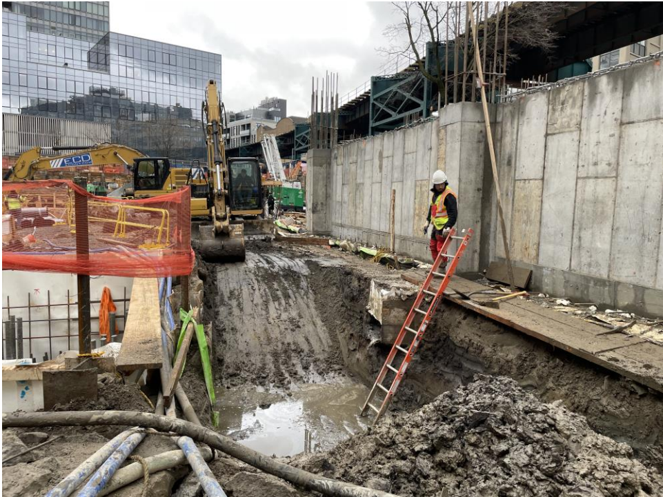
Photo 1: ECD excavating on the western side of the site (facing southwest).
