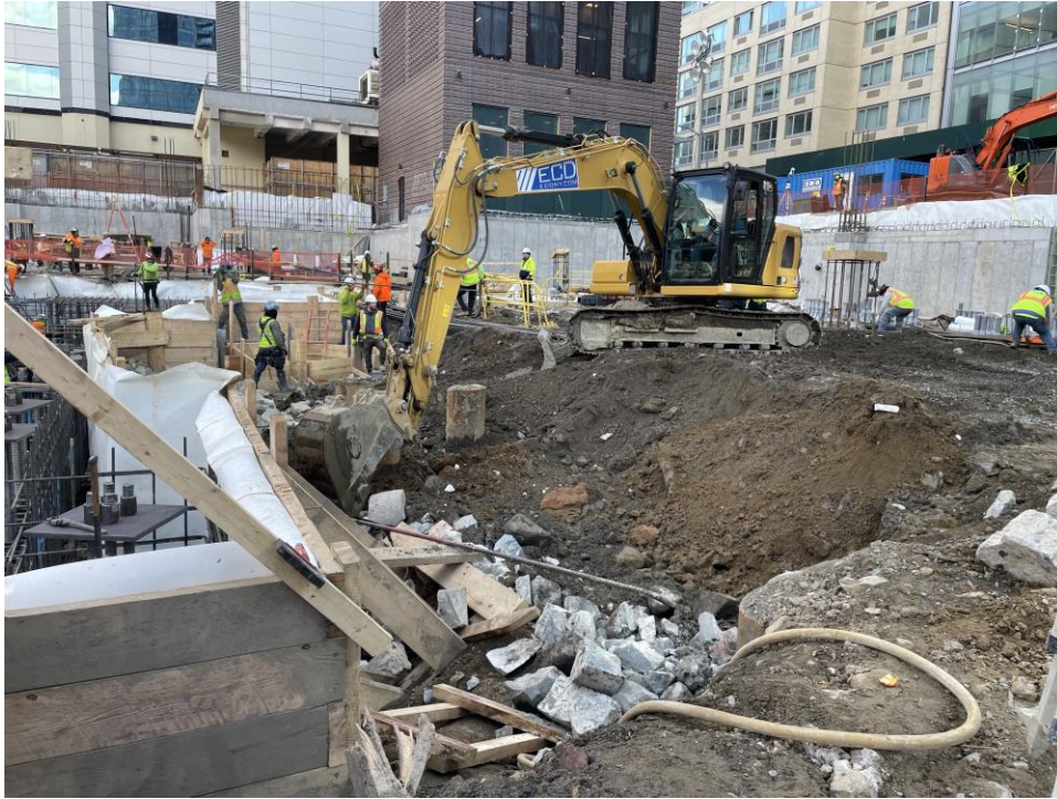
Photo 1: ECD excavating in the northeast part of the site (facing northeast).
