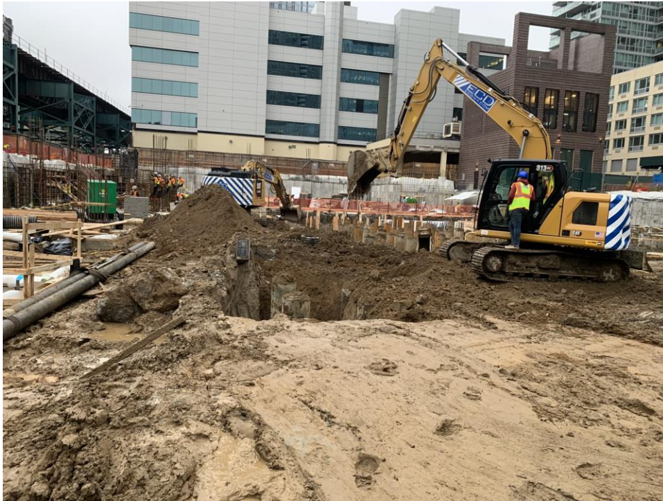
Photo 1: ECD excavating in WCG COMP F (facing north).
