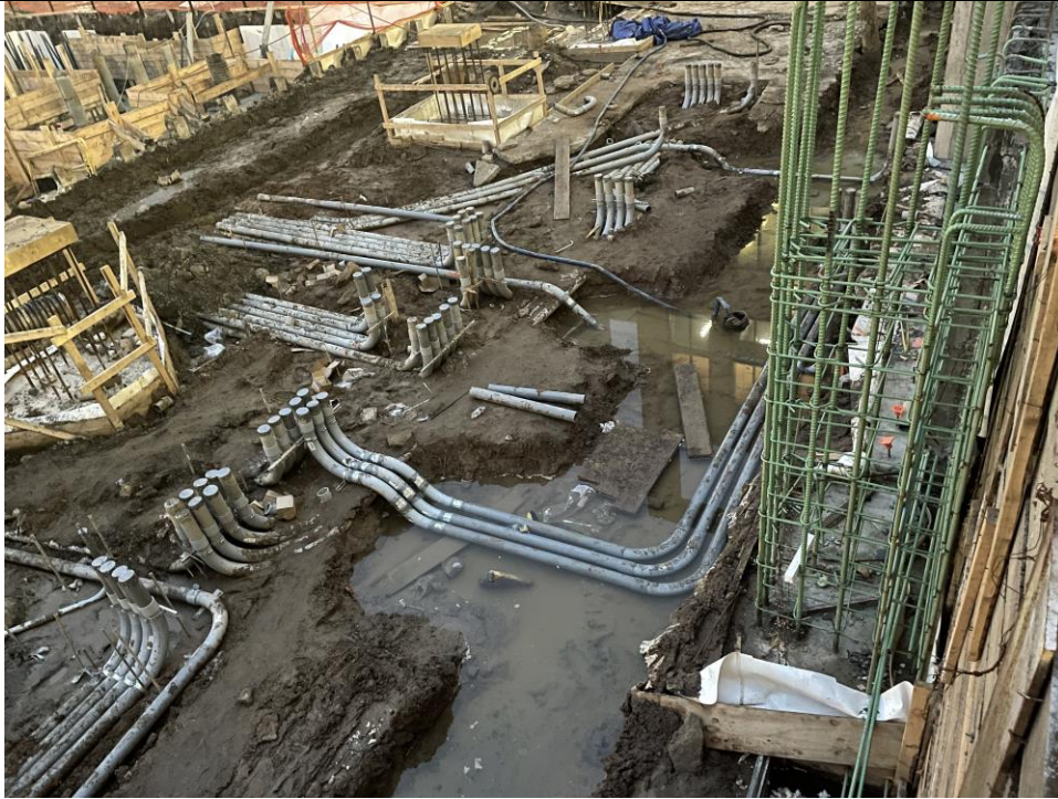
Photo 3: Utility excavation in WCG COMP L (facing north).
