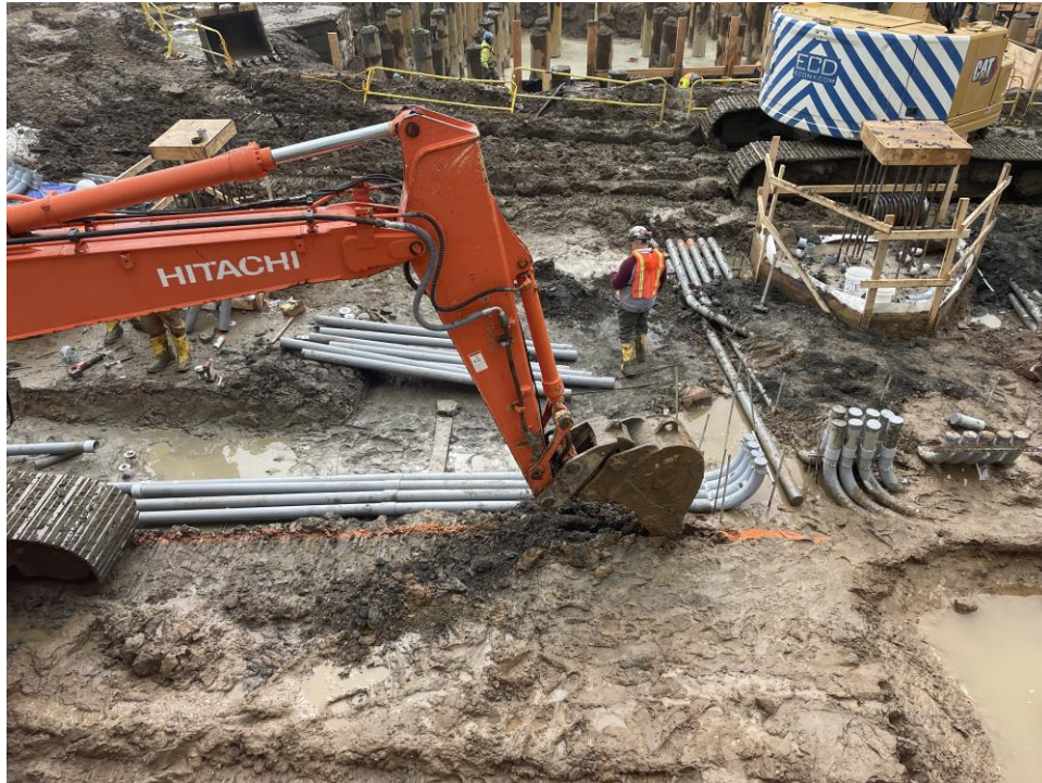
Photo 1: ECD excavating for piping installation in WCG COMP K (facing west).
