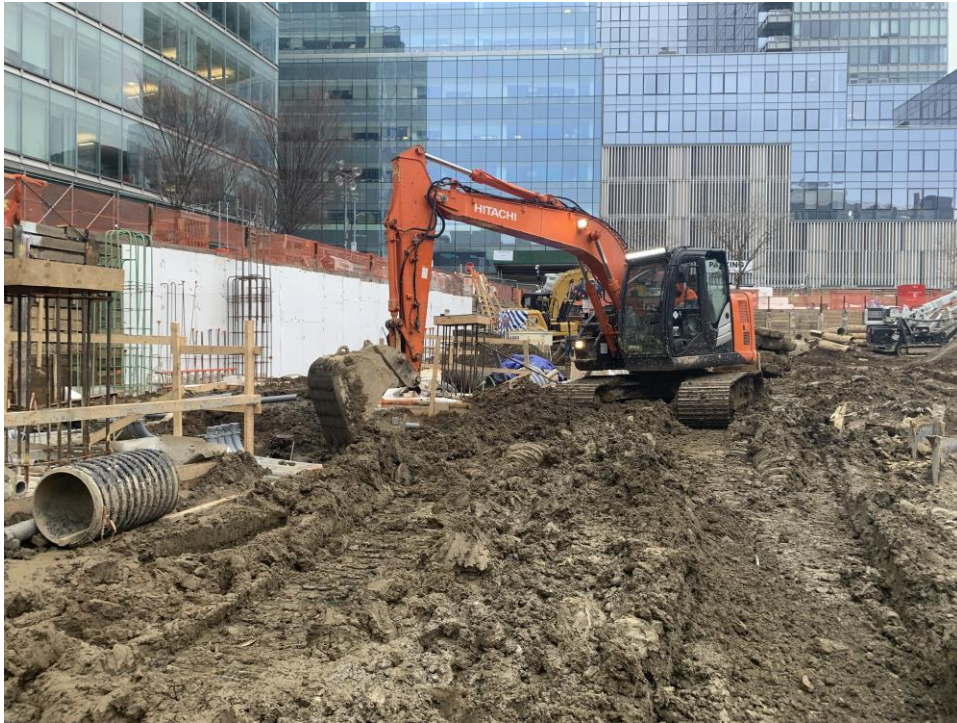
Photo 1: ECD excavating in WCG COMP K (facing south).
