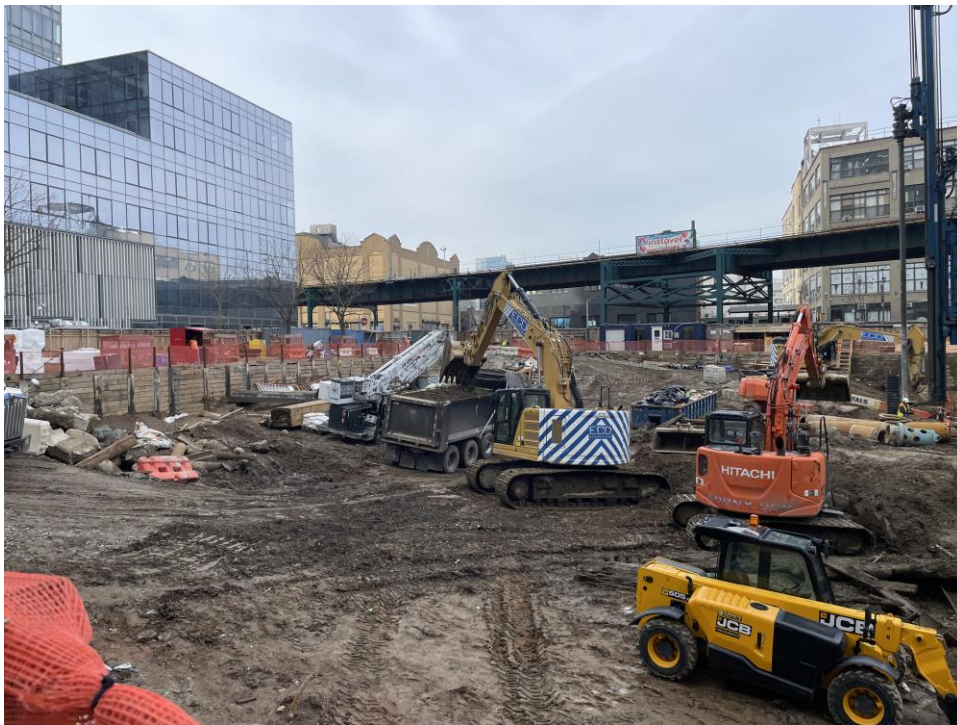
Photo 2: ECD loading non-hazardous soil/fill into trucks for offsite disposal (facing west).
