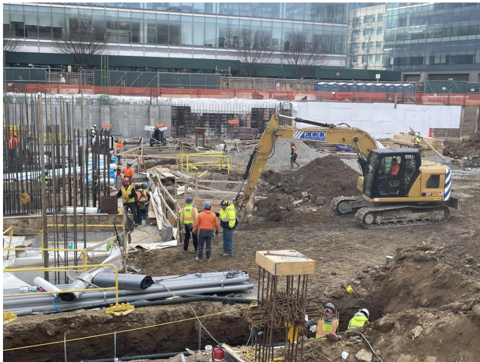
Photo 2: ECD excavating for pile cap formwork installation in the central part of the site (facing east).
