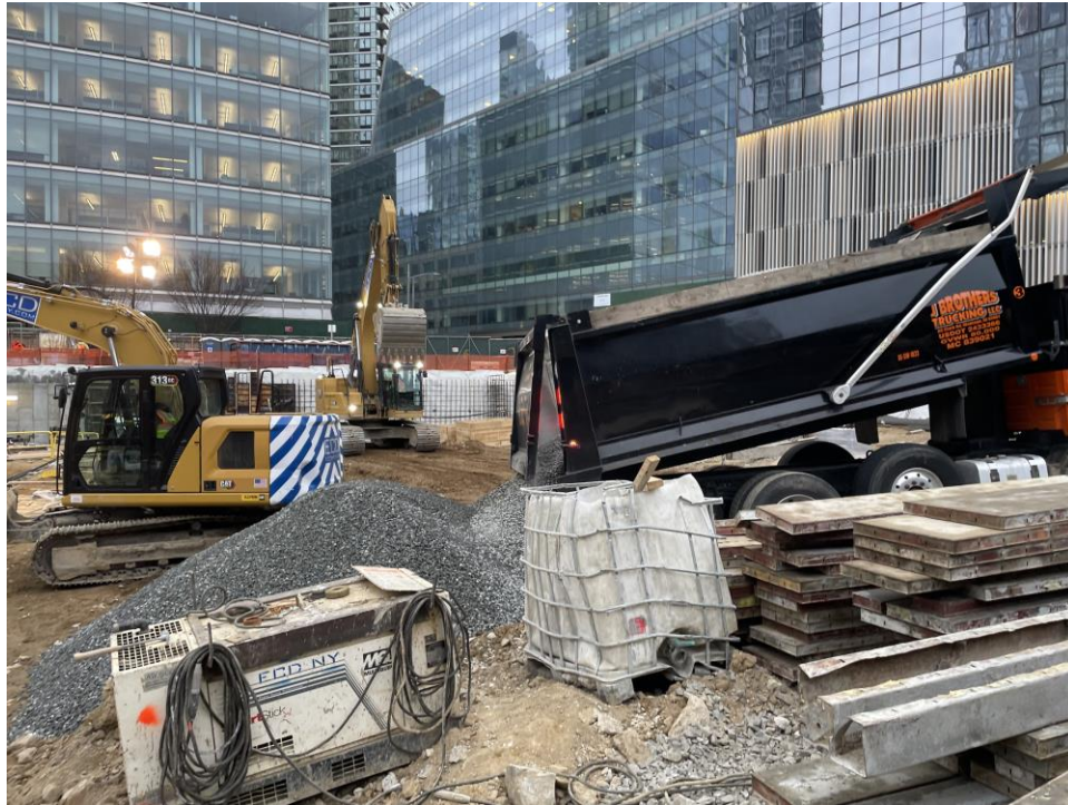
Photo 2: ECD importing 0.75-inch in the southern part of the site (facing southeast).
