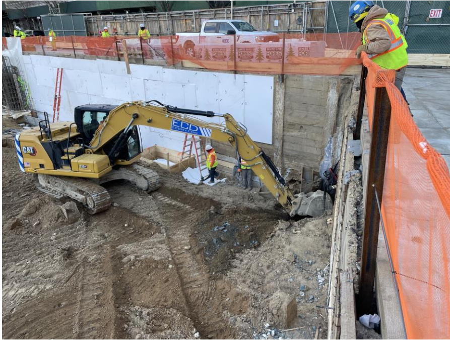
Photo 1: ECD excavating for SOE lagging in the southeastern part of the site (facing southeast).
