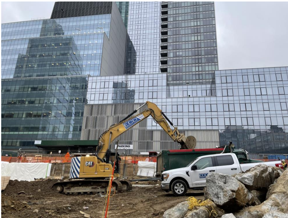
Photo 2: ECD loading a truck for off-site disposal in the southern part of the site (facing south).
