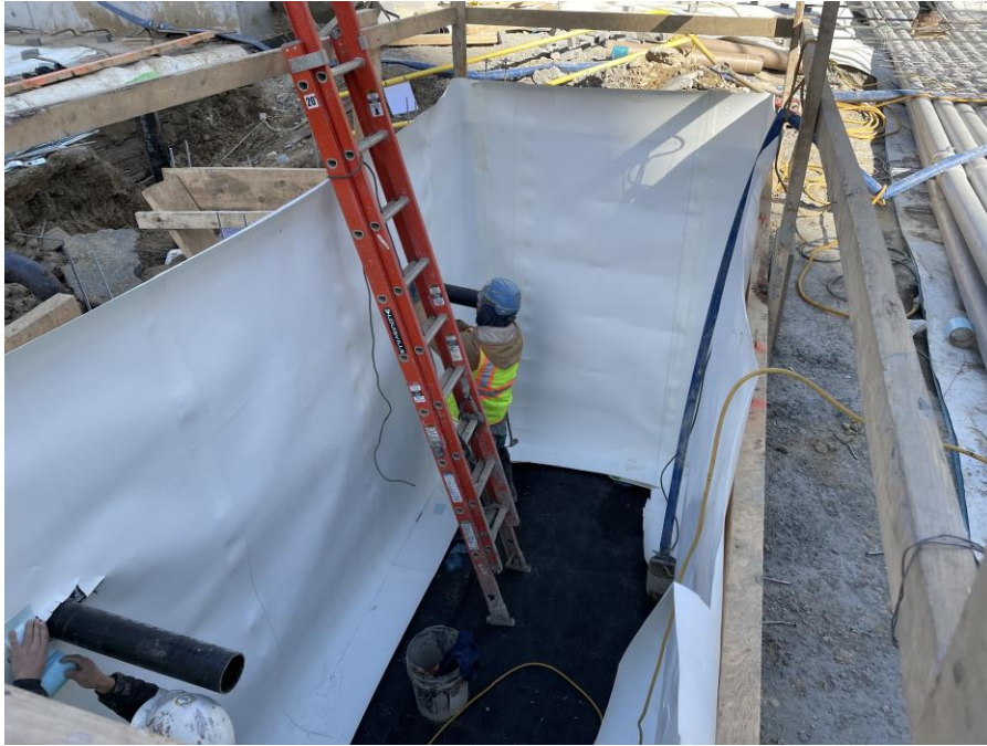
Photo 3: ECD installing Preprufe Vapor Barrier in the northern part of the trench in the northwestern part of the site (facing down).
