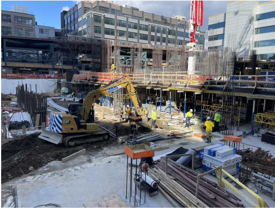
Photo 1: ECD backfilling with previously excavated material in the central part of the site (WCG F, facing northwest).
