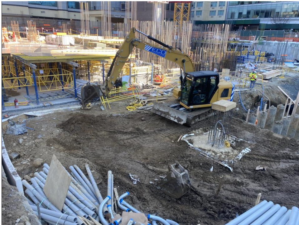
Photo 2: ECD stockpiling non-hazardous material from COMP B (12-15') in the western part of the site (facing northeast).
