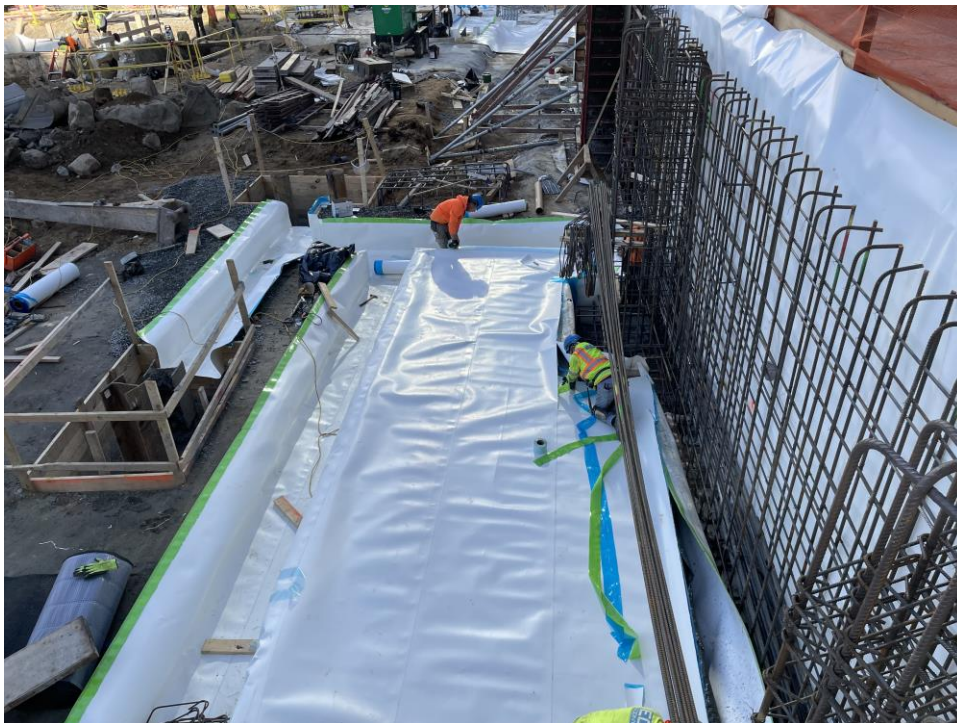
Photo 2: ECD installing waterproofing in the southeastern part of the site (WCG I, facing north).
