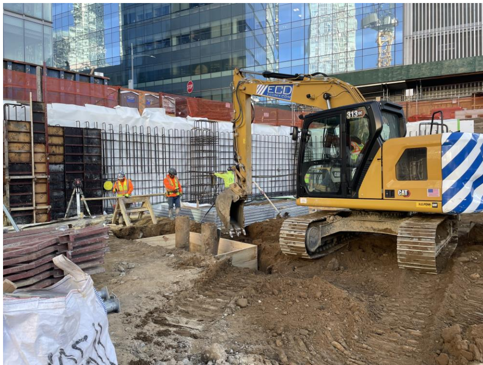
Photo 2: ECD backfilling around the pile cap formwork with previously excavated material from this location in the southeastern part of the site (WCG I, facing southeast).
