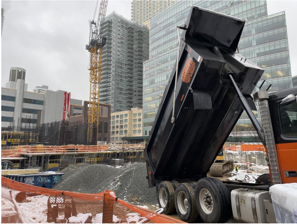
Photo 3: ECD importing 0.75-inch in the southern part of the site (facing northeast).
