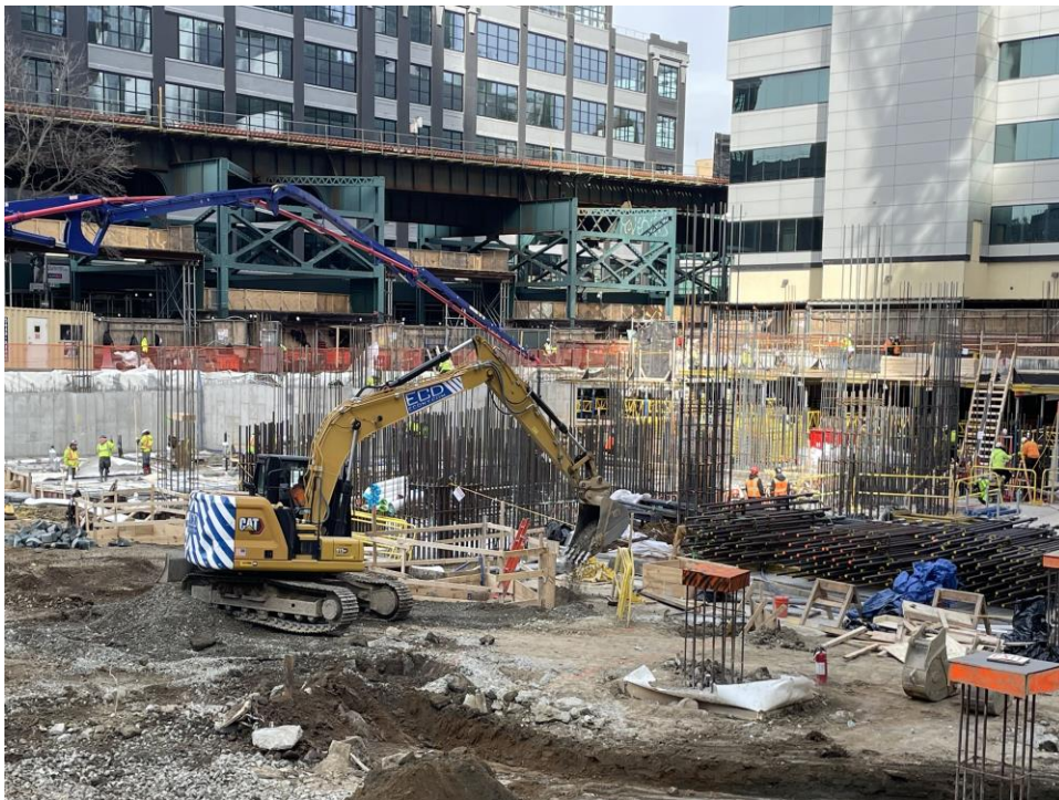
Photo 4: ECD backfilling around a pile cap with stone in the central part of the site (facing northwest).
