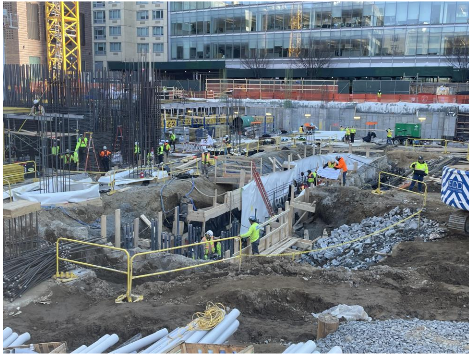
Photo 3: ECD installing waterproofing in the central part of the site (facing east).
