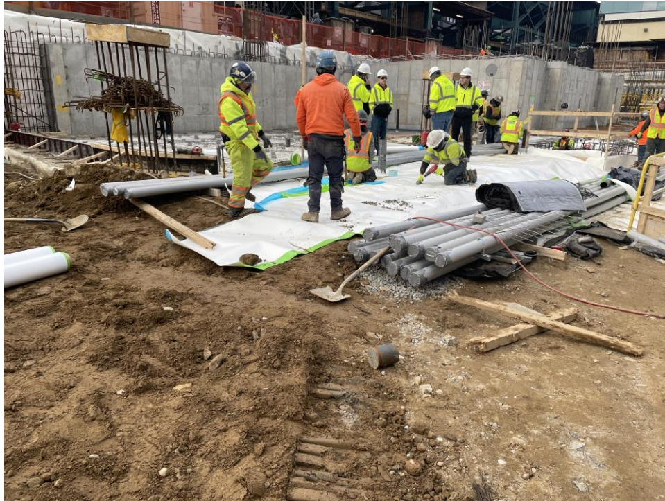
Photo 1 ECD installing waterproofing in the northwestern part of the site (facing northwest).
