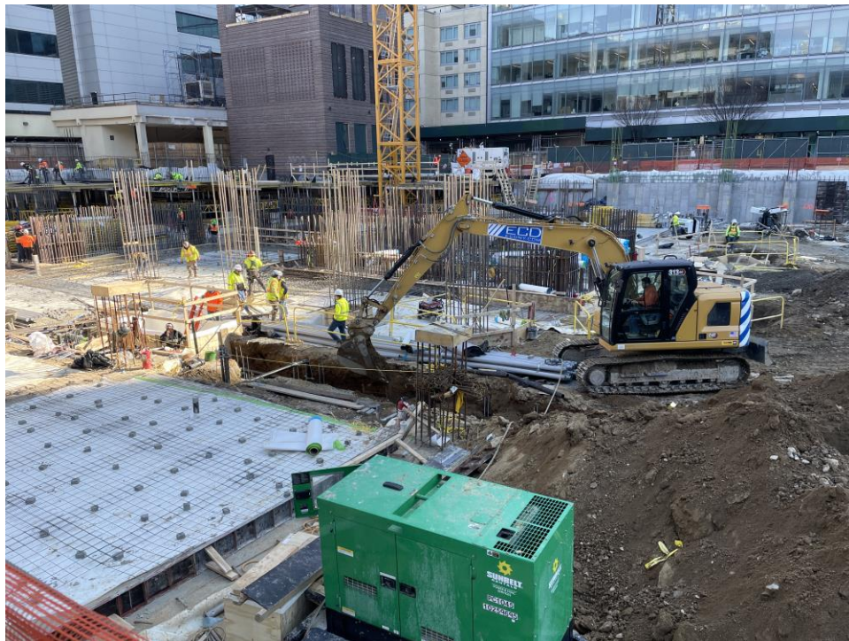
Photo 4: ECD backfilling the utility trench in the north-central part of the site (facing northeast).
