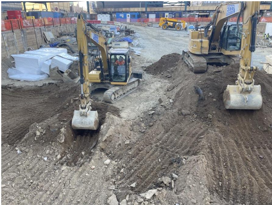
Photo 2: ECD excavating for pile cap formwork installation in the central part of the site (facing southwest).
