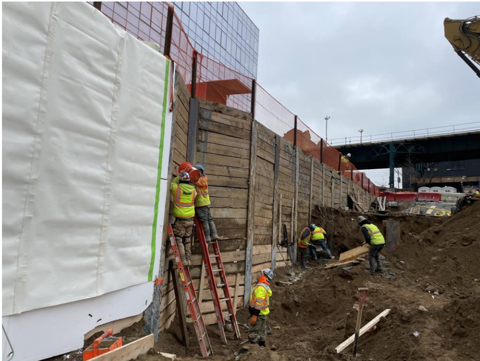
Photo 2: ECD installing waterproofing and SOE lagging in the southeastern part of the site (facing west).
