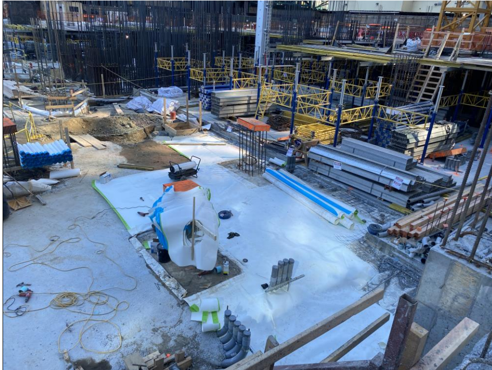
Photo 3: ECD installing waterproofing in the eastern part of the site (facing northwest).
