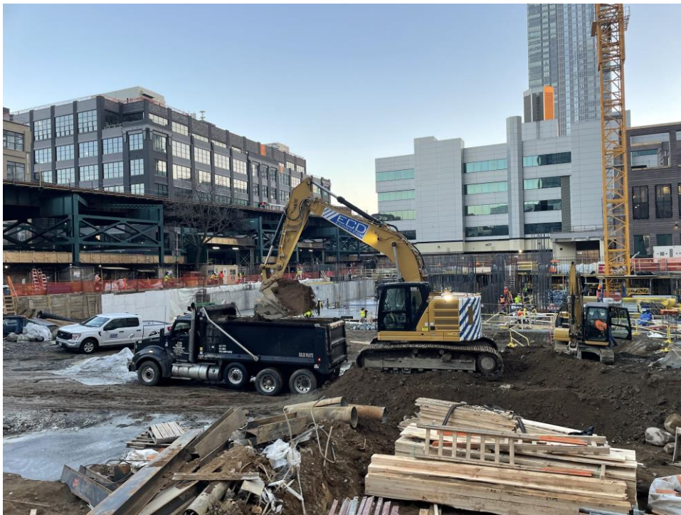
Photo 2: ECD loading a truck for off-site disposal in the central part of the site (facing north).
