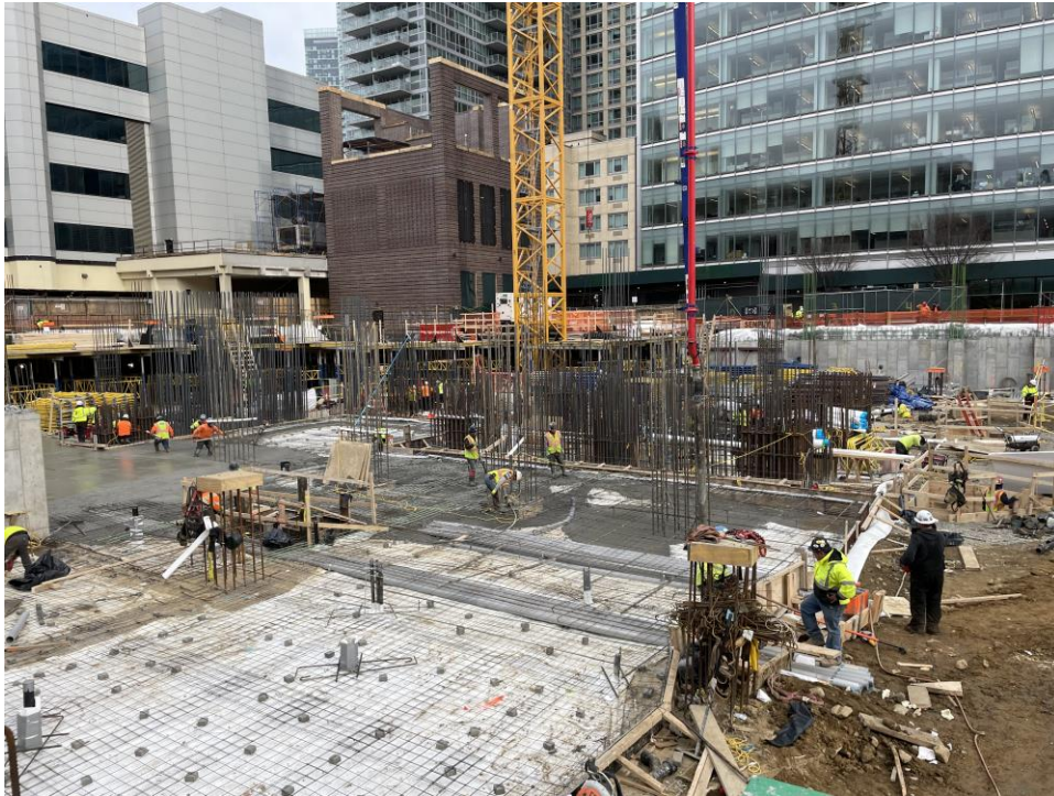
Photo 3: ECD pouring concrete for foundation slab in the western part of the site (facing northeast).
