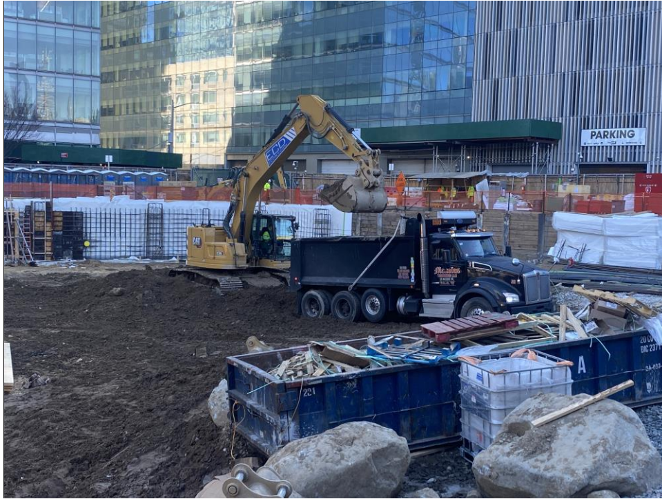
Photo 1 ECD loading trucks with non-hazardous fill from the stockpile in the southeastern part of the site (facing southeast)
