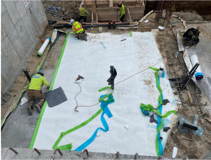
Photo 3: ECD installing Preprufe Vapor Barrier atop the mud slab in the northwestern part of the site (facing down).
