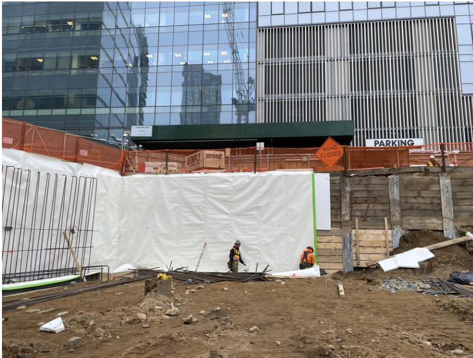
Photo 4: ECD installing waterproofing in the southern part of the site (WCG I, facing south).
