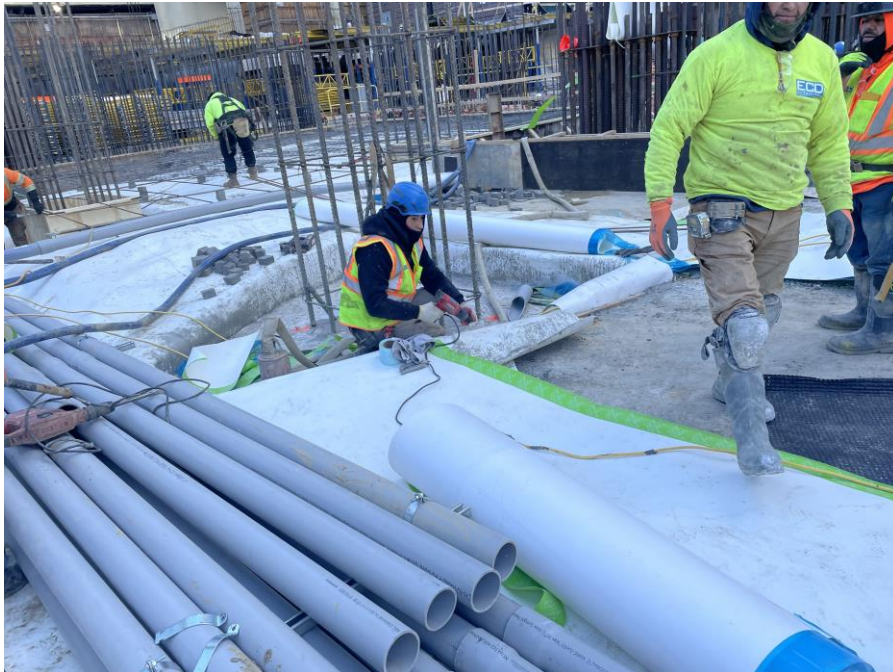
Photo 4: ECD installing Preprufe Vapor Barrier atop the mud slab in the central part of the site (facing north).
