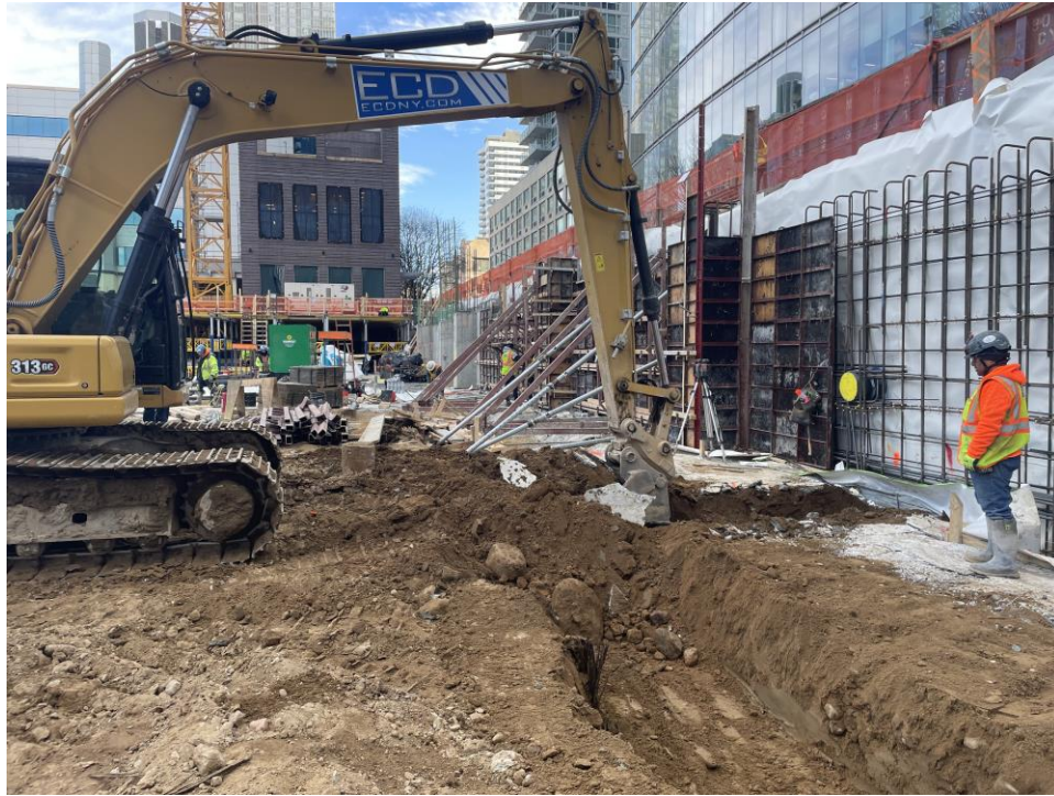
Photo 1: ECD excavating for utility trenches in the southeastern part of the site (WCG I, facing north).
