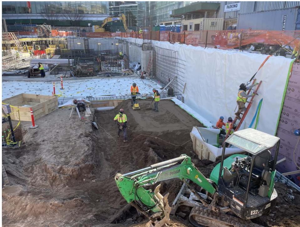
Photo 4: ECD compacting material and installing waterproofing in WCG COMP A (facing southeast).
