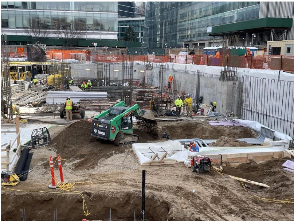
Photo 2: ECD backfilling with previously-imported 0.75-inch quarry stone in the southern part of the site (facing east).
