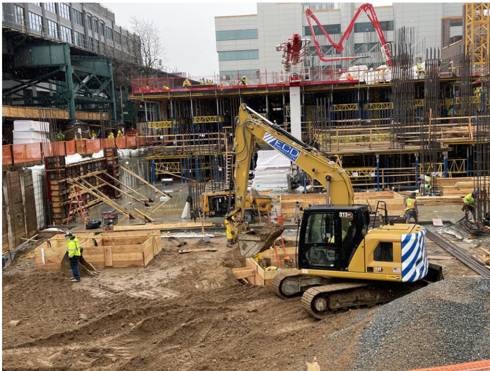
Photo 2: ECD backfilling with previously excavated material that had been temporarily stockpiled adjacent to the area in the southwestern part of the site (facing north).
