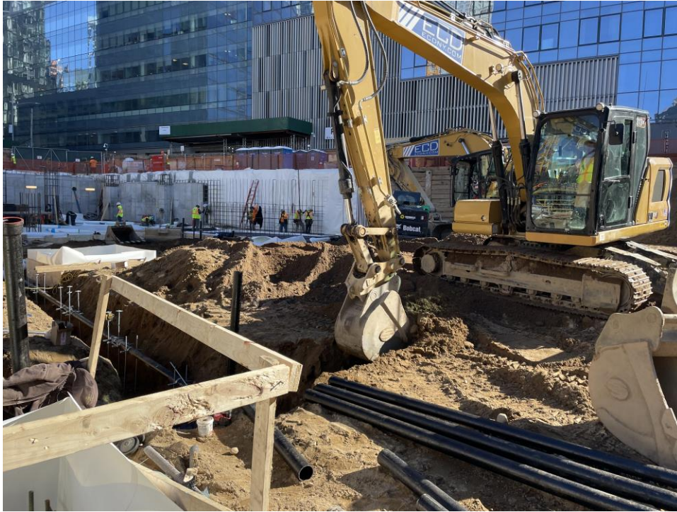
Photo 1: ECD excavating a utility trench in the southwestern part of the site (facing south).
