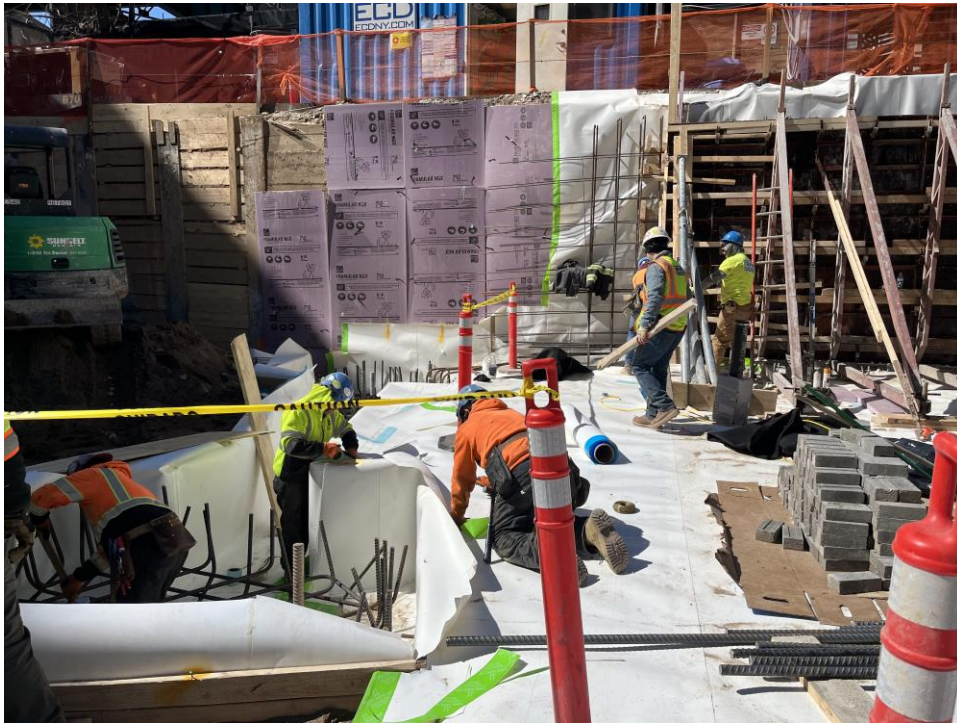
Photo 4: ECD installing waterproofing and formwork in WCG COMP A (facing west).
