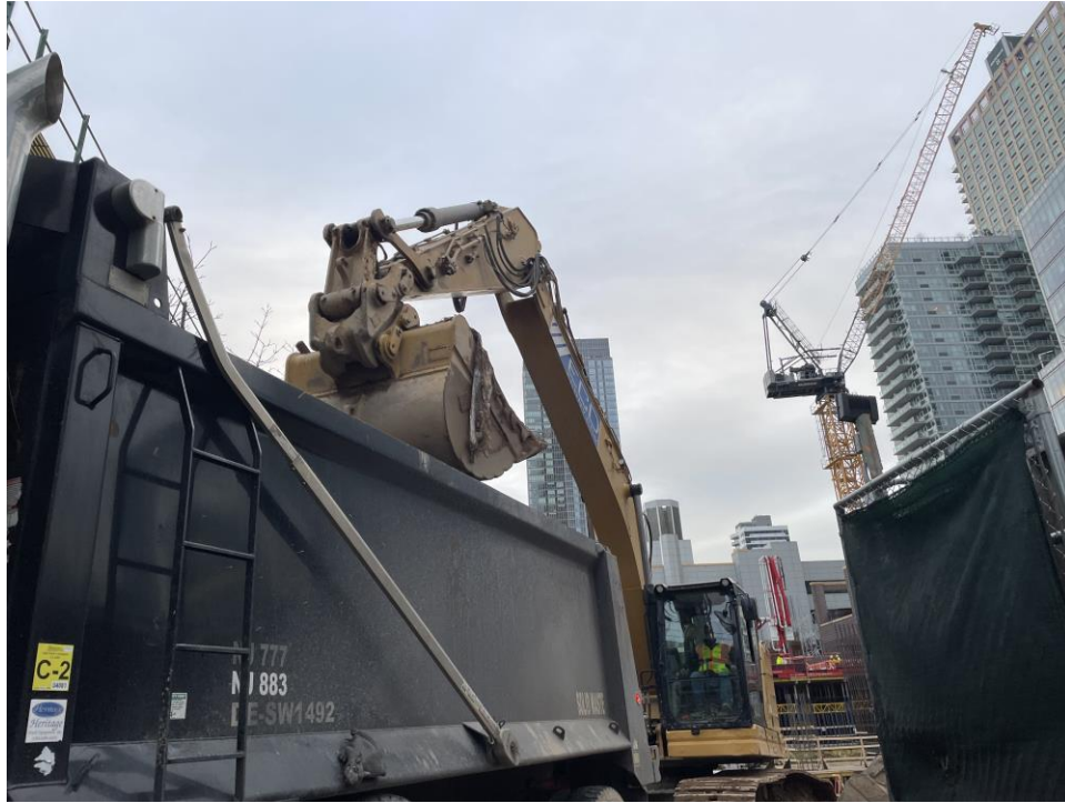
Photo 3: ECD loading a truck for off-site disposal in the southwestern part of the site (facing north).
