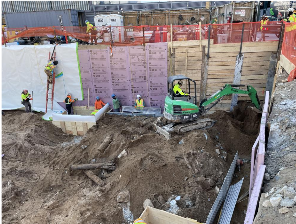
Photo 3: ECD excavating for lagging installation in WCG COMP A (facing south).
