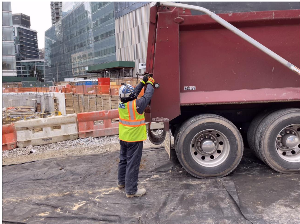
Photo 4: ECD securing a truck cover for off-site disposal (facing southeast).
