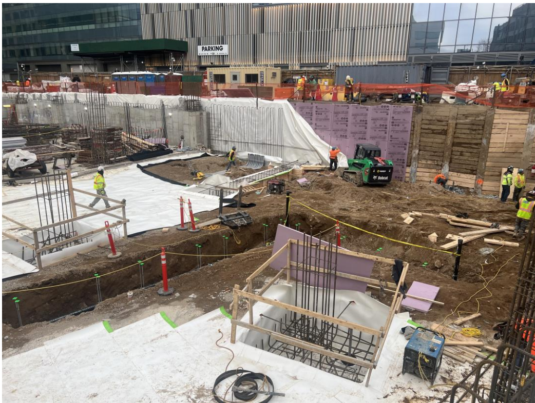
Photo 2: ECD installing waterproofing in WCG COMP A (facing south).
