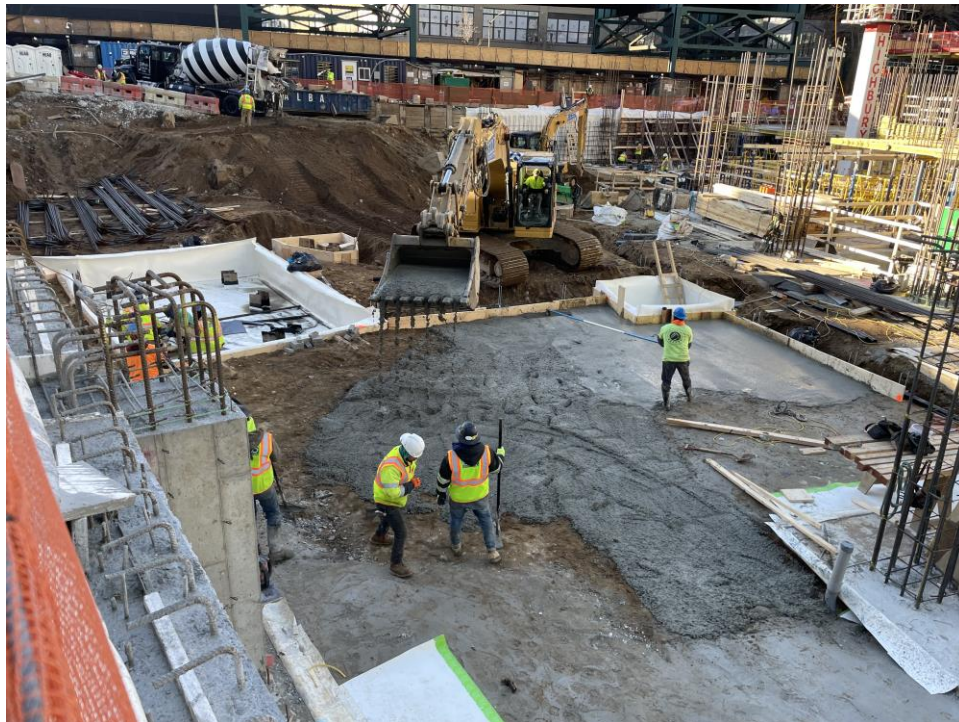
Photo 4: ECD pouring concrete for mat slab in the southern part of the site (WCG I, facing west).
