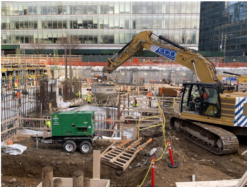
Photo 4: ECD pouring concrete for foundation elements in the central part of the site (facing east).
