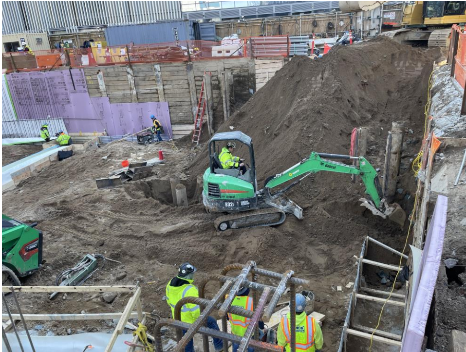
Photo 1: ECD excavating for SOE lagging installation in the southwestern part of the site (facing south).
