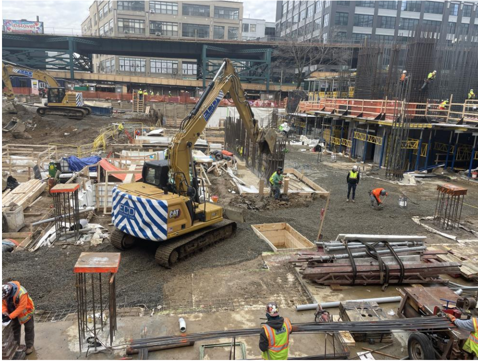
Photo 3: ECD excavating around SOE soldier piles in the central part of the site (WCG J, facing northeast).
