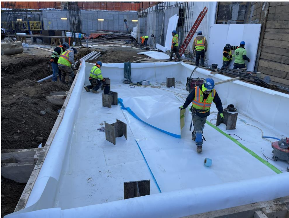
Photo 2: ECD installing waterproofing in the southern part of the site (WCG A, facing east).
