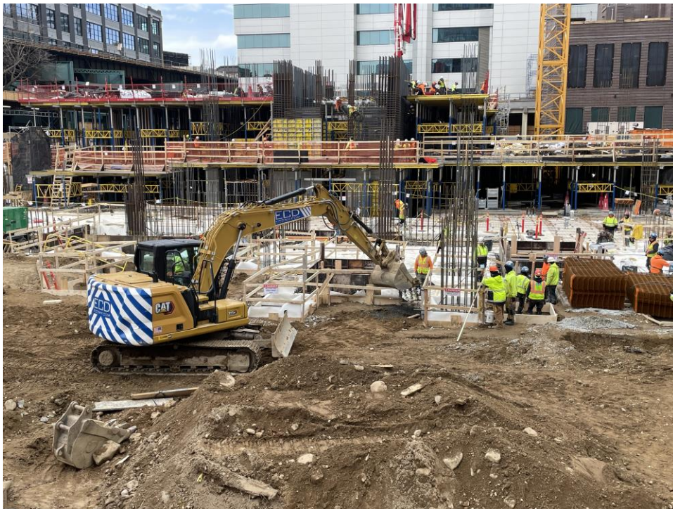
Photo 2: ECCO backfilling with 0.75-inch imported stone in the central part of the site (WCG F/E, facing north).
