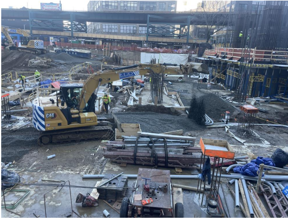
Photo 1: ECD backfilling with 0.75-inch stone for a utility trench in the southern part of the site (WCG J, facing northeast).
