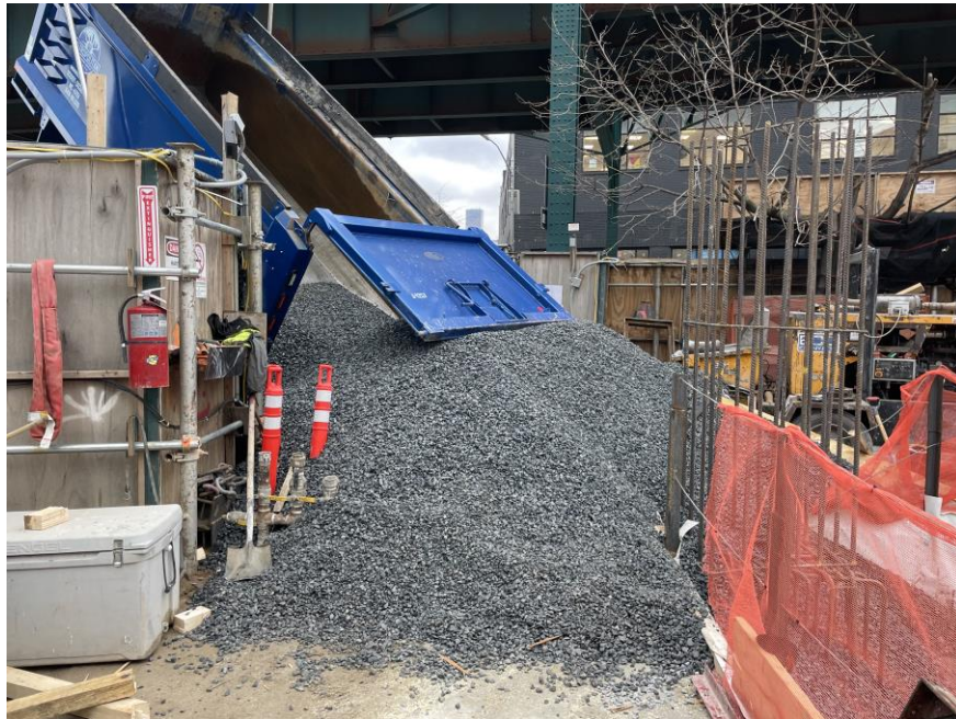
Photo 2: ECD stockpiling imported 0.75-inch stone in COMP A (facing northeast).
