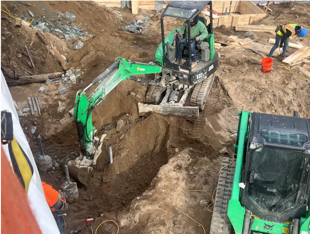
Photo 1: ECD excavating around a pile cap in WCG COMP A (facing west).
