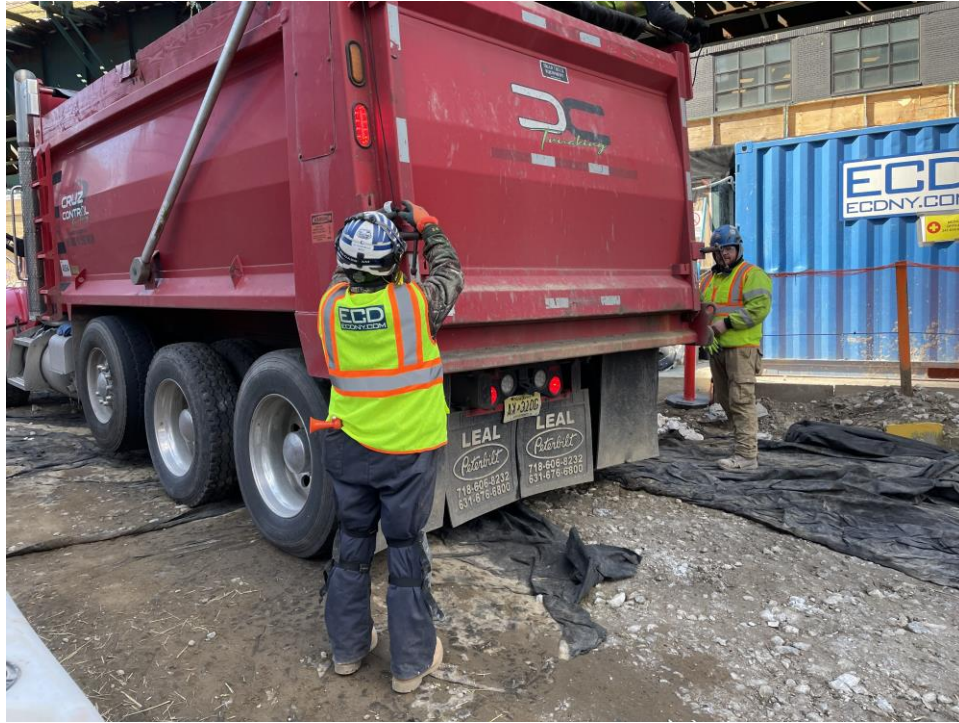
Photo 3: ECD securing a truck cover for offsite disposal (facing southwest).
