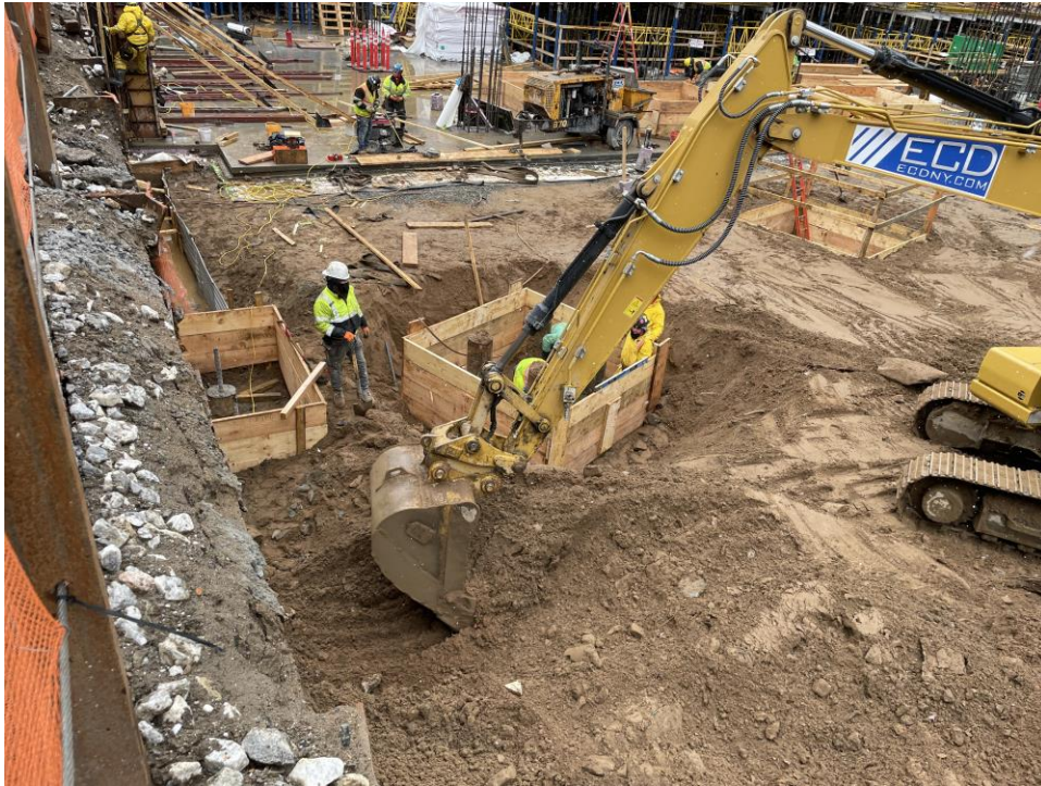
Photo 1: ECD excavating for SOE lagging installation in the southwestern part of the site (facing northeast).
