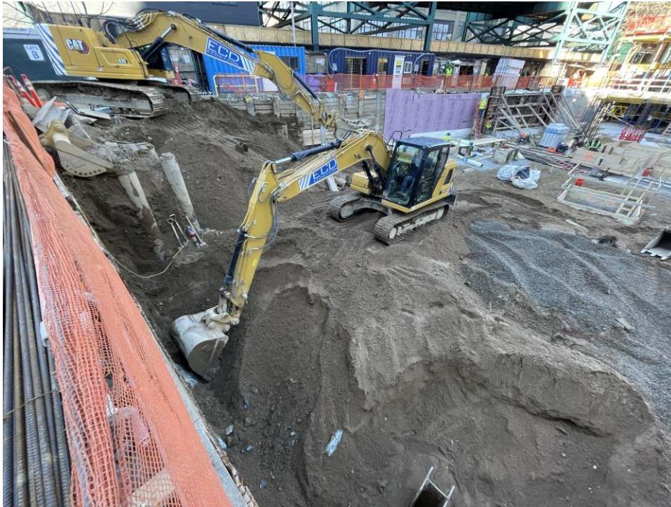
Photo 1: ECD excavating for SOE lagging installation in the southwestern part of the site (facing northwest).
