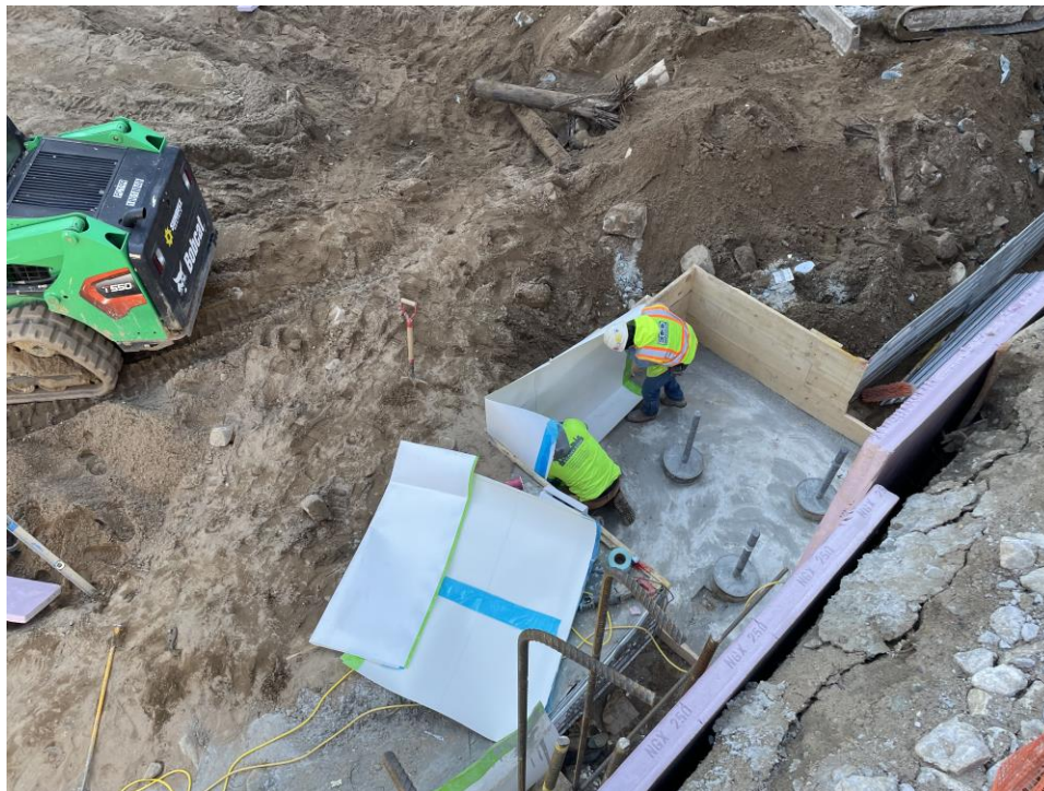
Photo 2: ECD installing waterproofing in WCG COMP A (facing northeast).
