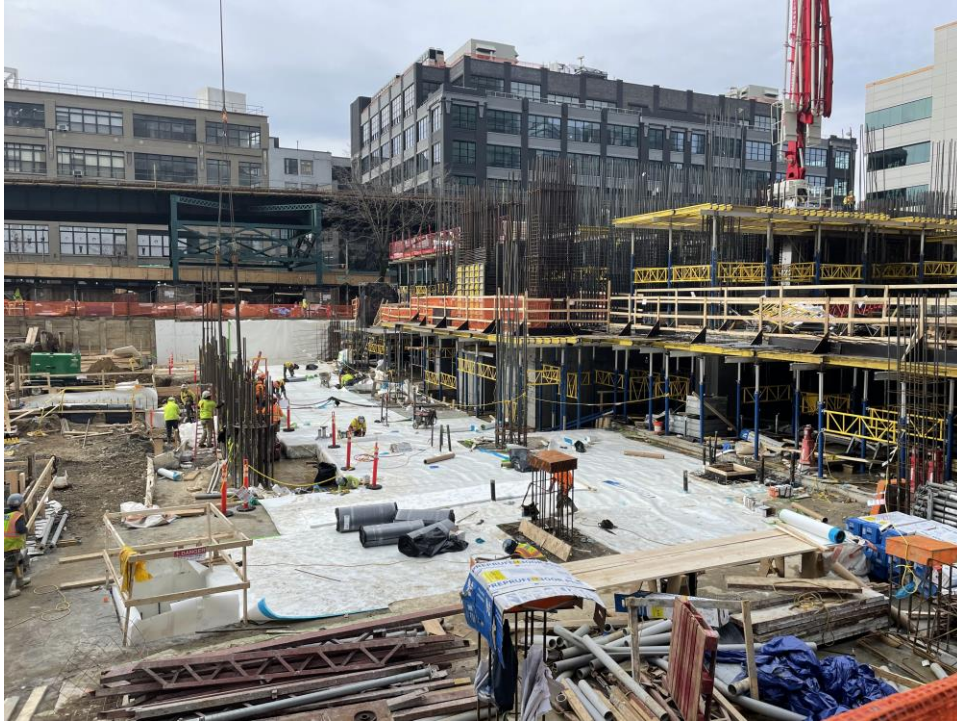
Photo 3: ECD installing waterproofing for foundation in the central part of the site (WCG B, J and F facing northwest).
