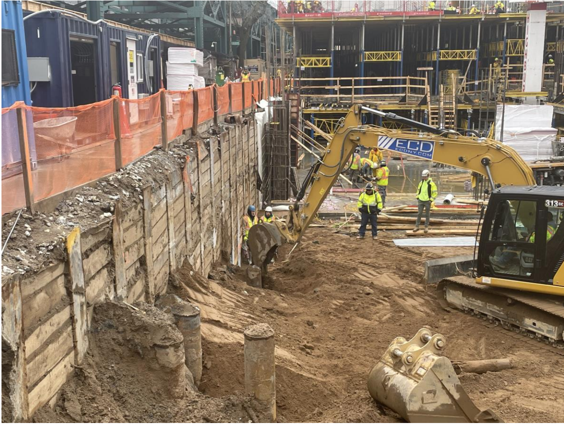
Photo 1: ECD excavating in the western part of the site and installing SOE lagging (facing north).
