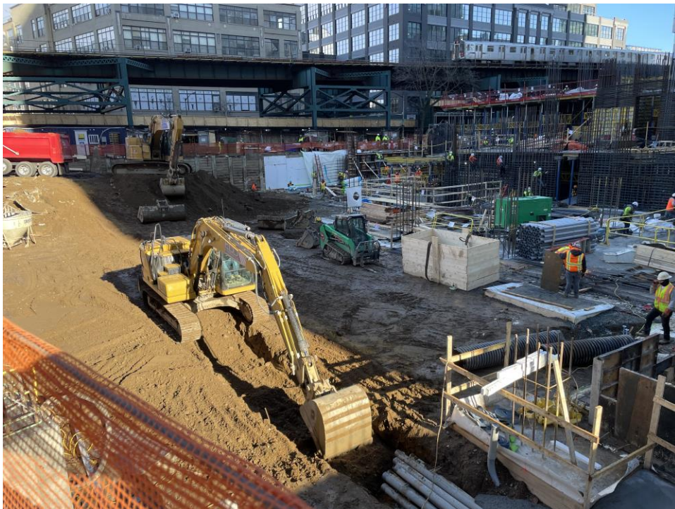
Photo 2: ECD excavating for a utility trench in the western part of the site (WCG I, facing west).
