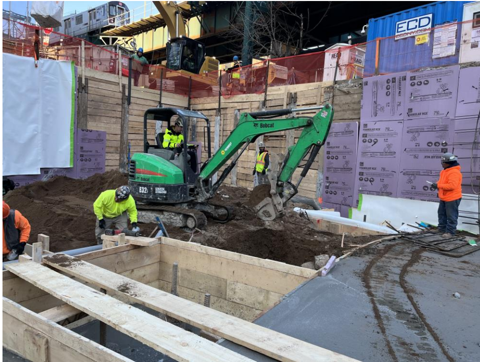
Photo 1: ECD excavating around a pile cap in WCG COMP A (facing southwest).
