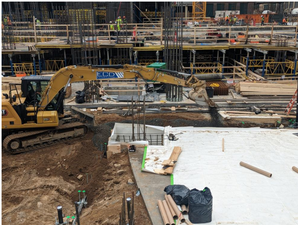
Photo 4: ECD backfilling 0.75-inch stone for waterproofing installation in the southern part of the site (WCG E, facing north).
