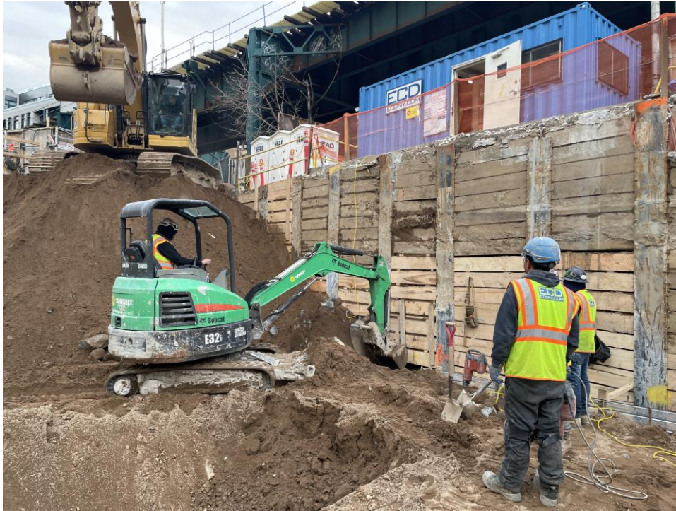
Photo 1: ECD excavating for SOE lagging installation in the southwestern part of the site (facing southwest).
