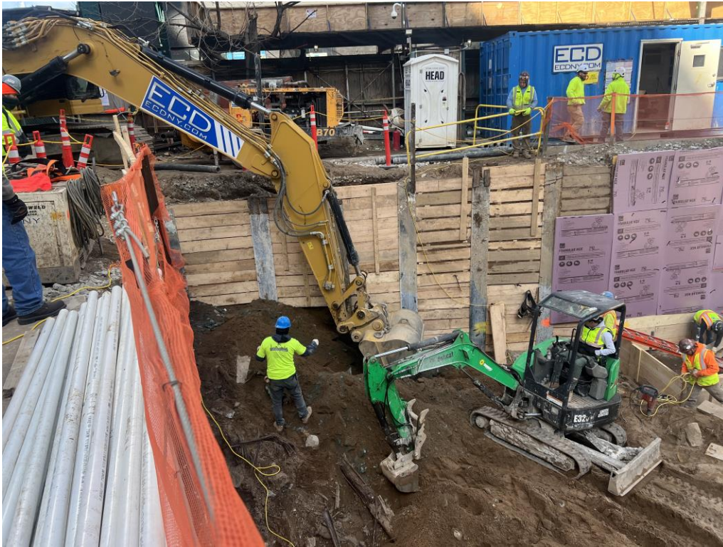
Photo 3: ECD excavating for lagging installation in WCG COMP A (facing west).
