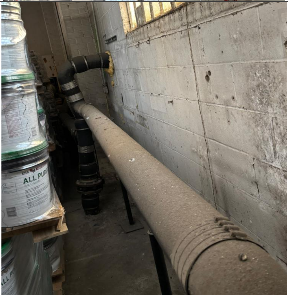
Photo 8 – View of SVE wells and riser pipe.
