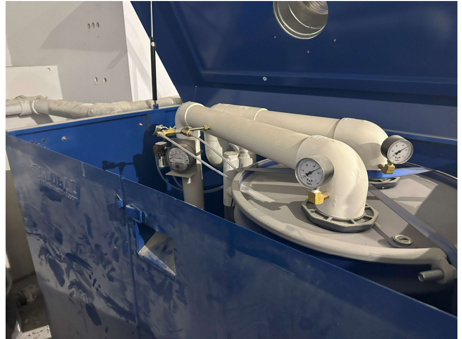
8- View of vacuum gauge at SSDS-1 blower
