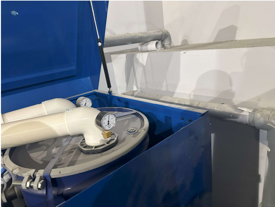
7- View of vacuum gauge at SSDS-2 blower
