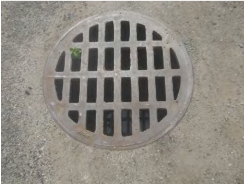
A storm drain at the property.
