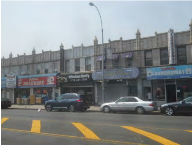
The property to the north.
