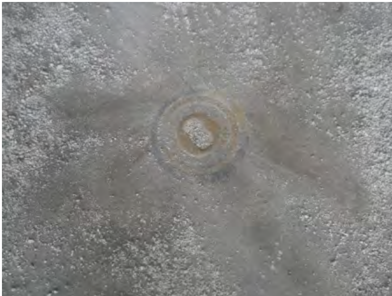
The fill pipe for the inactive underground storage tank.
