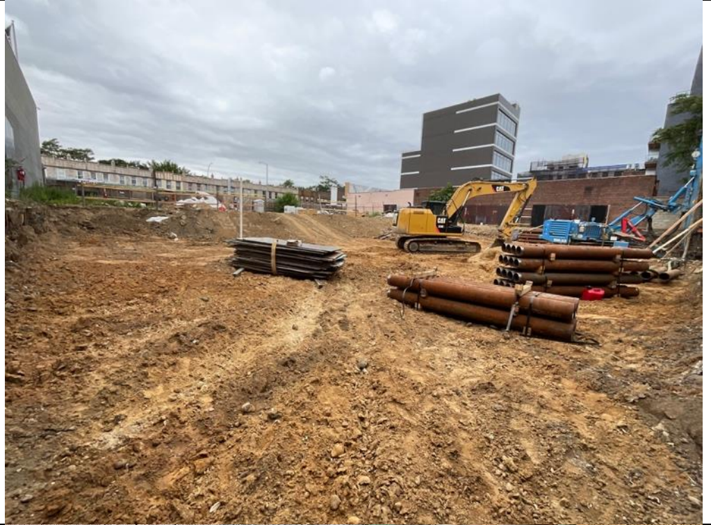
Photo 1 – An overview of the site at the end of working day.
