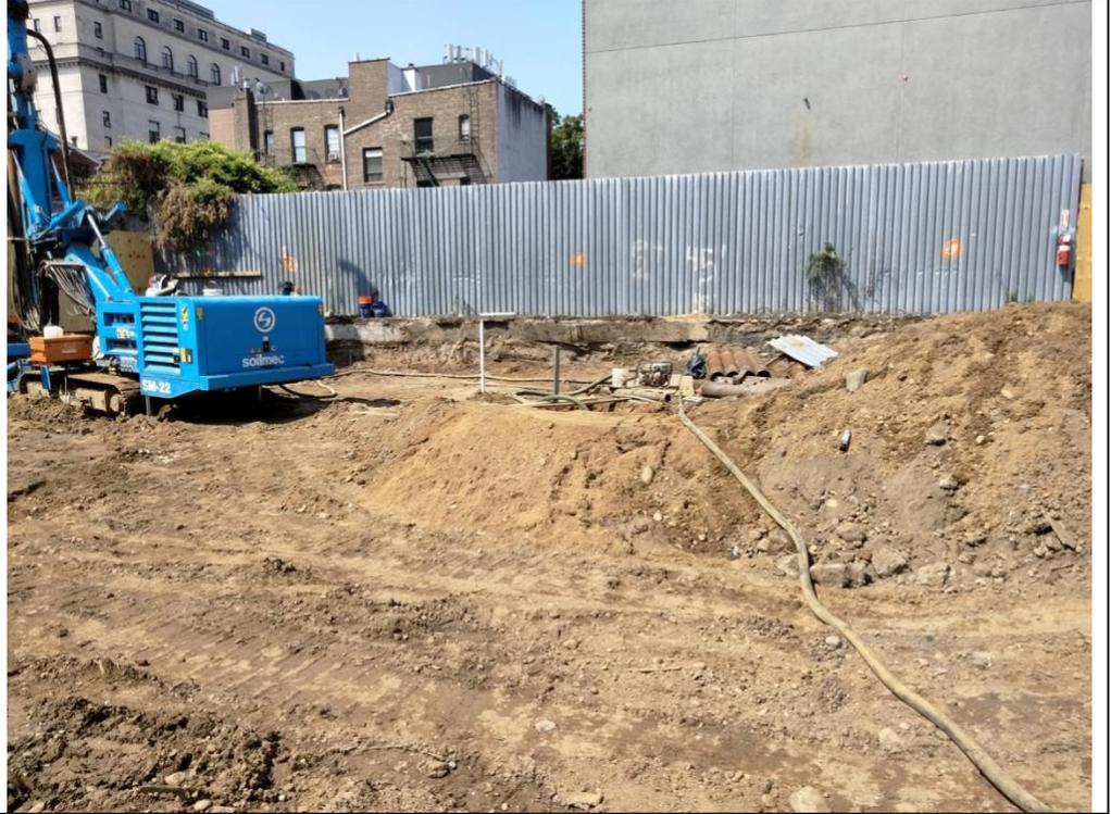
Photo 2 – Installing shoring piles along the southeastern perimeter of the site.
