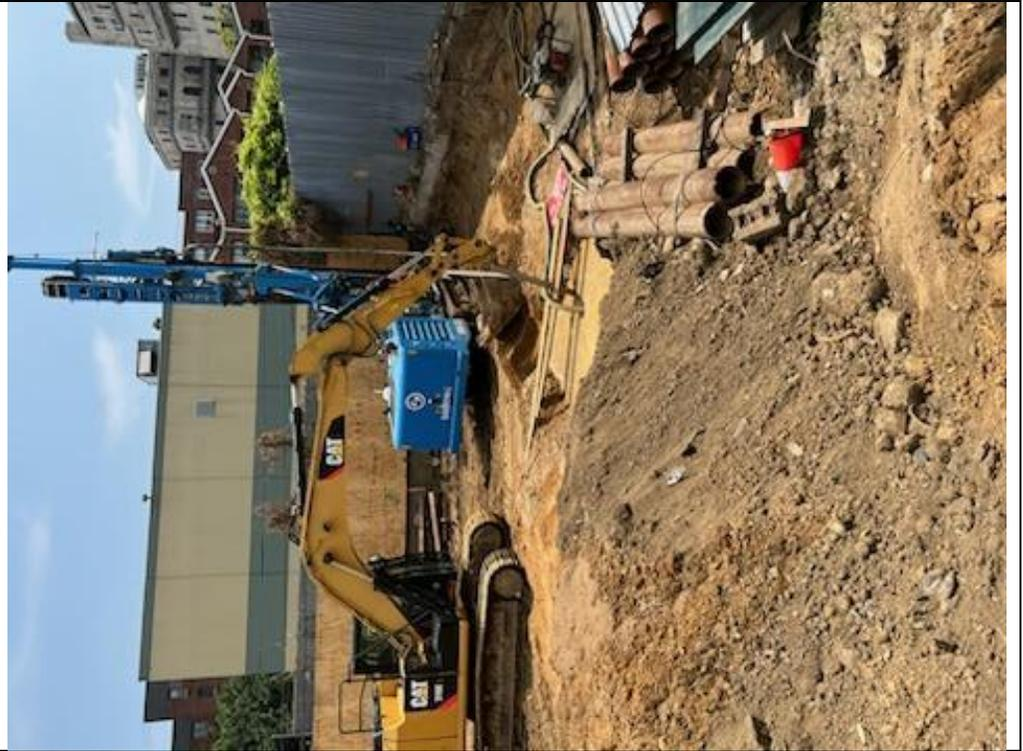
Photo 2 – Installing shoring piles along the southwestern perimeter of the site.
