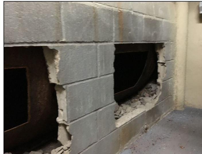
Photograph 4: View of the concrete vault for abandoned in-place AST.
