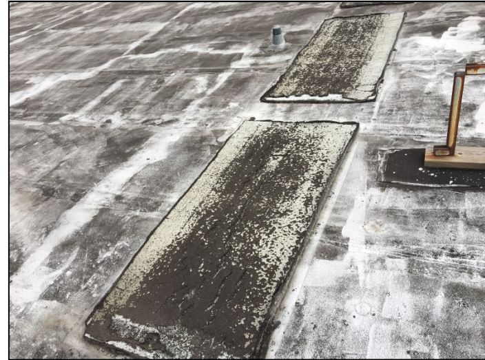
Photograph 10: Repair patches from former roof repairs.
