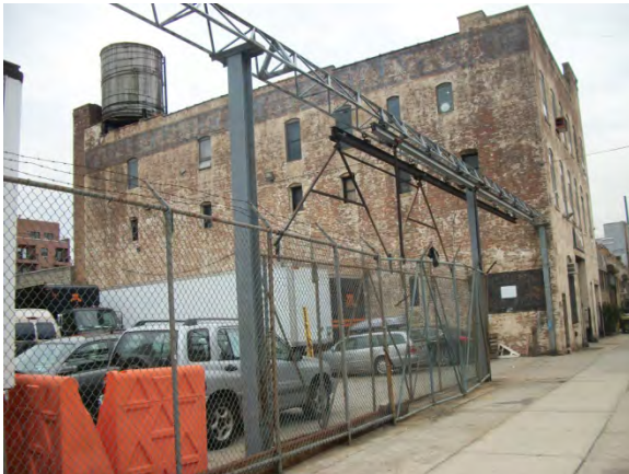
Subject Property – Northeast Elevation
