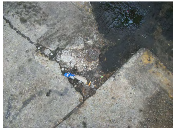
Sealed Fill Port on Southeast Side of Property
