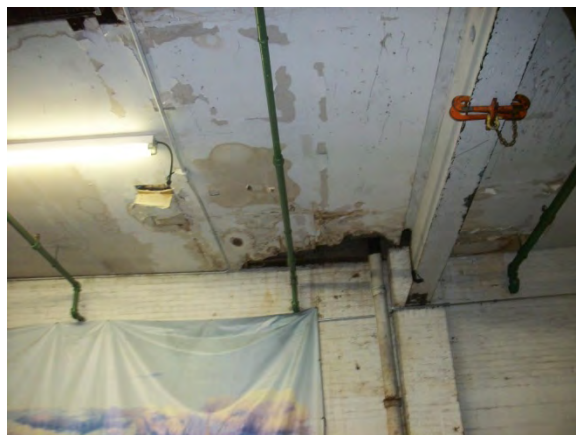
Water Staining on Basement Ceiling
