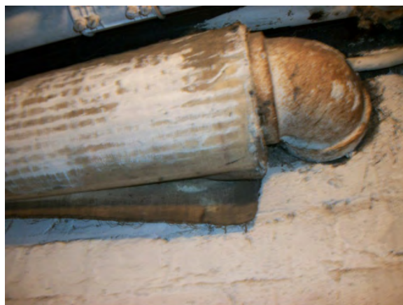
Suspect Asbestos Containing Pipe Insulation in Basement
