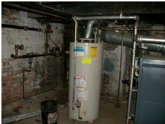
Gas Hot Water Heater Located in Main Basement
