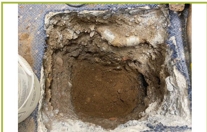
Photo #3: Interior of excavation.
