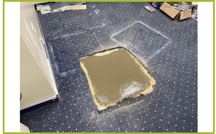
Photo #8: Concrete surface restoration.
