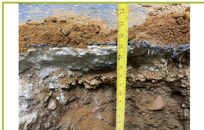
Photo #4: Excavation completed to 3.0 feet below slab.
