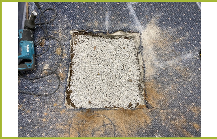
Photo #7: Excavation backfilled with quarry stone.
