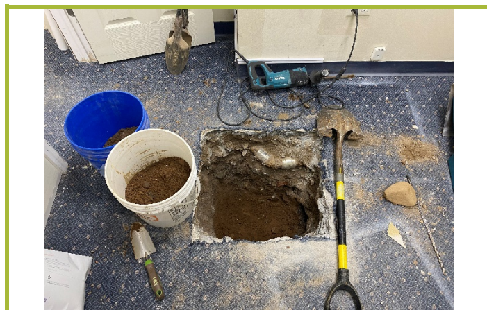
Photo #2: Excavation completed with hand equipment.
