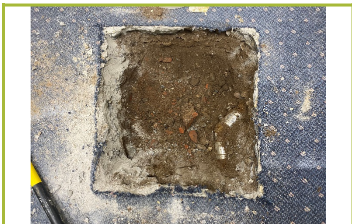
Photo #1: View of concrete slab removal.
