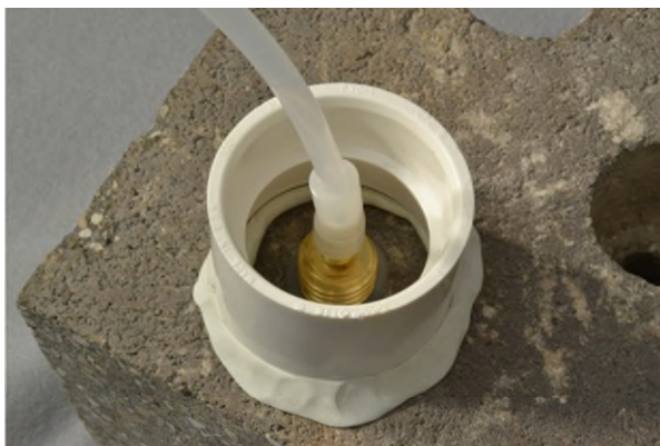
Figure 10. Water dam used for leak detection
