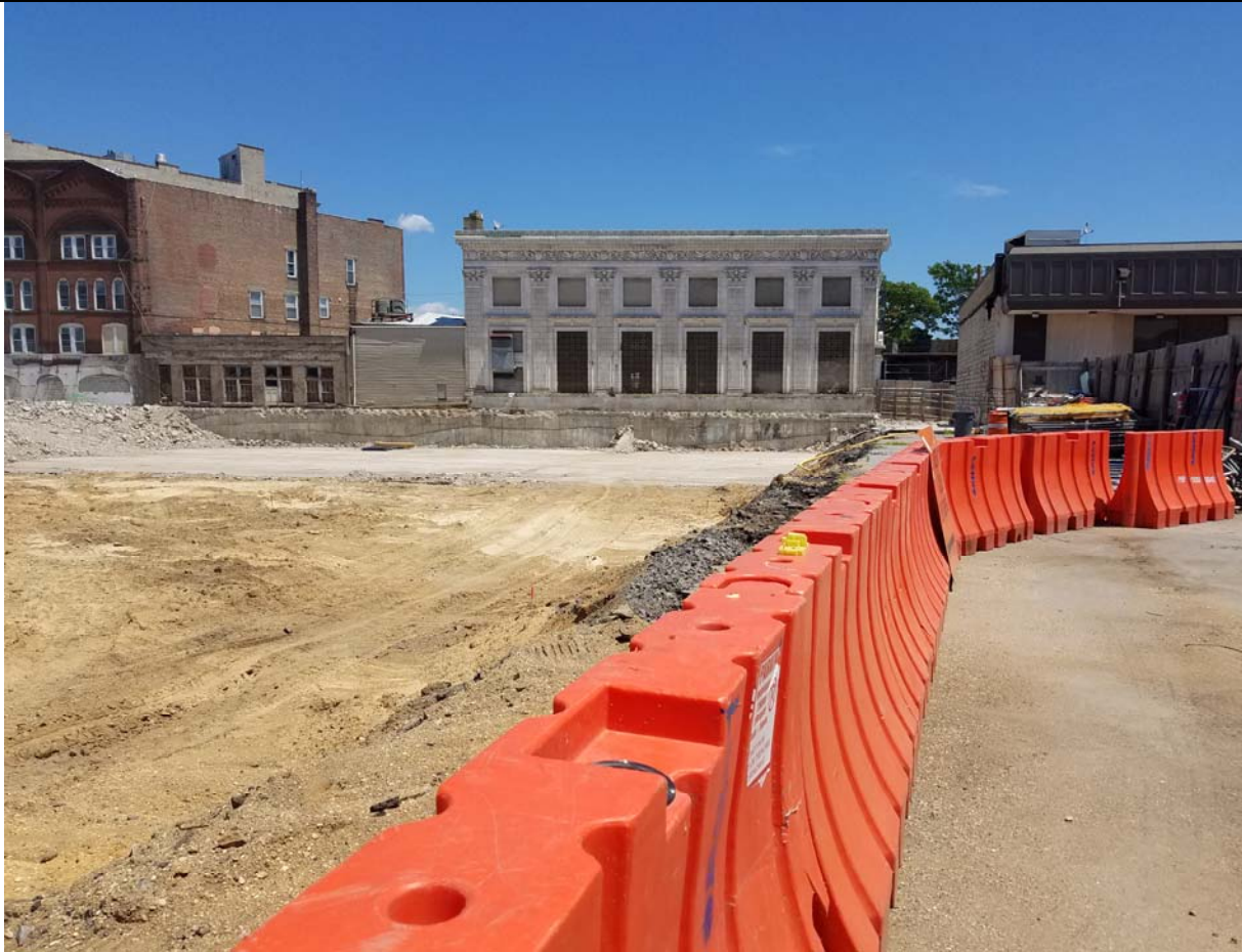
Photo 2 – View of southeastern excavation portion of the Site.
