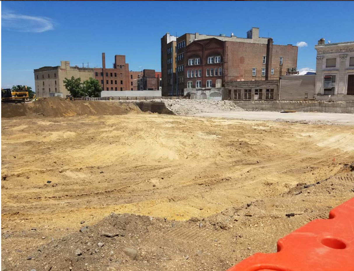
Photo 3 – View of Southeast excavation portion of the Site.
