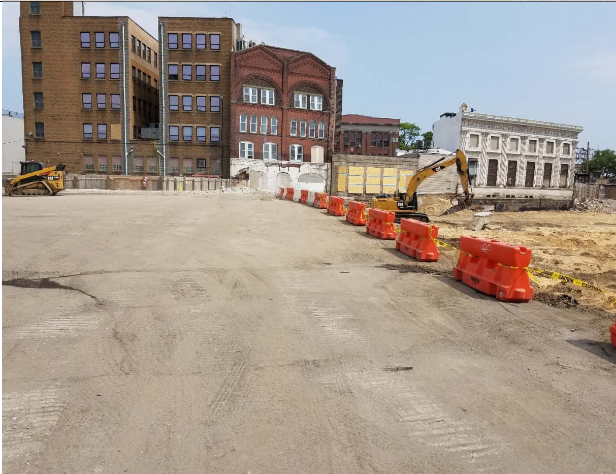
Photo 9- View of the excavation near Grids D, E, and F 4.
