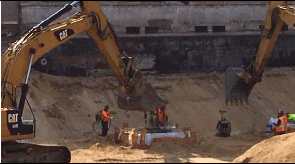
Photo 3 – View of pouring concrete in F3.
