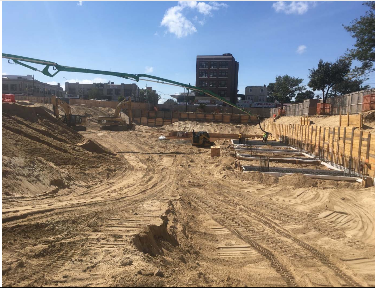
Photo 3- View of Building C footprint.
