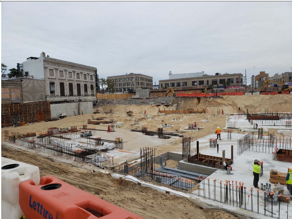
Photo 6 – View of Building B. The view is looking towards the southeast.
