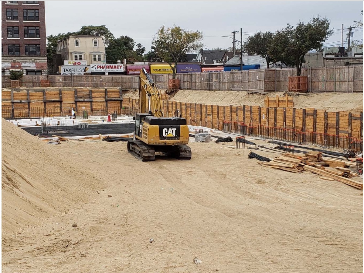
Photo 8 – View of Building C excavation. View is looking south.
