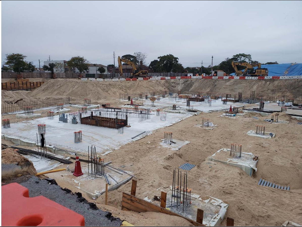
Photo 3- View of Building B excavation area. View is looking towards northwest.
