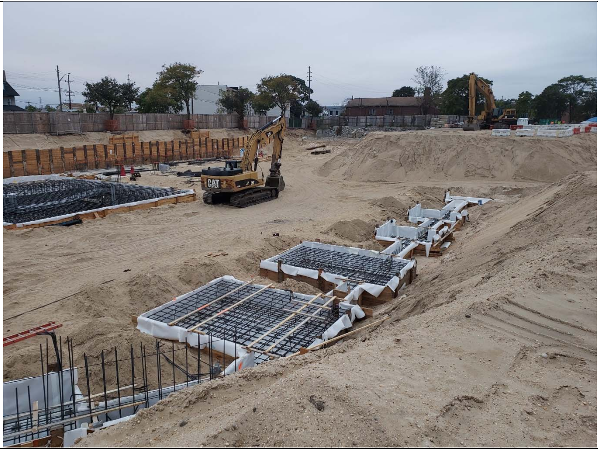
Photo 5 – View of the excavation in Building C. View is looking northwest.
