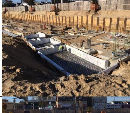
Photo 2- View of backfilling in B1 and B2.
