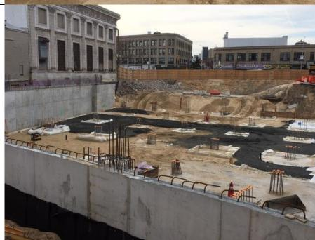
Photo 3- View of installed waterproofing membrane bituthene and hydroduct in A1 and B1.
