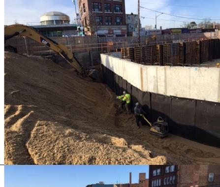
Photo 2- View of Preprufe 200 installation in E2 and E3.
