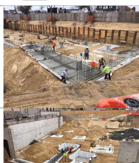
Photo 2- View of Preprufe 200 installation in E3, E4, and F3.
