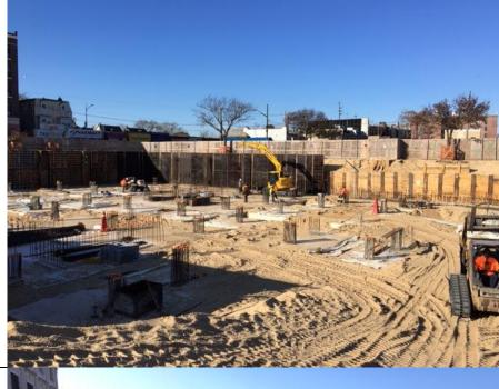
Photo 2- View of formwork, rebar, and Preprufe 200 installation in E2 and E3.
