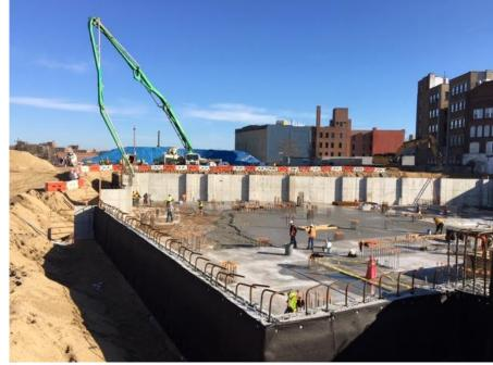
Photo 3- View of installed waterproofing membrane bituthene and hydroduct in B1 and B2.
