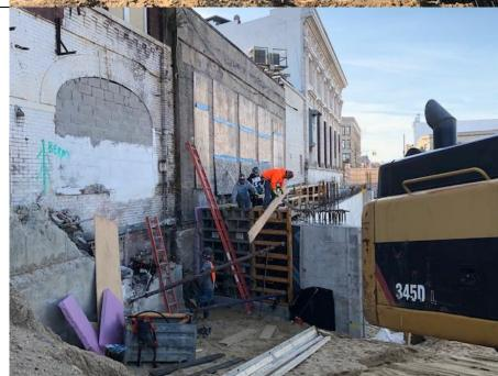
Photo 3- View of rebar installation in D2.
