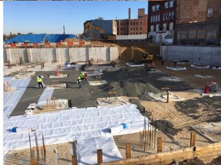
Photo 3- View of rebar installation in A3.
