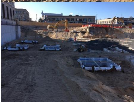
Photo 3- View of Preprufe 200 and rebar installation in E2.
