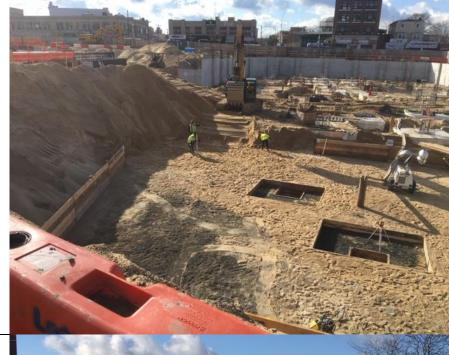
Photo 2- View of trenching and grading soil in A2 for utility installation.
