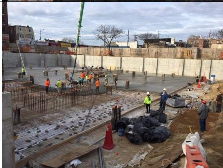
Photo 3- View of formwork and rebar installation in A4 and B4.
