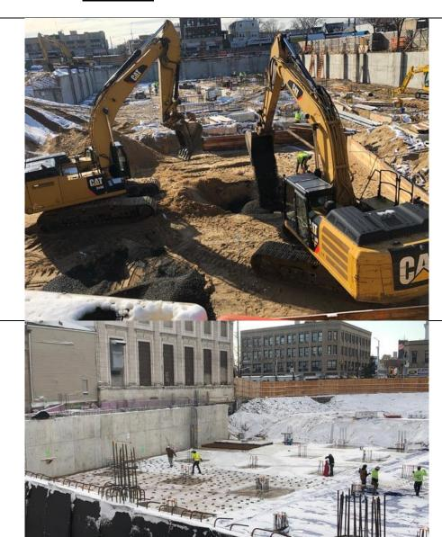
Photo 2- View of rebar installation in E2, E3, E4, F2, F4, and F4. Photo 3- View of excavating for utilities in A1 and B1.
