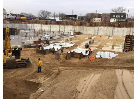
Photo 3- View of formwork and Preprufe 200 installation in B3.
