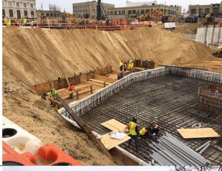
Photo 2- View of backfilling soil and installation of Bituthene and Hydroduct in A4.
